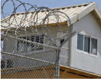
DoD IG reviewed construction of the detention facility in Parwan.
