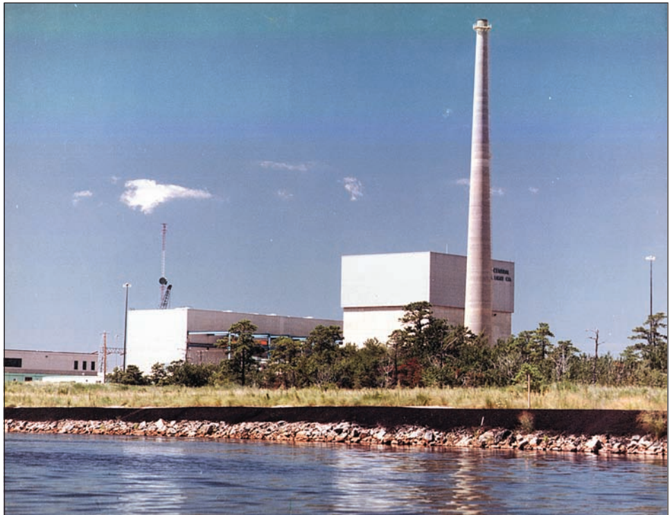
Figure 5: Oyster Creek Generating Station
