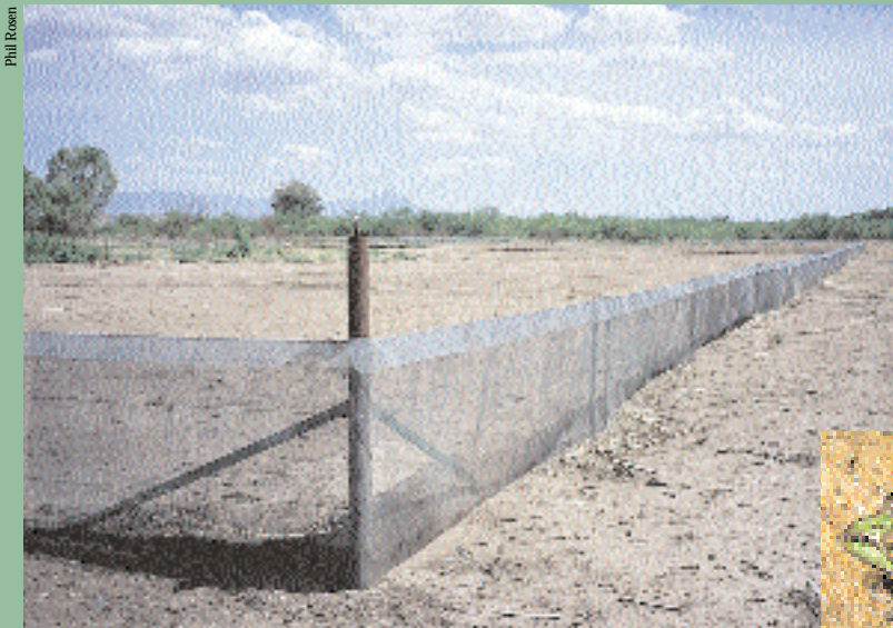
A bullfrog enclosure fence around leopard frog ponds. Bullfrogs are so adept at climbing that enclosure fences must have eaves.
