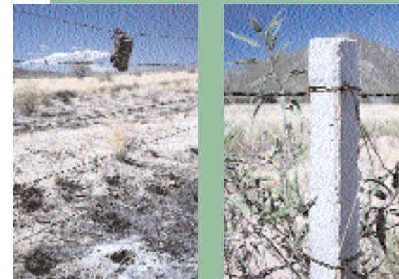
Because of frequent and severe buffelgrass fires (left), many wooden fence posts in Sonora have been replaced by concrete ones (right).
