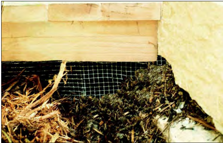
The hardware cloth extends behind the stone on the right but is hidden by mulch in this photograph.
