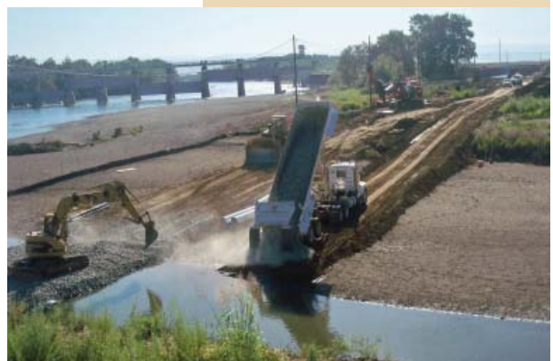
Contractors building an access road.
