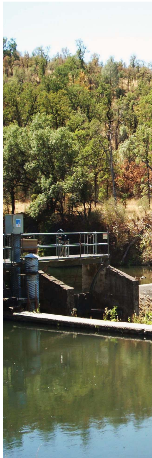
Coleman Diversion Dam is one of the affected structures.
