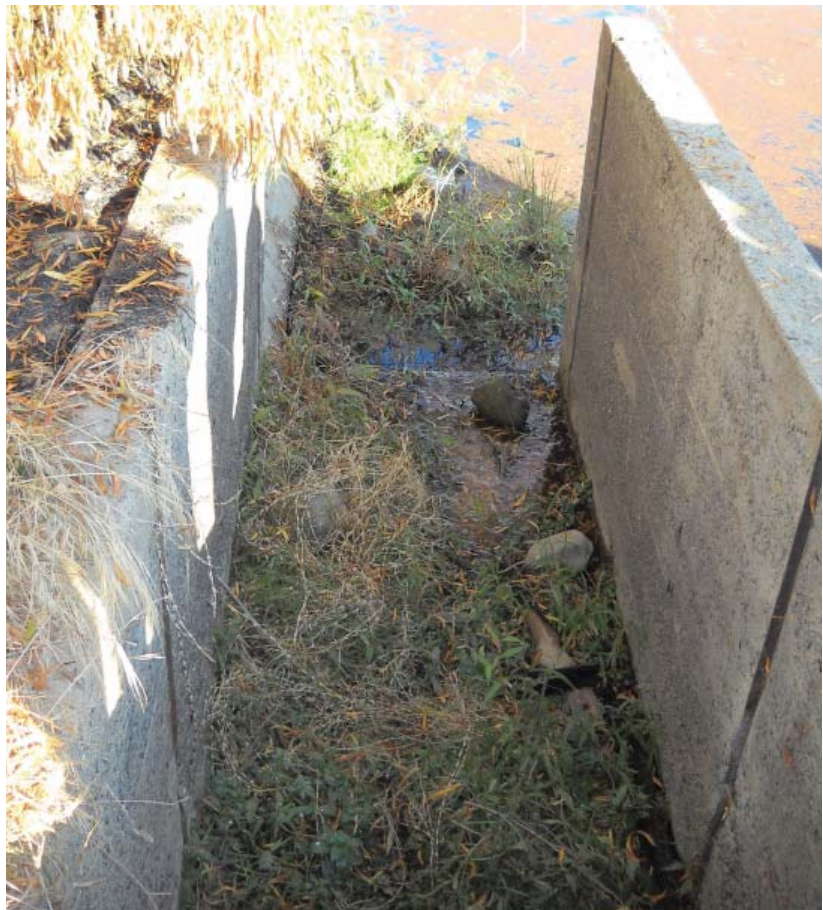
Before: The fish-ladder structure at Sack Dam on the San Joaquin River in 2009 before the return of flows.
