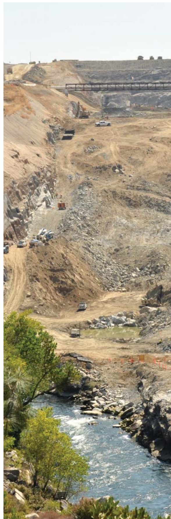
A view looking up into the auxiliary spillway.
