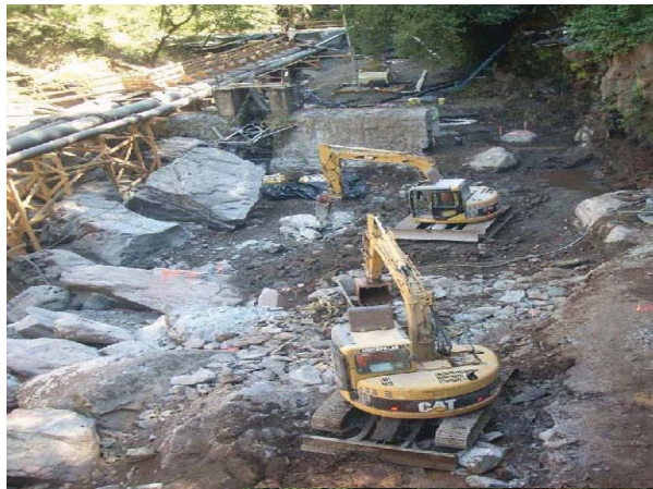
Excavating fish screen and ladder.
