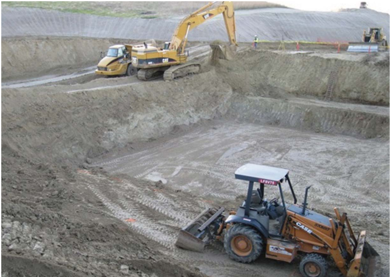
This January 2011 photograph shows excavation work for a pump plant intake for the project.
