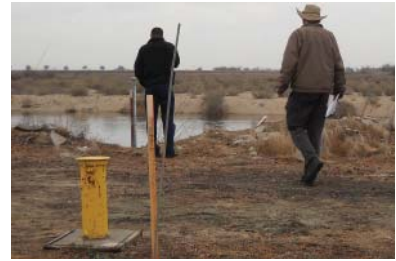
Wells have been installed to monitor the groundwater table near the river
