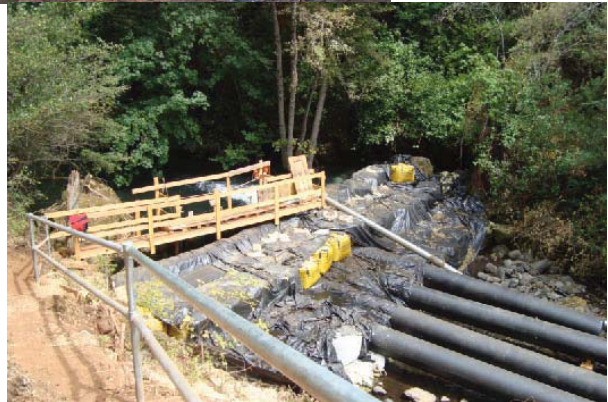
Cofferdam and bypass pipes upstream from a dam.
