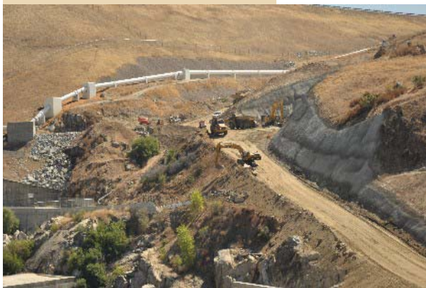
Construction improvements underway at Folsom Dam.
