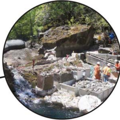
Clearing the Way Along 48 Miles for Fish
