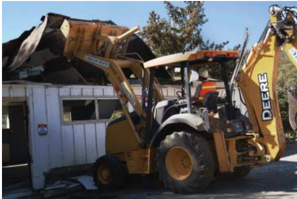
Contractor's tractor demolishes old buildings at Lake Berryessa.
