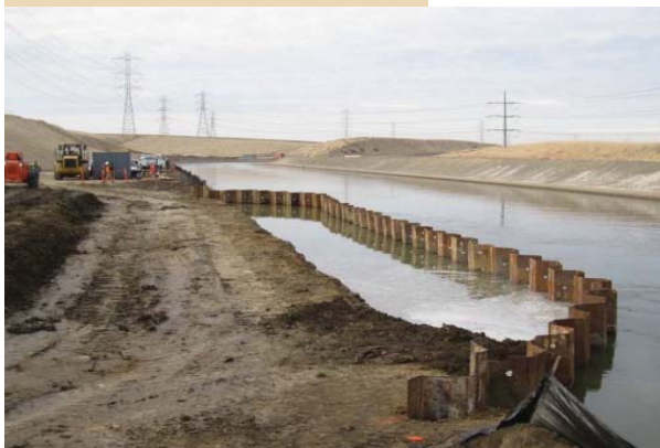
Contractors begin work on the Intertie Project along the Delta-Mendota Canal.
