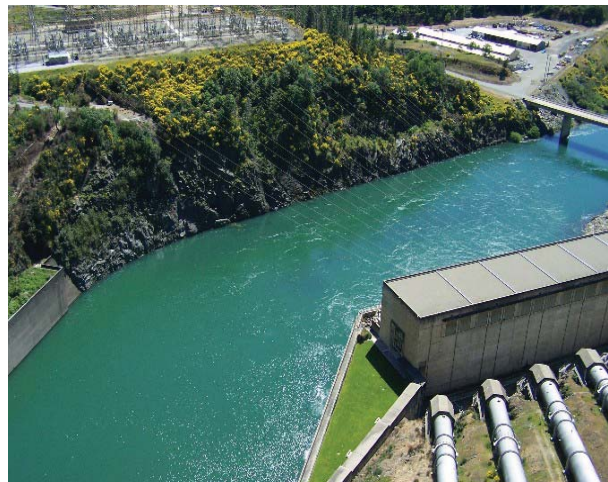
The hydroelectric power plant at Shasta Dam is one of many in the Central Valley Project.
