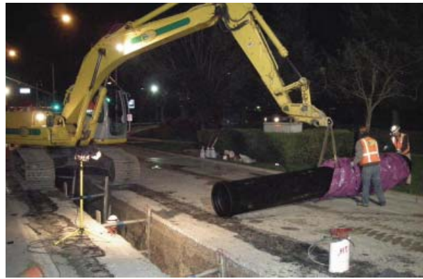
Workers use an excavator to install a recycled-water distribution pipe below a road at night to reduce effects on traffic.
