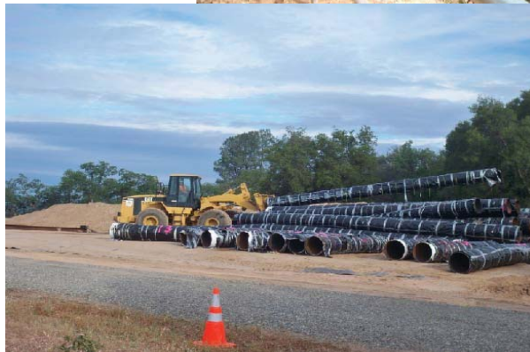
Workers stack sections of pipeline from Wildcat Diversion Dam.
