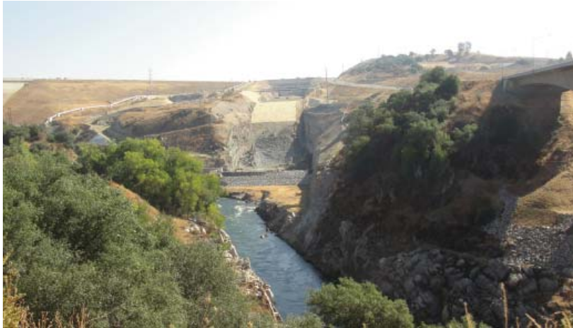
Water released into the new auxiliary spillway, shown at the top, will flow into the American River in the foreground.
