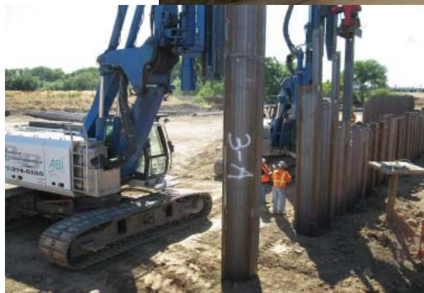
Diesel hammers drive sheet piles.
