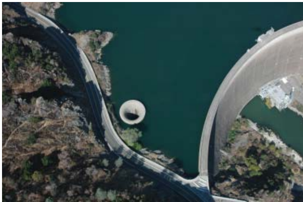
Monticello Dam in the Solano Project is noted for its "glory hole," a type of spillway with an intake shaped like an inverted bell.
