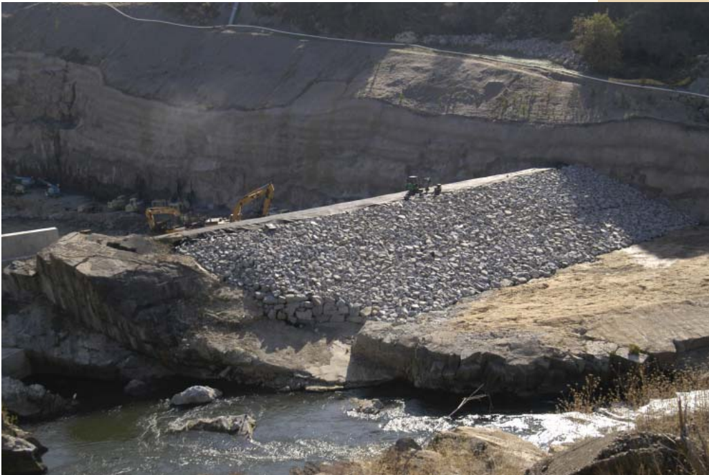
View of a temporary cofferdam nearing completion.
