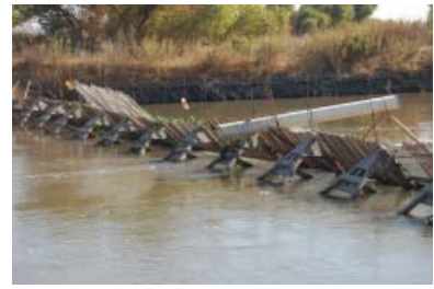
The Hills Ferry Barrier is installed seasonally to prevent anadromous fish in the San Joaquin River from following false migratory paths.
