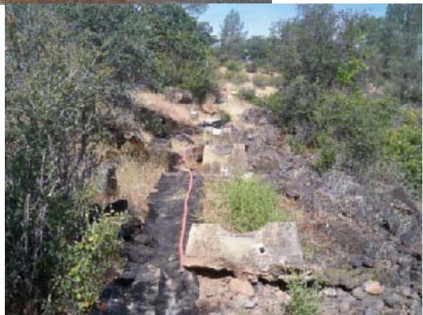
The concrete footings for the pipeline.
