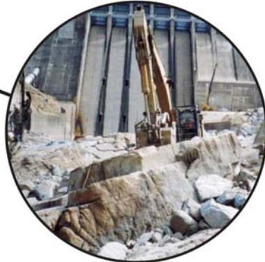
Increasing Safety at Major Reservoir
