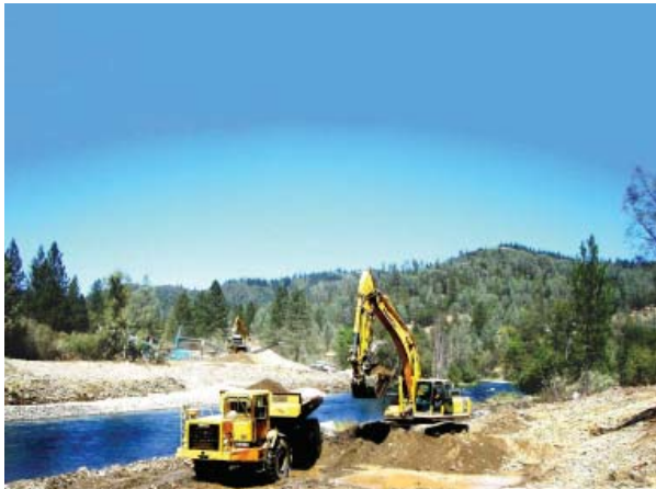
Contractors work on restoration of Trinity River.
