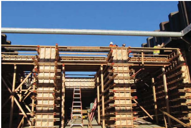
The siphon outlet structure under construction.
