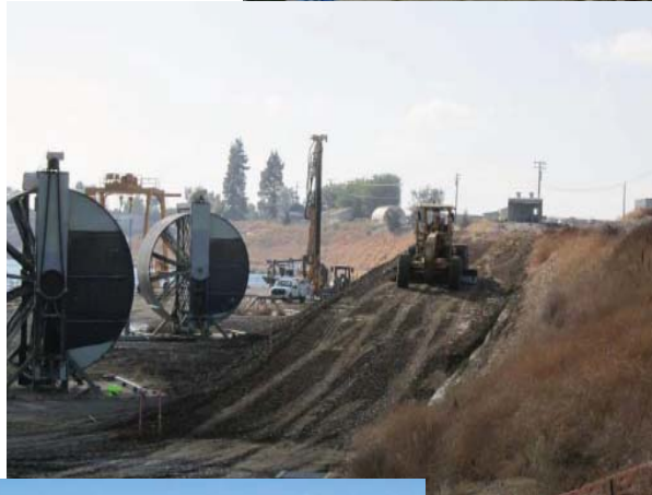
Heavy equipment excavates the canal on the east side of Red Bank Creek.
