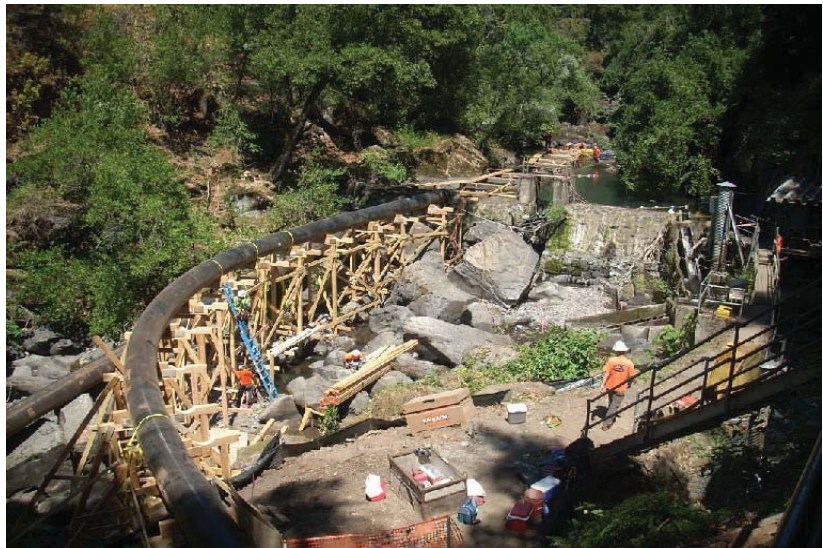
Cofferdam and bypass pipes being installed at Eagle Canyon Diversion Dam.
