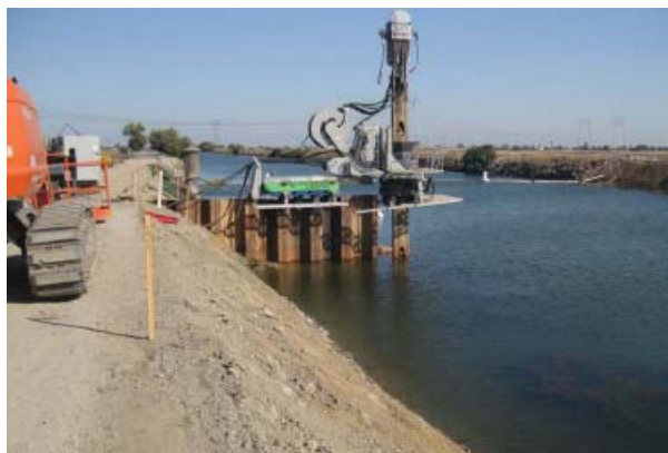
Contractors building the Contra Costa Canal Fish Screen.
