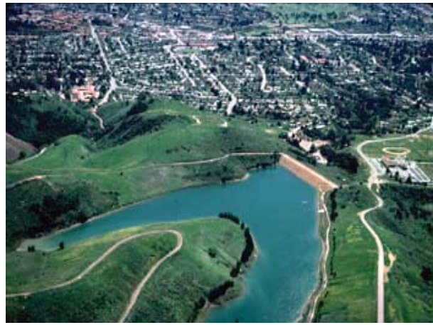
Lauro Dam is one of the facilities in the Cachuma Project.
