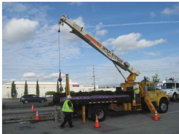
Loads of pipe to convey recycled water are hauled to sites by flat-bed trucks equipped with cranes.
