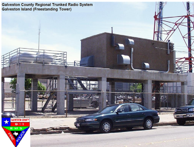
Figure 22 - Galveston Site Photo 16
