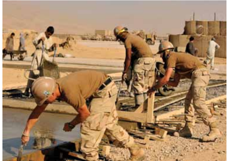
U.S. sailors and Afghan contractors building helicopter landing pads at base in Afghanistan (U.S. Navy Photo, Nov. 2010).
