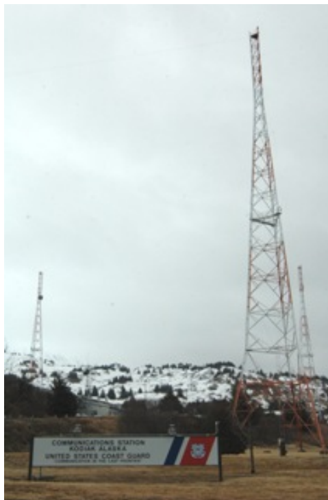
KODIAK, Alaska – Transmission antennas reach hundreds of feet into the sky over Communication Station Kodiak. The high frequency radio antennas enable the Coast Guard to communicate with vessels and Coast Guard aircraft thousands of miles out to sea. Official U.S. Coast Guard photo by PA1 Kurt Fredrickson.
