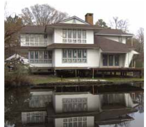
A distinctive 3,400-square-foot 1970s beach house is about to become the administrative headquarters for Back Bay National Wildlife Refuge, VA. (Greg Owens/USFWS)
