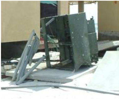
Storm surge damage.
