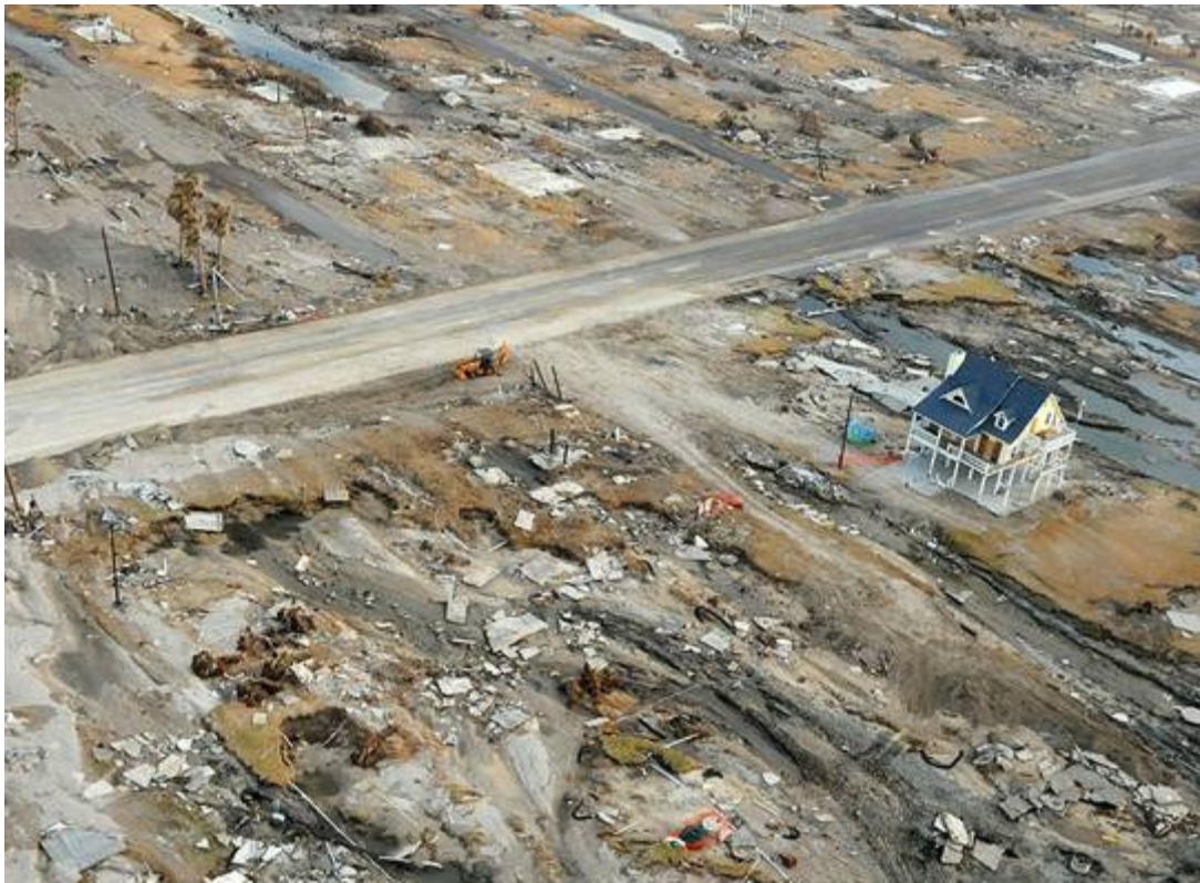
Figure 2-5. Damage in Gilchrist as a result of Hurricane Ike.
