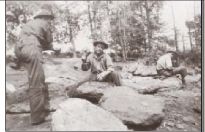
O.C. Gunn works on the children's wading pool in the Beauchamp Springs area in the 1930s. Remnants of the pool remain on the interpretive trail.
