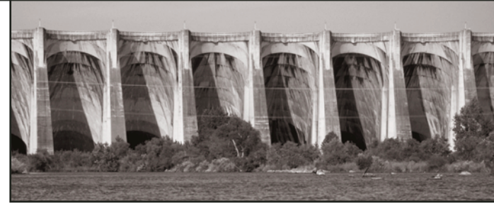
Completed in the 1937 by the LCRA after the original builder went bankrupt, Buchanan Dam is the longest multiple-arch dam in the nation. This technique is no longer used in dam building due to the amount of labor necessary. Although less labor intensive, modern dams require many more materials to build.
