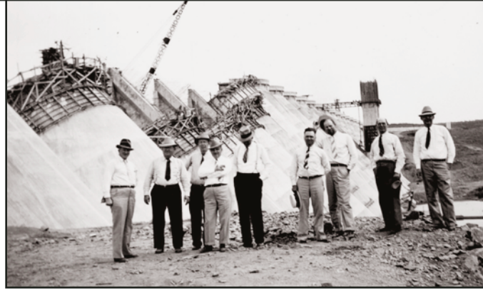
Completed in the 1937 by the LCRA after the original builder went bankrupt, Buchanan Dam is the longest multiple-arch dam in the nation. This technique is no longer used in dam building due to the amount of labor necessary. Although less labor intensive, modern dams require many more materials to build.
