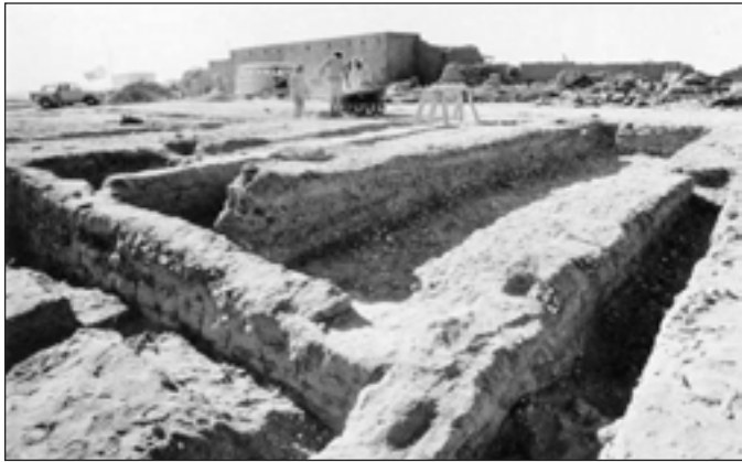
Fort Leaton in 1971 during archeological investigations and restoration work
