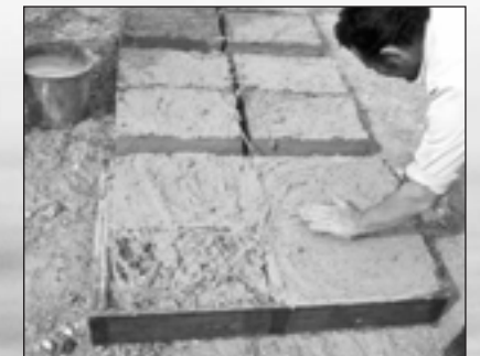
Adobe brick being made during restoration work.
