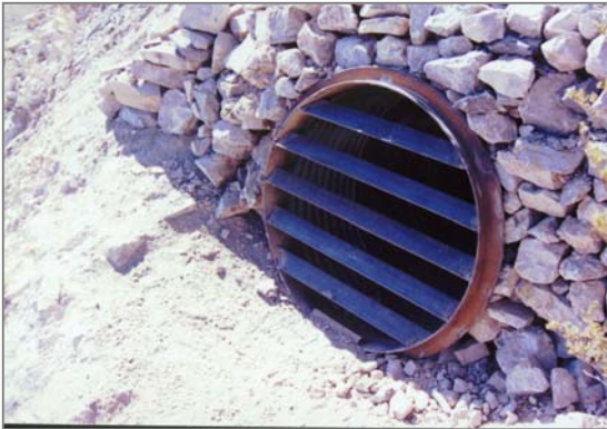
Portal with corrugated metal pipe and angle iron bat gate closure
