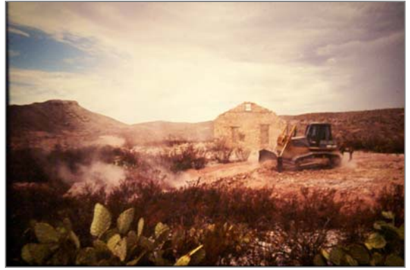
Lone Star-Mariposa mine shaft being backfilled
