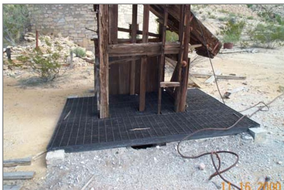
Terlingua mine shaft with steel grate closure
