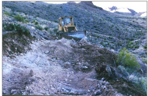
Christmas Mountain mine shaft being backfilled
