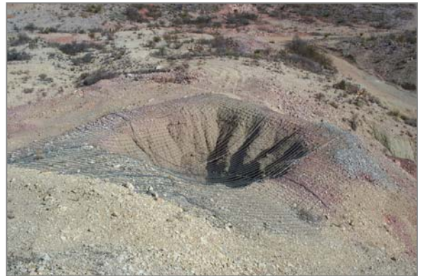
Lone Star-Mariposa mine shaft with cable-net closure
