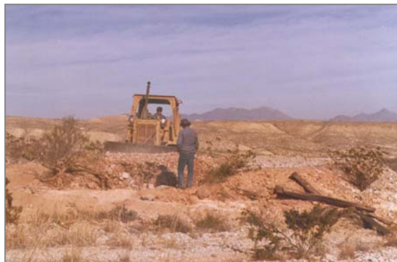
Terlingua mine backfilled shaft
