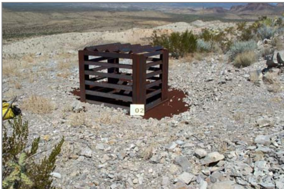
Big Bend National Park –mine shaft with angle-iron bat cupola closure
