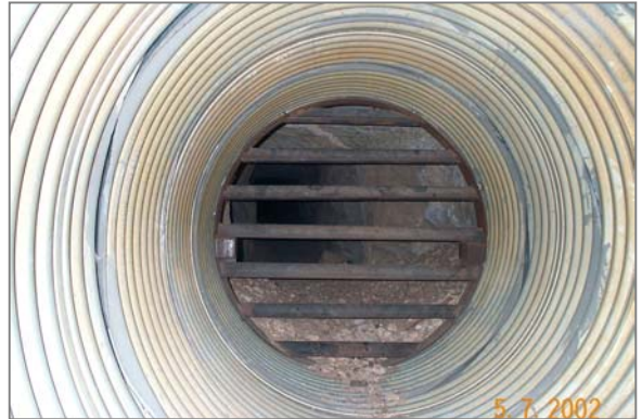
Portal with corrugated metal pipe and angle iron bat gate closure
