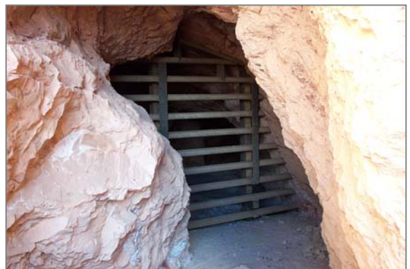
Portal with angle iron bat gate closure
