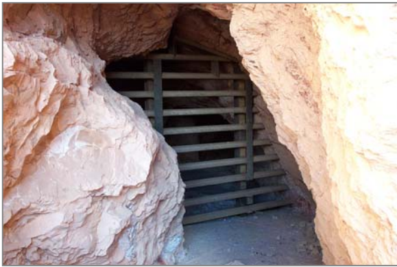
Lone Star-Mariposa adit with bat gate closure
