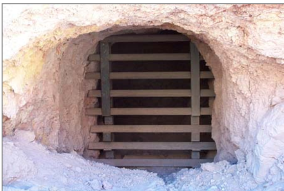
Portal with angle iron bat gate closure
