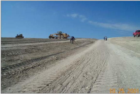
Constructing drainage channels.
