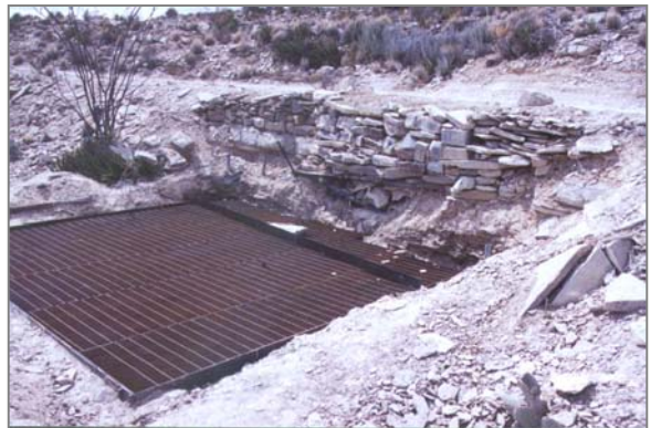
Big Bend National Park – mine shaft with steel grate closure
