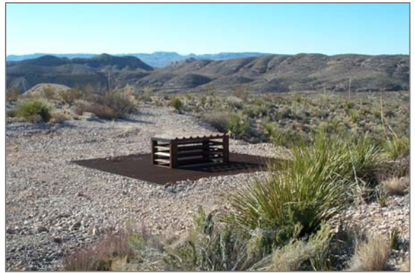
Lone Star-Mariposa mine shaft with steel grate closure
