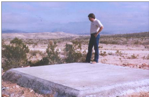
Terlingua mine shaft with concrete cap closure
