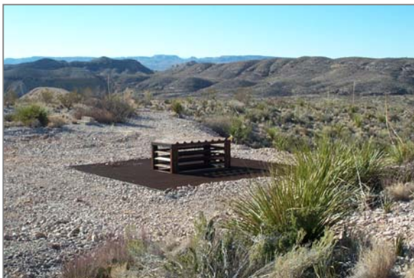
Mine shaft with angle iron bat gate cupola closure
