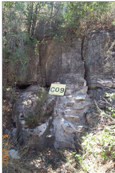
Rock and mortar closure
