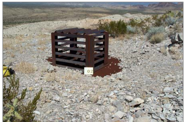
Mine shaft with angle iron bat gate cupola closure
