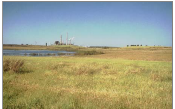
Alcoa Area 9 Post-Construction
