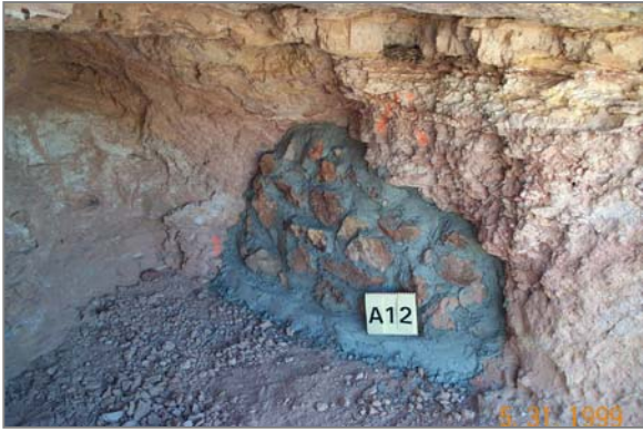
Lone Star-Mariposa adit with rock mortar wall closure
