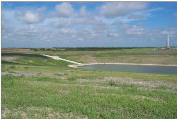
A drainage control network is needed to transport overland flow into the reclaimed pit bottom.
