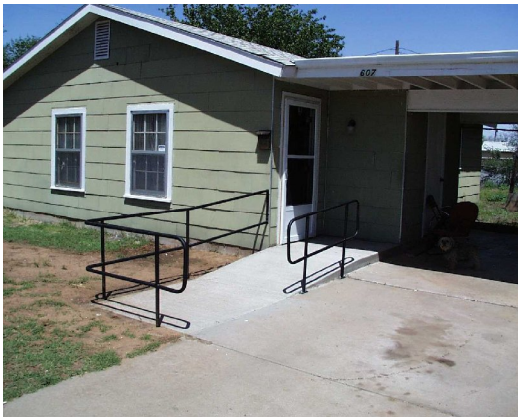
(View of exterior wheelchair ramp)
