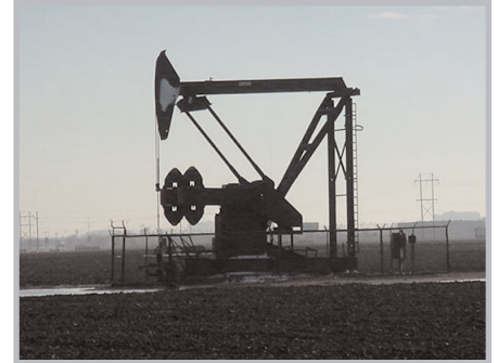
OIL PUMP LOCATED IN STUDY AREA
