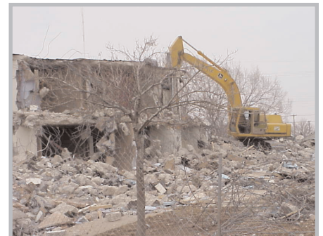
DEMOLITION OF INADEQUATE HOUSING
