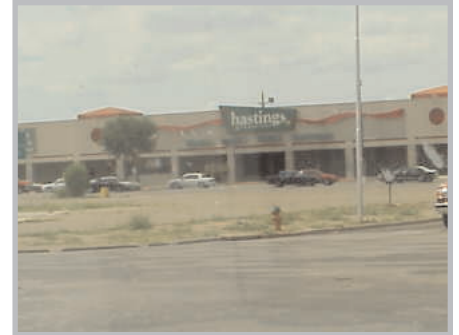
EXISTING RETAIL ON SITE 1
