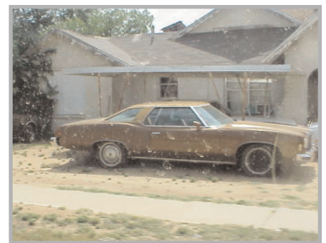
EXAMPLE OF CODE VIOLATION
