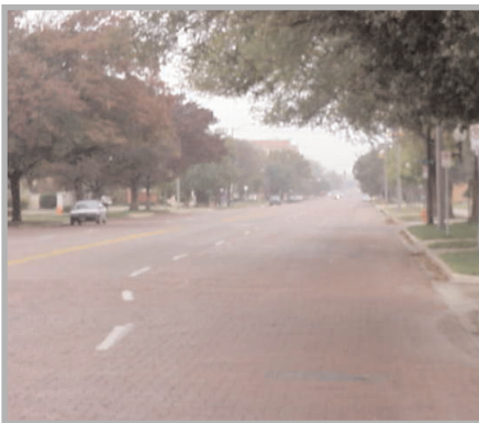
EXISTING BROADWAY CORRIDOR
