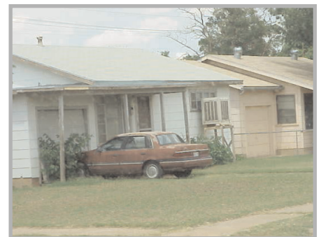
HOUSE LOCATED IN AREA DESIGNATED "NEIGHBORHOOD STABILIZATION"
