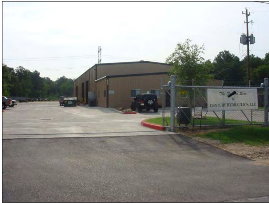
Figure 7: Century Hydraulics to the southeast of subject site.
