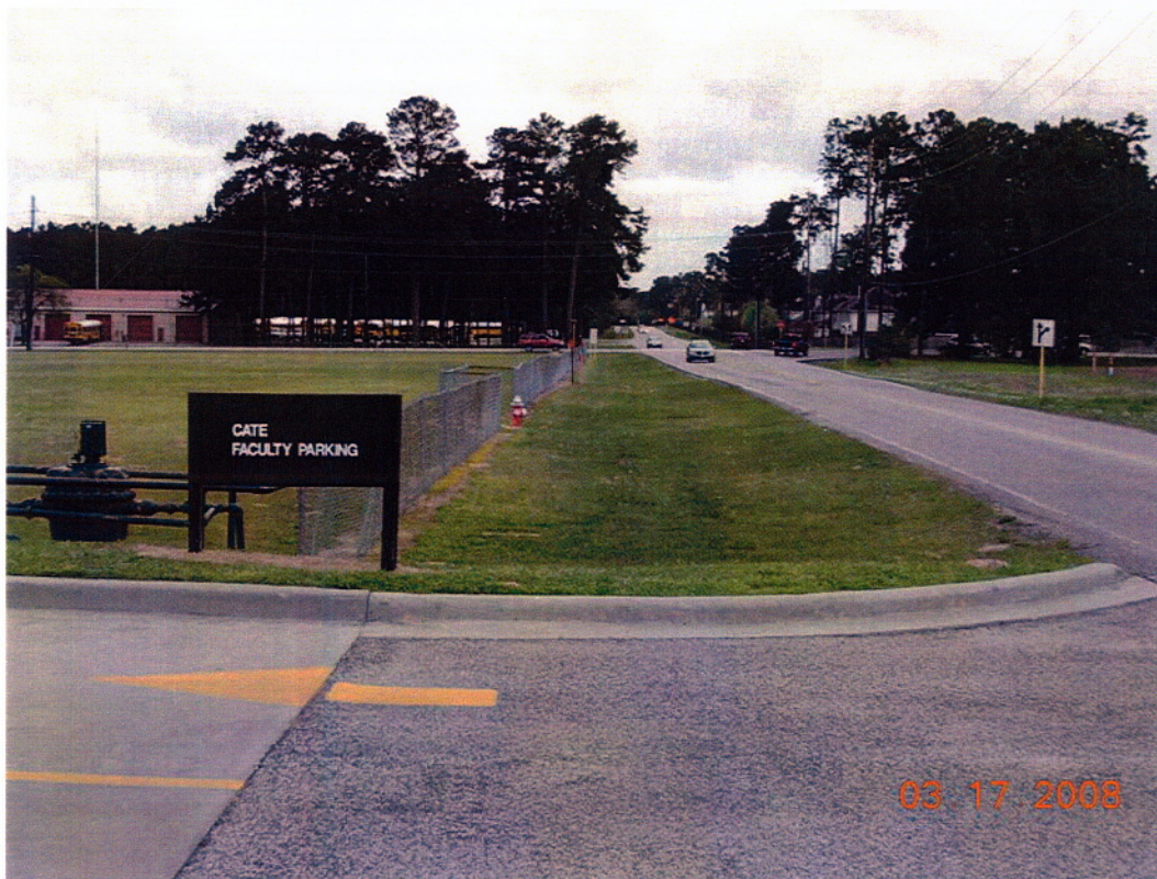
Segment 2 – Looking south along east side of Quinn Road; Baker Road in distance
