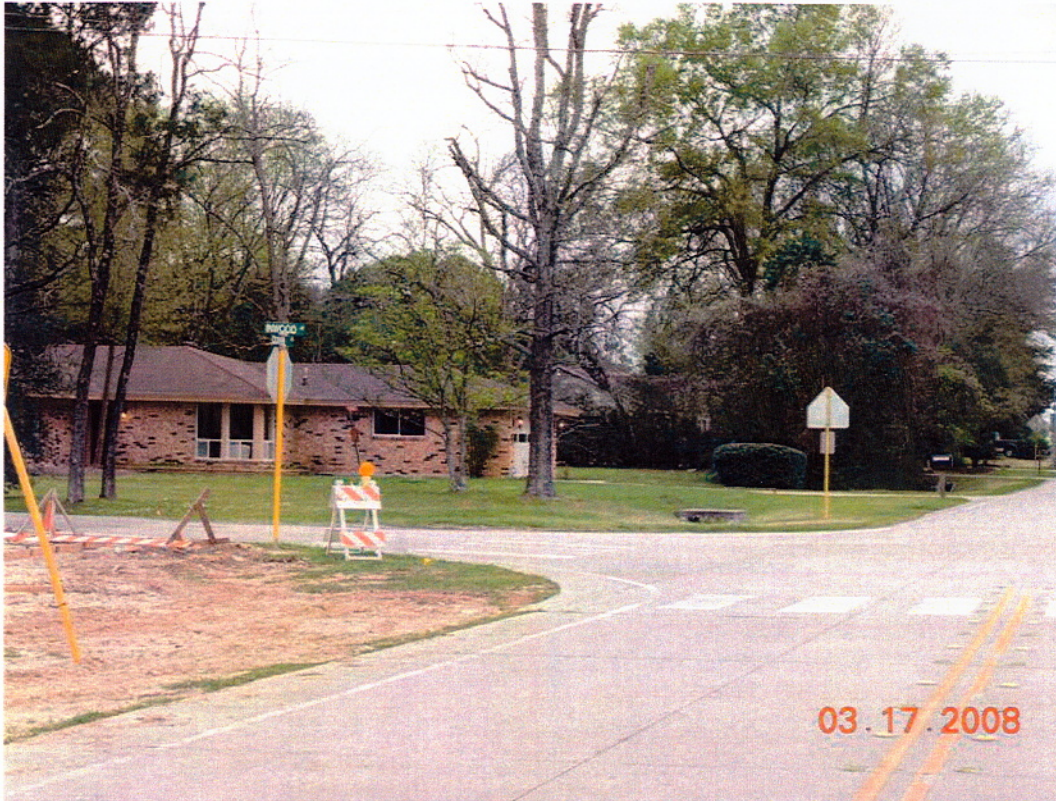
Segment 6 – Looking southeasterly at east side of Quinn Road/Inwood Street intersection
