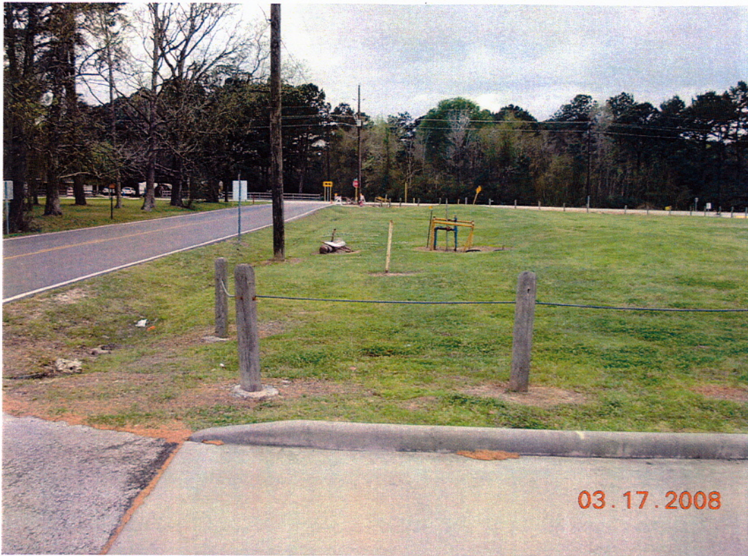
Segment 5 – Looking west along north side of Inwood Street
