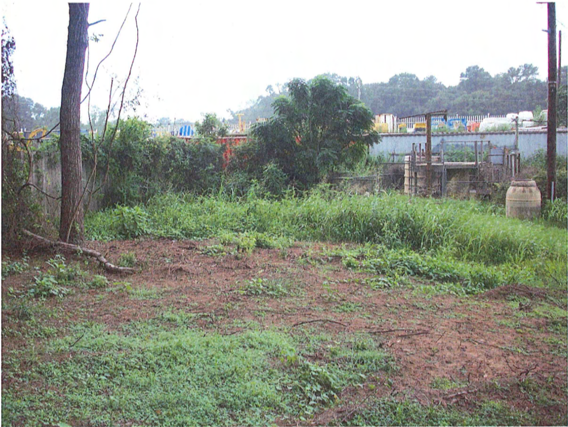
EXISTING TOMBALL HILLS LIFT STATION & WESTERN PORTION OF LOT 37 IN TOMBALL HILLS ADDITION
