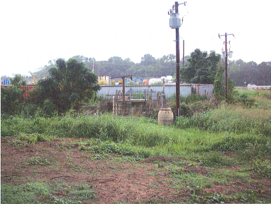
EXISTING TOMBALL HILLS LIFT STATION
