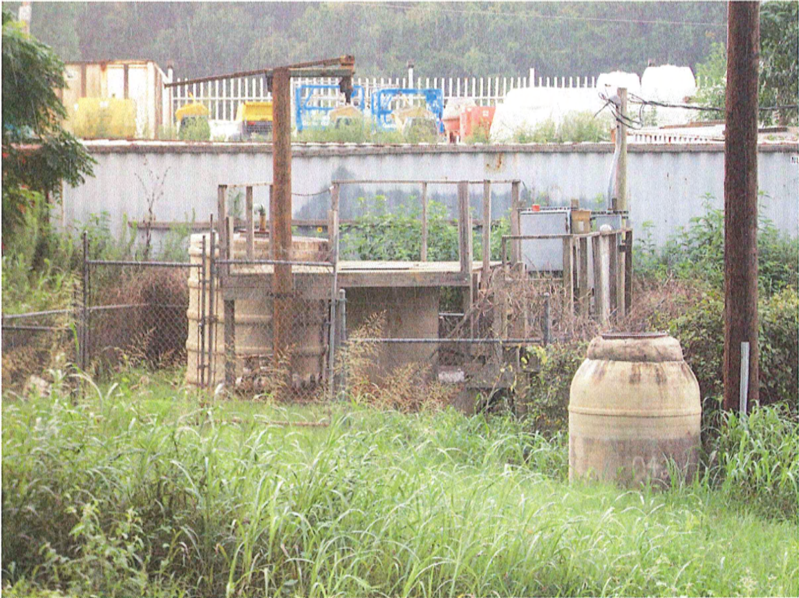
EXISTING TOMBALL HILLS LIFT STATION
