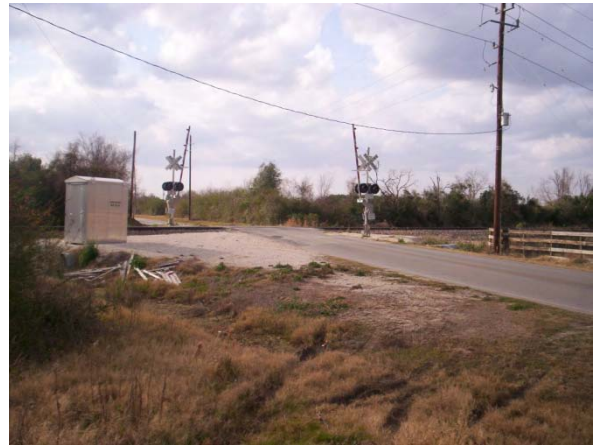
Intersection of Prop. Medical Complex Dr. (Exist Agg Rd) and BNSF RR Looking West
