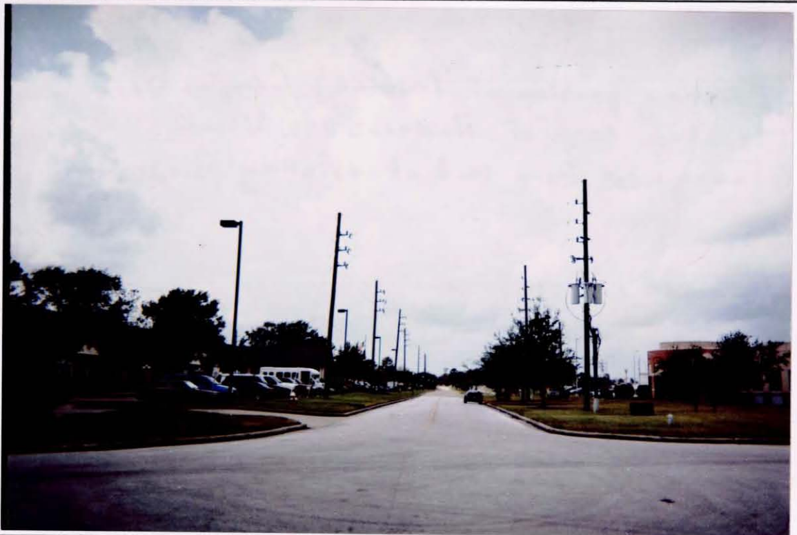
Existing portion of Medical Complex Dr. located east of Business 249. View is facing west from end of existing paved roadway.
