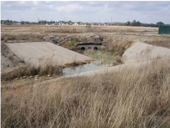
Detention Pond Outfall Looking Northwest
