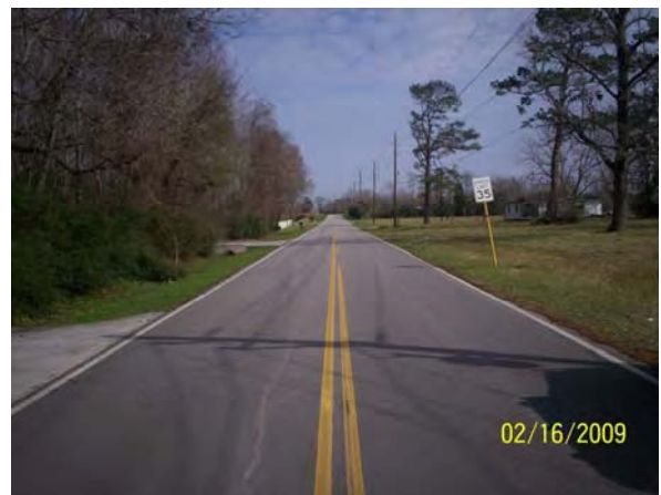
Calvert St. Near Prop. Medical Complex Dr. Looking East
