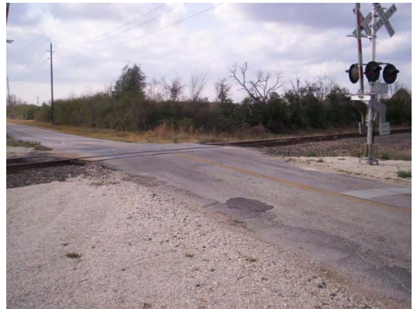
Intersection of Agg Rd. and BNSF Railroad Looking West
