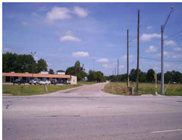
Building at Sta. 42+00 Looking West
