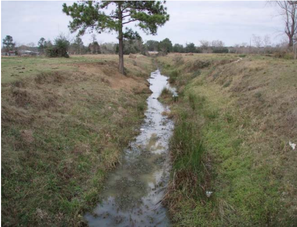
M124-00-00 approx. 1000-ft S of Triechel Looking North
