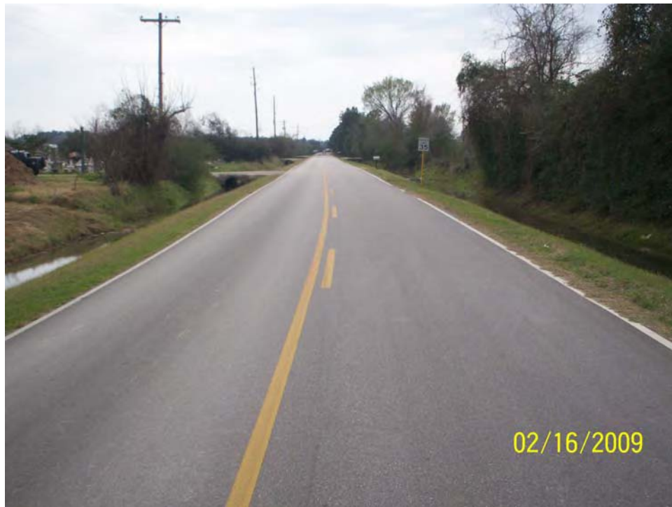
Future Medical Complex Drive @ Triechel Rd. (existing Triechel Rd.) Looking south
