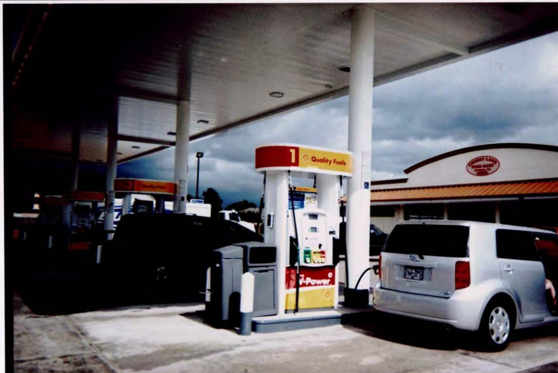
Convenience store located at northeast corner of Agg Rd. and S. Cherry.
