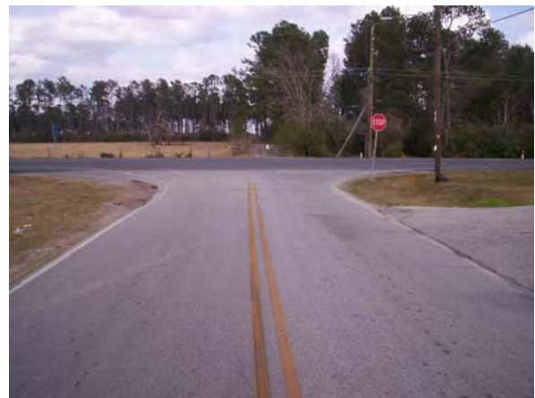
Intersection of Mahaffey Rd @ FM 2920 Looking East
