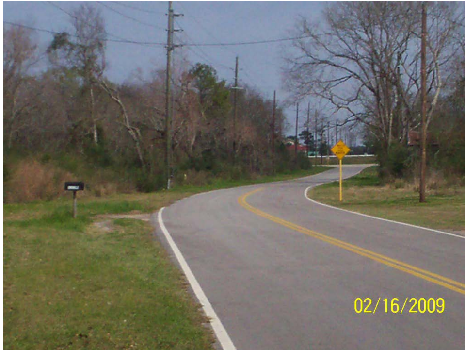
Future Medical Complex Drive access to proposed bridge west of SH 249 (existing Medical Complex Dr.) Looking east
