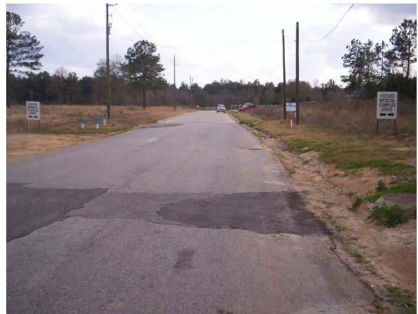
Prop. Medical Complex Dr. at School St. Looking South
