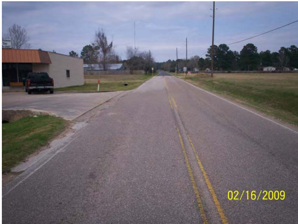
Future Medical Complex Drive (existing Park St.) @ 2920 Looking north
