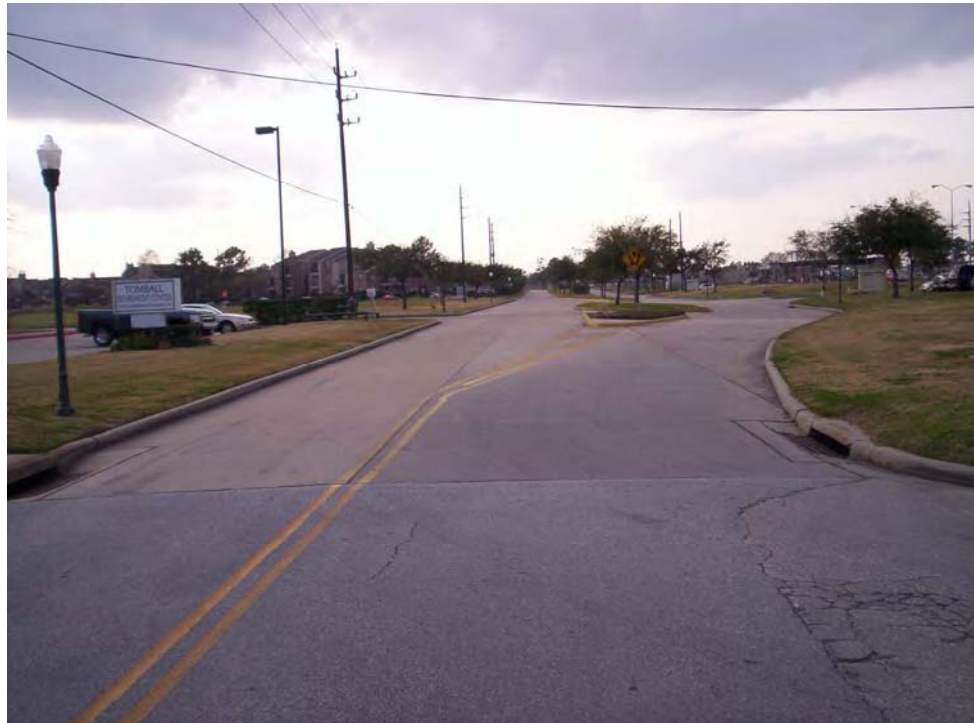
Future Medical Complex Dr. tie-in to existing Medical Complex Dr. west of Holderrieth S. Blvd. Looking west
