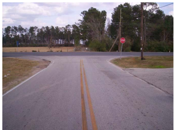
Intersection of Mahaffey Rd. and FM 2920 Looking East
