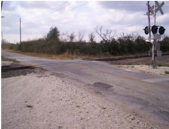
Intersection of Prop. Medical Complex Dr. (Exist Agg Rd) and BNSF RR Looking West
