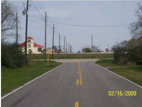
Prop. Medical Complex Dr. West Access to Prop. Bridge West of SH 249 Looking East
