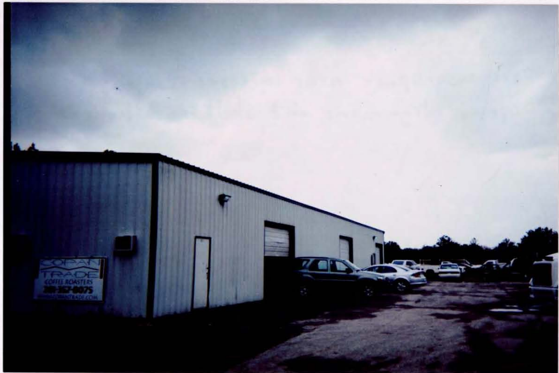
Warehouse space near intersection of proposed alignment and Huffsmith-Kohrville.
