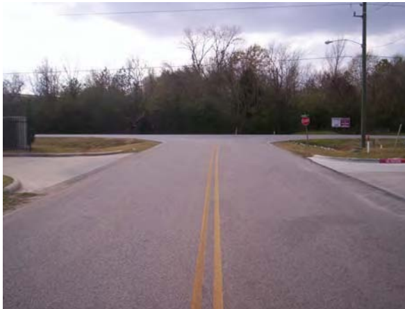
Intersection of Prop. Medical Complex Dr. (Exist Agg Rd.) and S. Cherry St. Looking West
