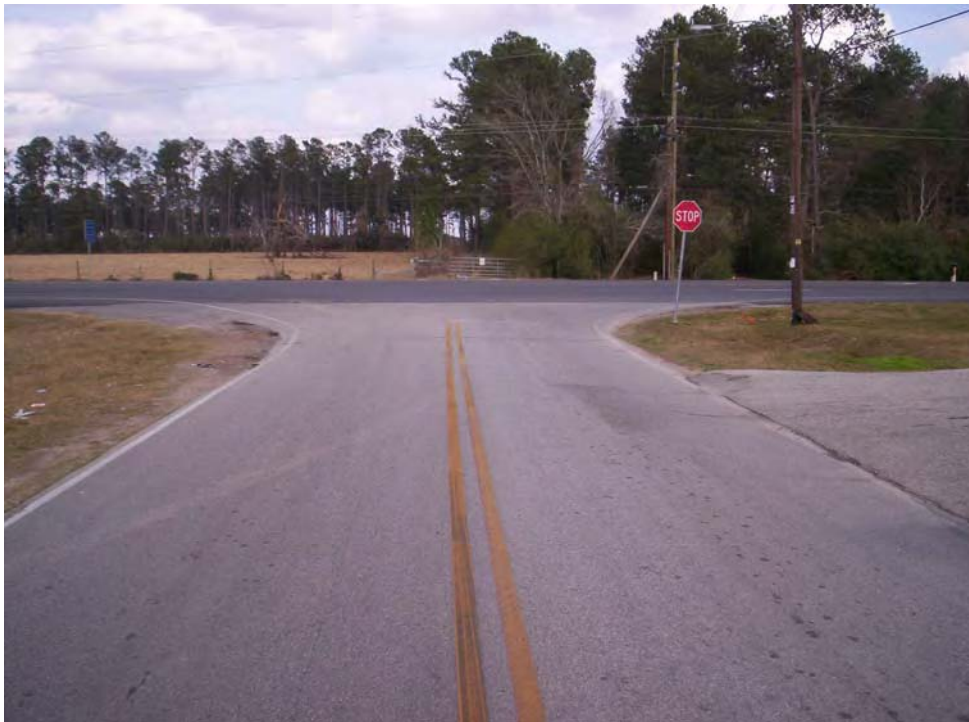
Future Medical Complex Drive (existing Mahaffey Rd.) @ FM 2920 Looking east
