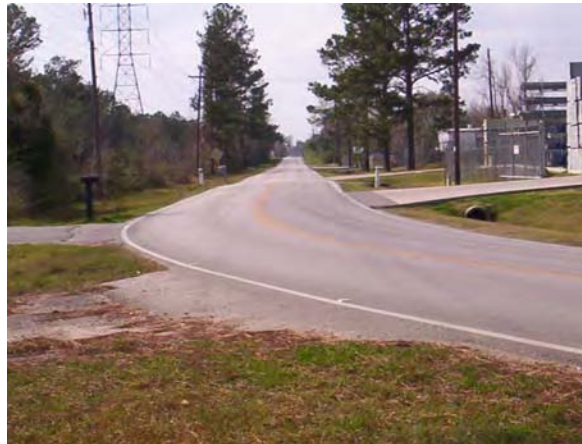
Existing Mahaffey Rd. Looking West
