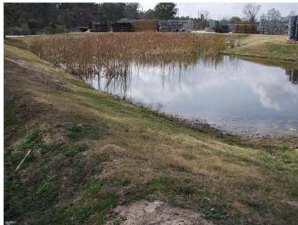
Detention Pond on Mahaffey Rd. Looking Southwest
