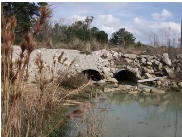
M116-00-00 Upstream (East Side) Looking East
