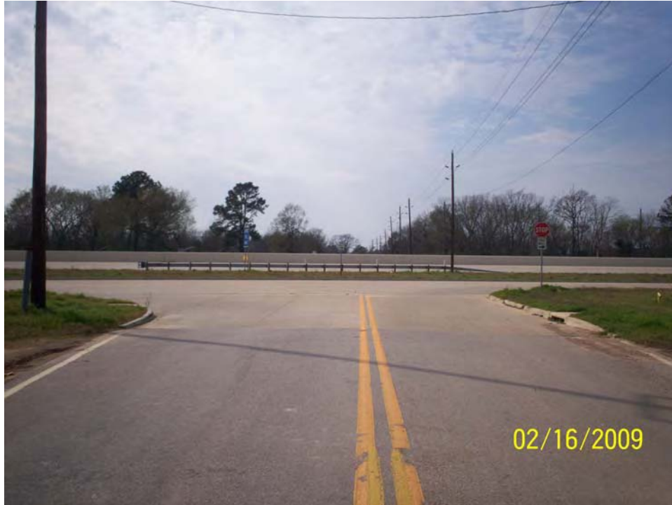
Future Medical Complex Drive proposed bridge east of SH 249 Frontage Rd. (existing Medical Complex Dr.) Looking west
