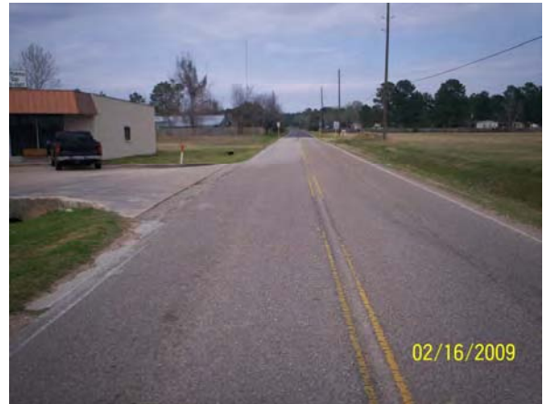
Intersection of Park St. and FM 2920 Looking North
