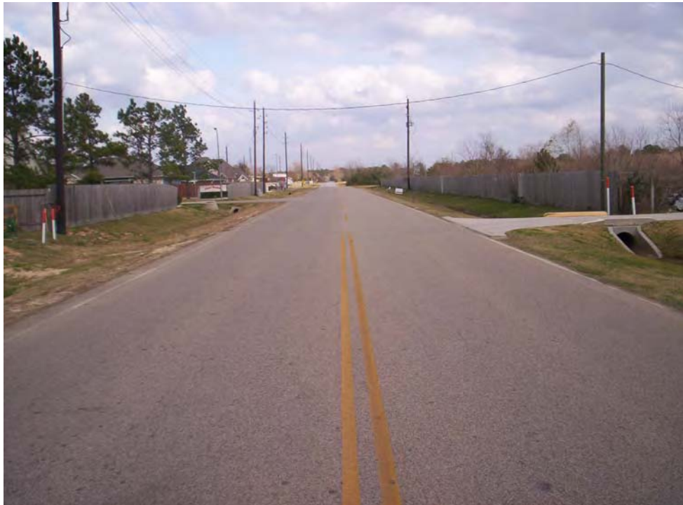
Future Medical Complex Drive (existing Agg Rd.) @ S. Cherry Looking east
