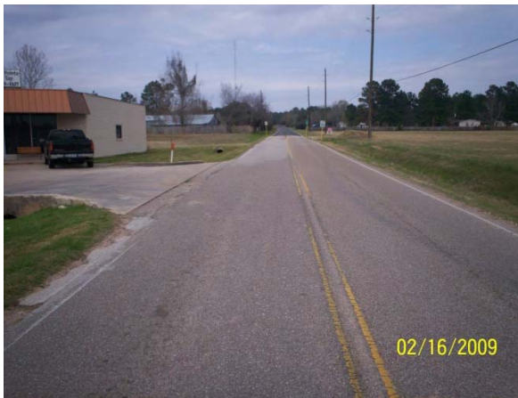
Intersection of Park St. and FM 2920 Looking North
