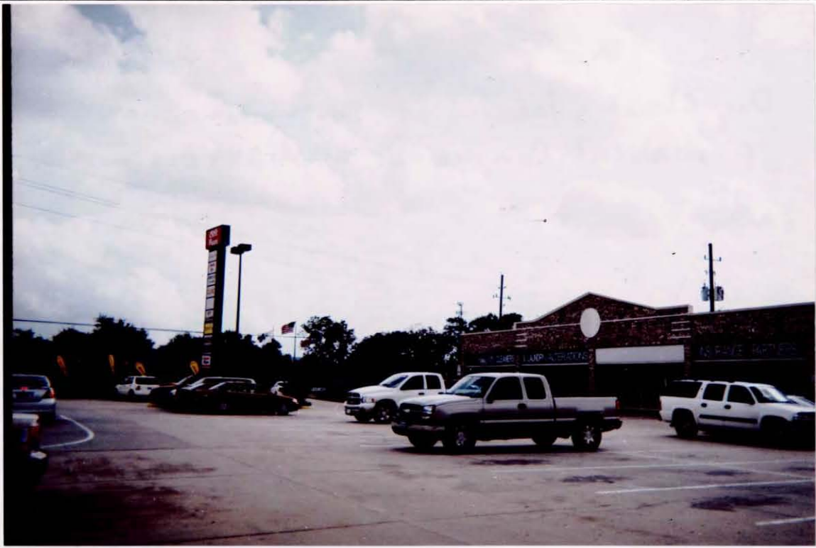
Dry Cleaners located at southwest corner of Medical Complex Dr. and 249 Business.
