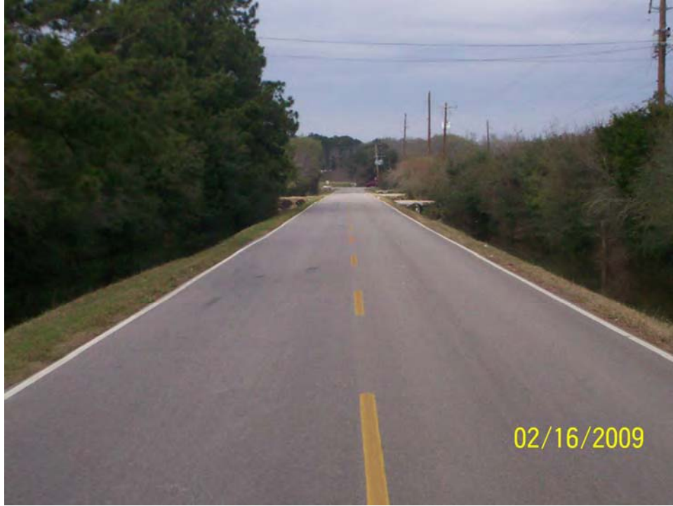
Future Medical Complex Drive @ Triechel Rd. (existing Triechel Rd.) Looking north
