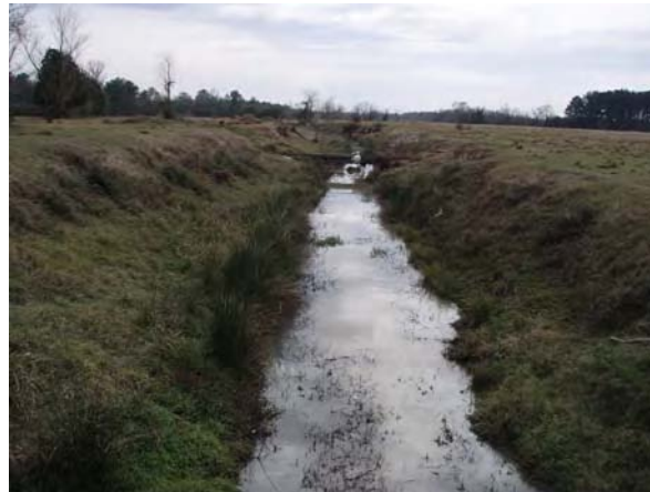
M124-00-00 South of Triechel Rd Looking South
