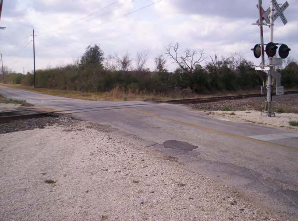
Future Medical Complex Drive (existing Agg Rd.) @ BNSF RR Looking northwest
