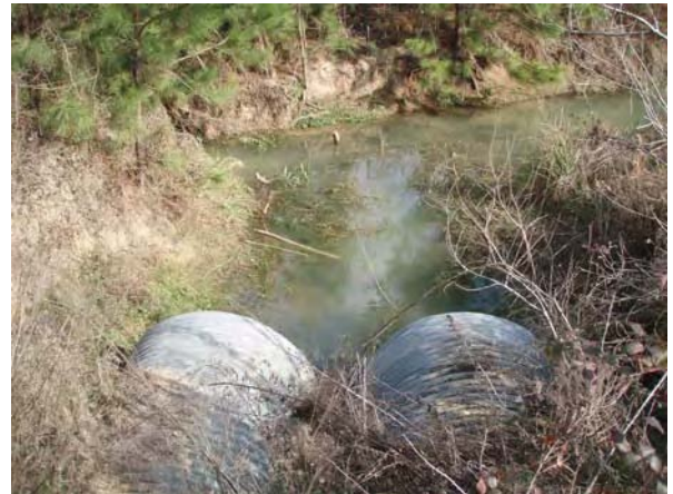
M116-00-00 Upstream (West Side) Looking East
