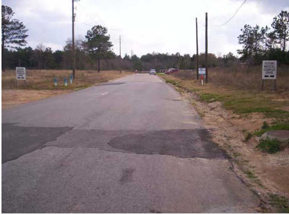
Future Medical Complex Drive @ School St. (existing School St.) Looking south
