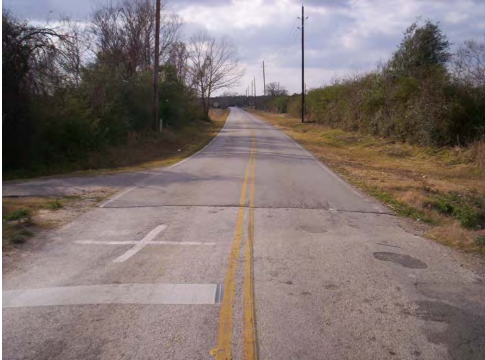
Future Medical Complex Drive (existing Agg Rd.) west of BNSF tracks Looking west
