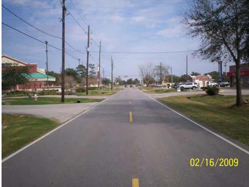
Future Medical Complex Drive access to proposed bridge east of SH 249 (existing Medical Complex Dr.) Looking east
