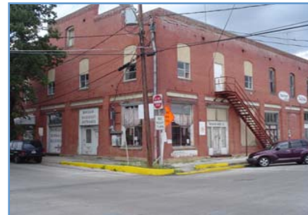
Before Burial of Electrical Conversion and Sidewalk Improvements
