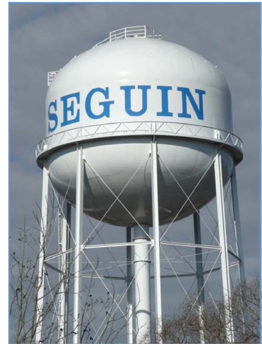
Ireland Street Water Storage Tank
