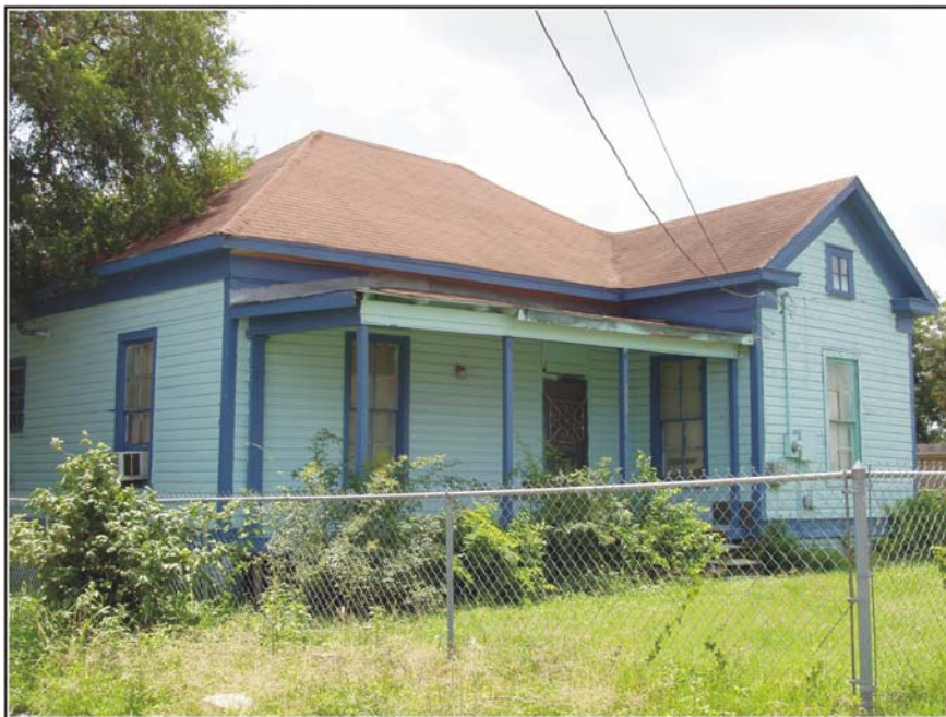
Figure 3-7. Photograph of 203 South Guadalupe.
