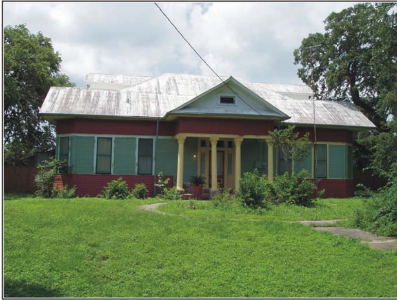
Figure 3-18. Photograph of the Goodrich-Adams House taken June 29, 2007.
