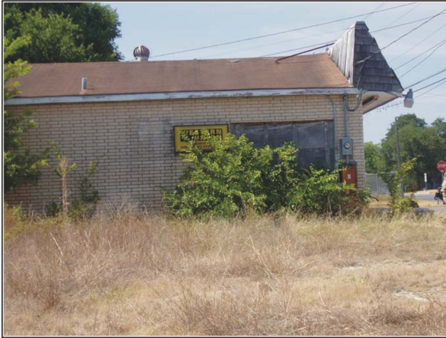
Figure 5-5. Southeast corner of Guadalupe and Court Streets (abandoned building).
