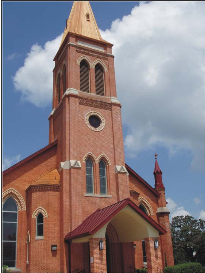
Figure 3-10. Photograph of St. James Catholic Church.
