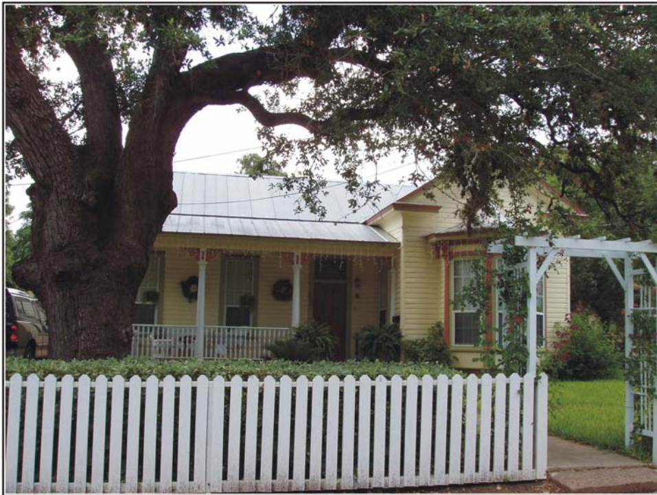
Figure 3-8. Photograph of 323 West Nolte Street.
