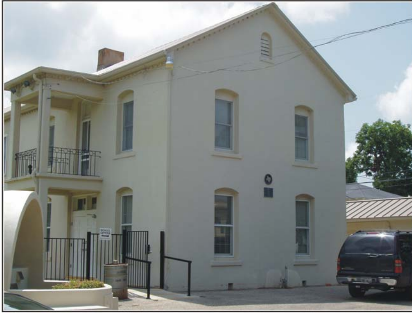
Figure 3-11. Photograph of the schoolhouse at St. James Church.
