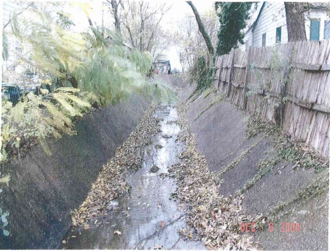
looking upstream from Wisconsin St
