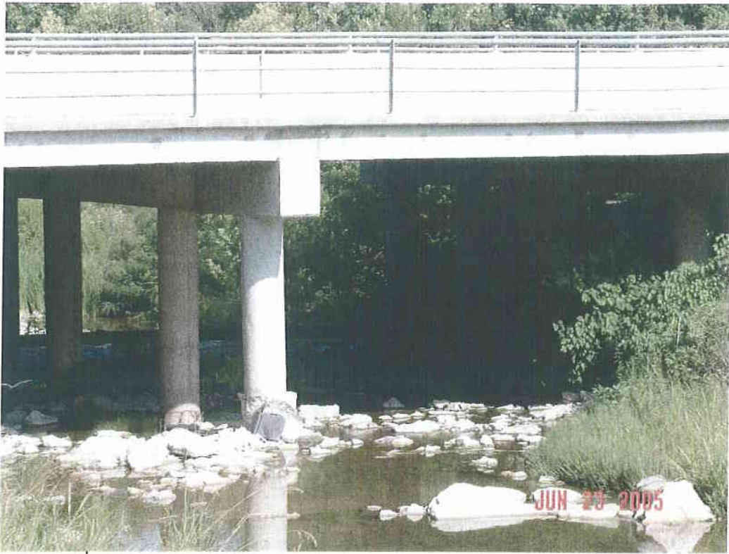
Under 2 nd St bridge
