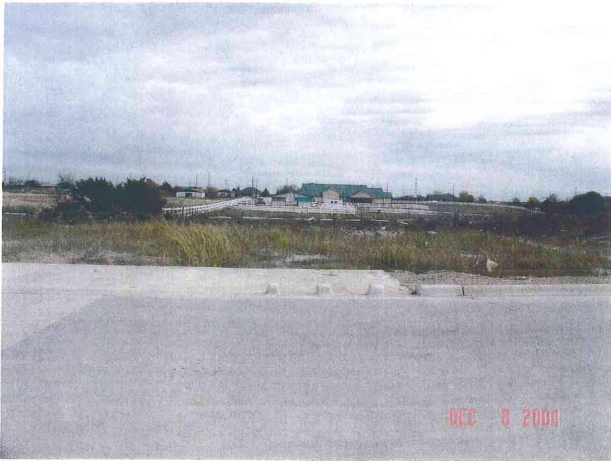
Detention pond in Saegert Ranch
