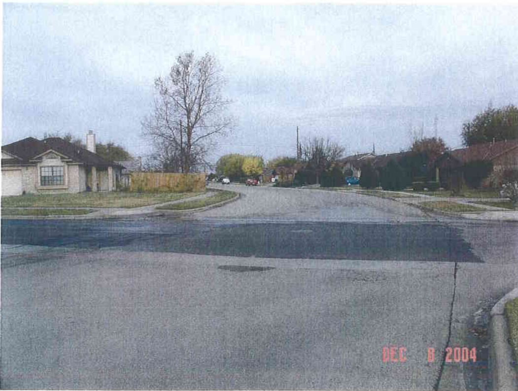
Gutter flow at GreenLee Dr and Honeysuckle Dr
