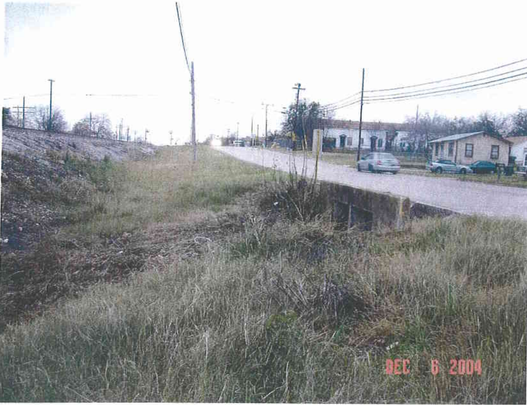
Downstream face of Norris St culverts
