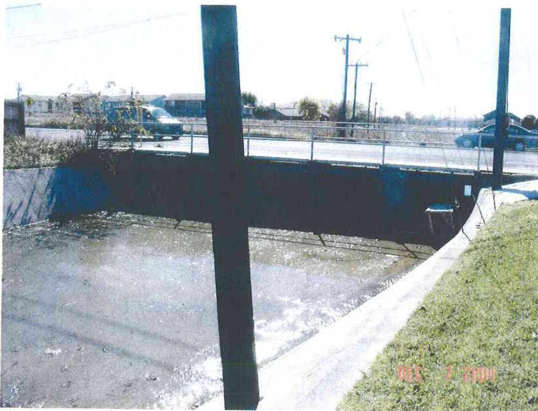
Upstream face of Westcliff Rd culvert
