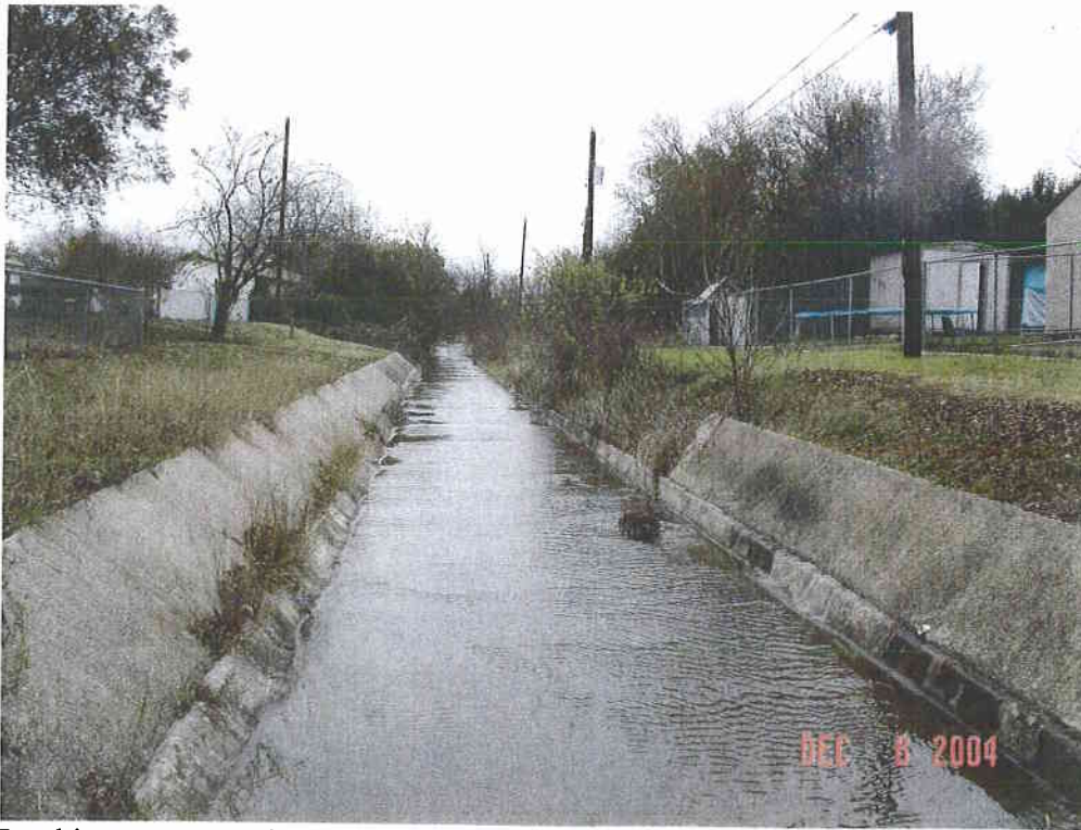
Looking upstream from Greenwood Ave flume
