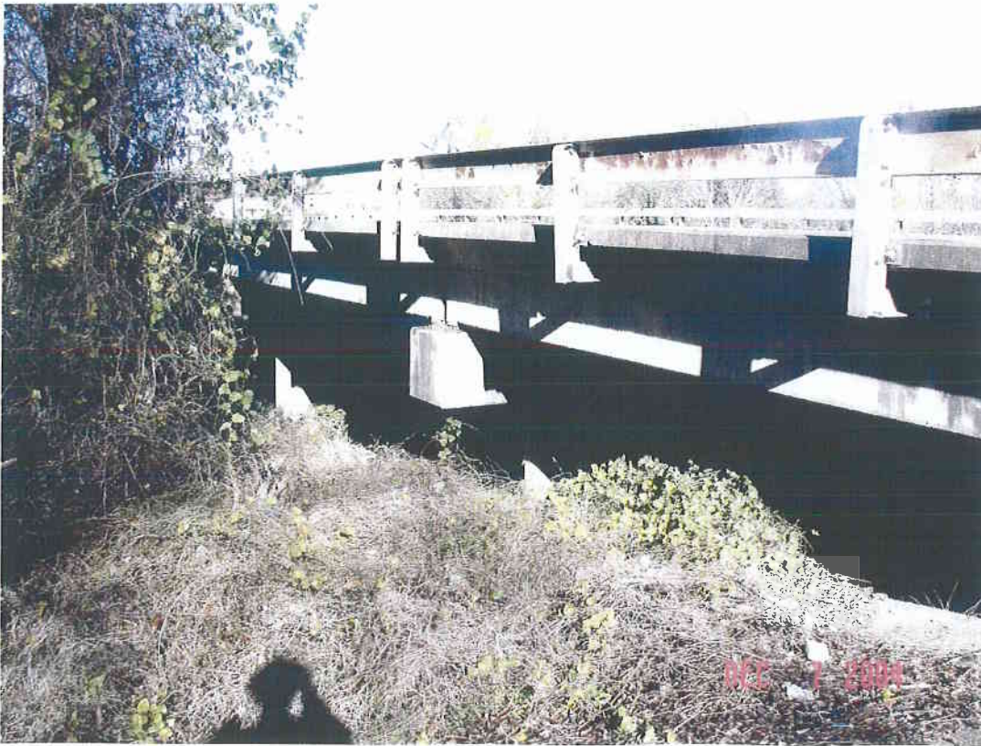
Upstream face of Little Nolan Creek bridge at SH 190
