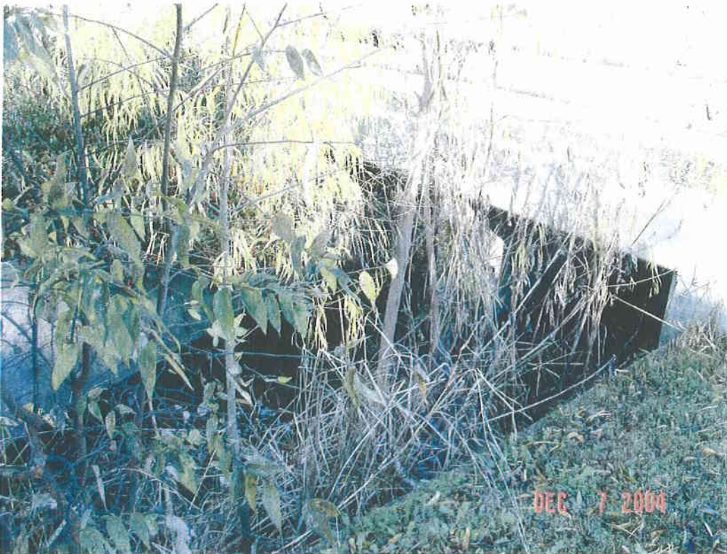
downstream face of Trotwood Tr culvert
