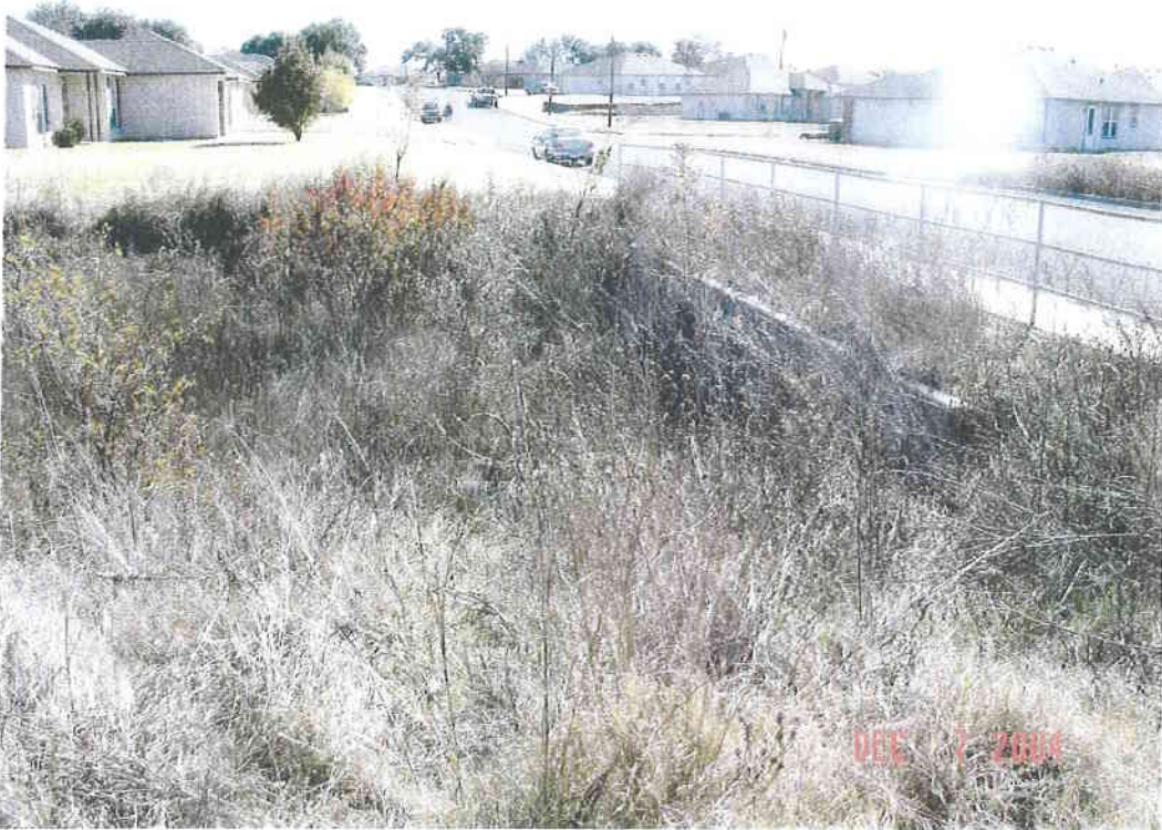
Upstream face of Ridgehaven Dr culvert
