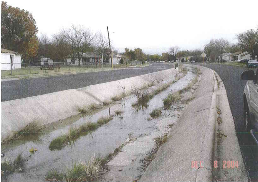
Looking upstream Valley Ditch
