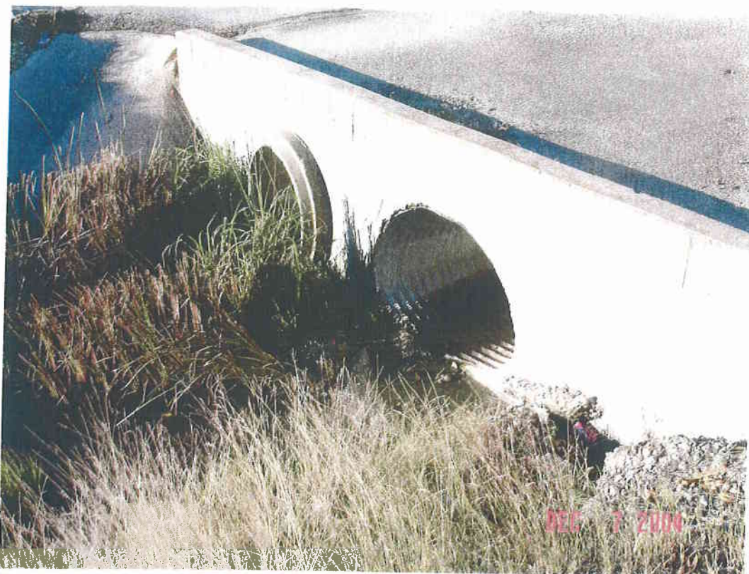
Downstream face of Branch Dr culverts
