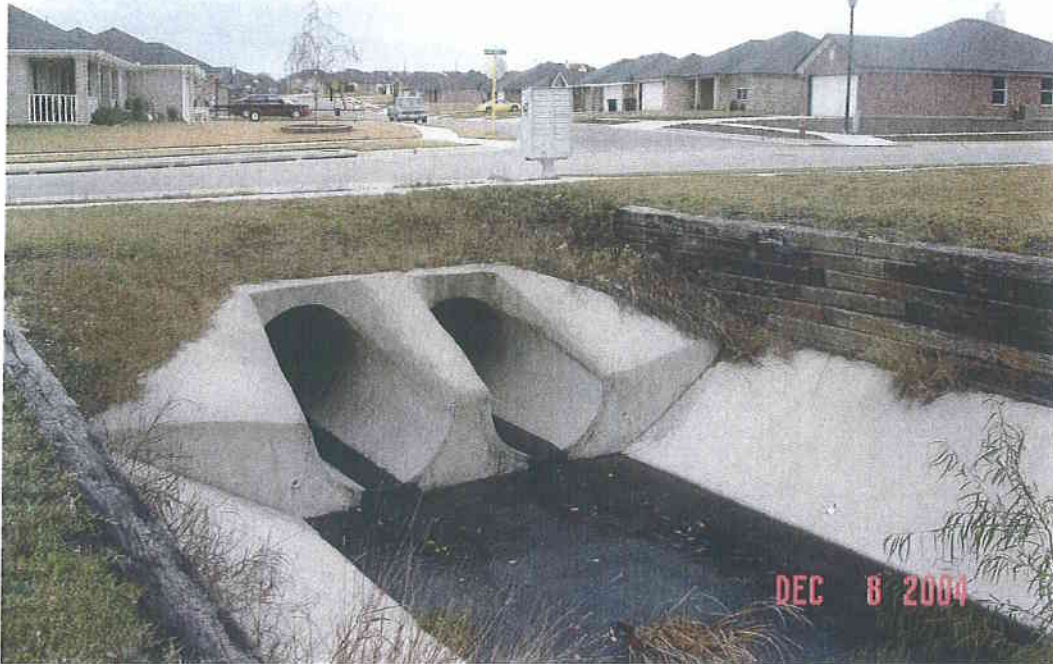
Storm sewer discharge
