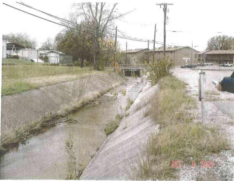
looking downstream Stewart Ditch at Harris Ave
