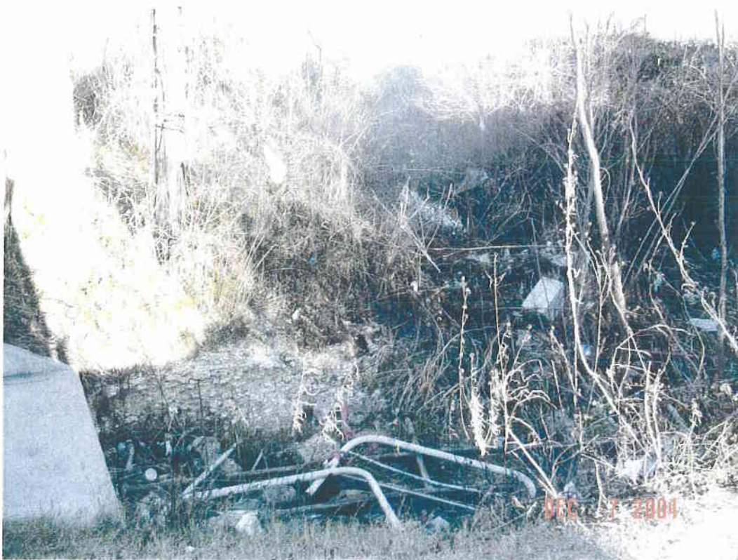
end of flume at Cantabrian & Valencia St.
