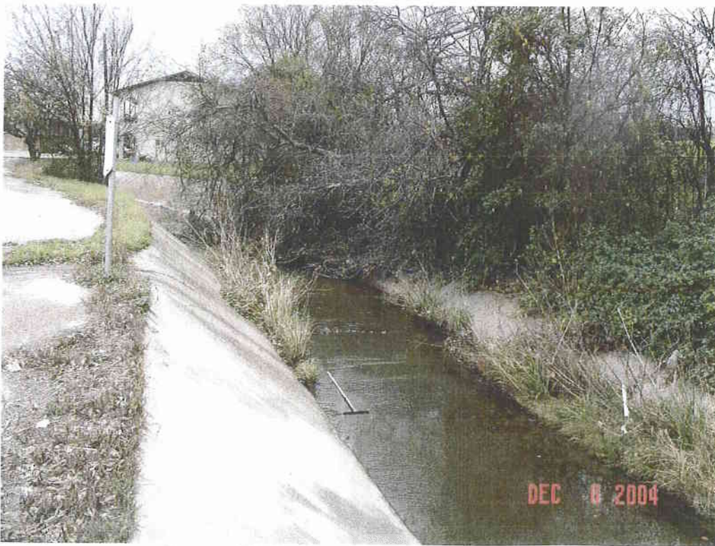
looking upstream Stewart Ditch, downstream of Rancier Ave
