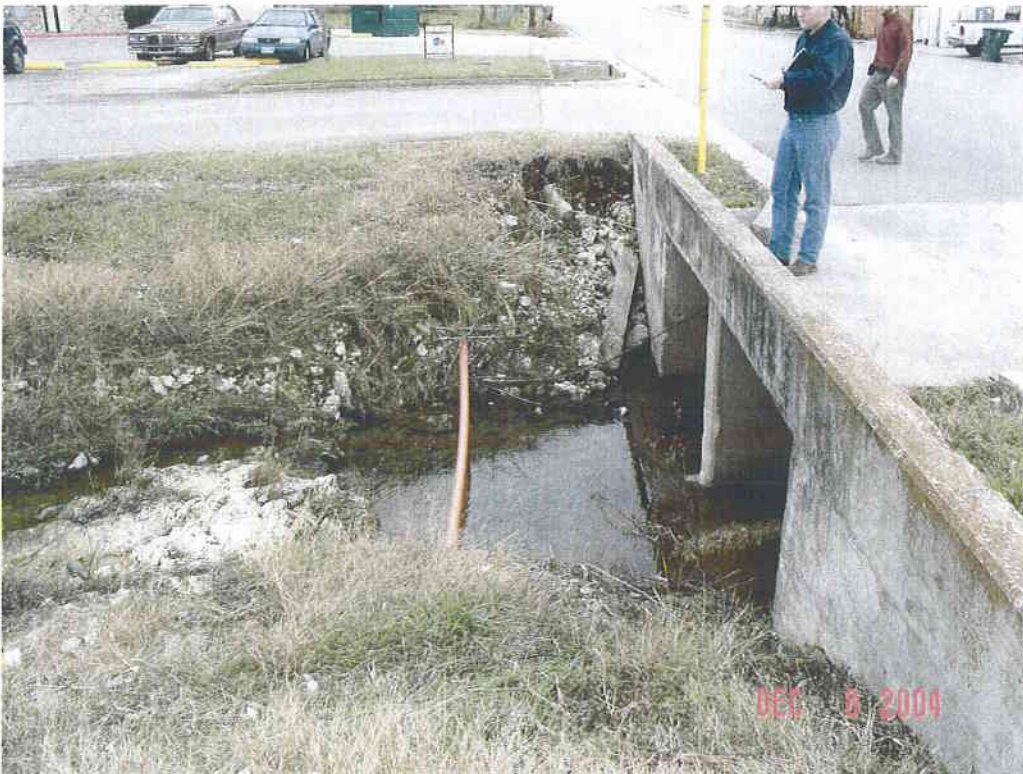
Upstream face of Atkinson Dr culvert
