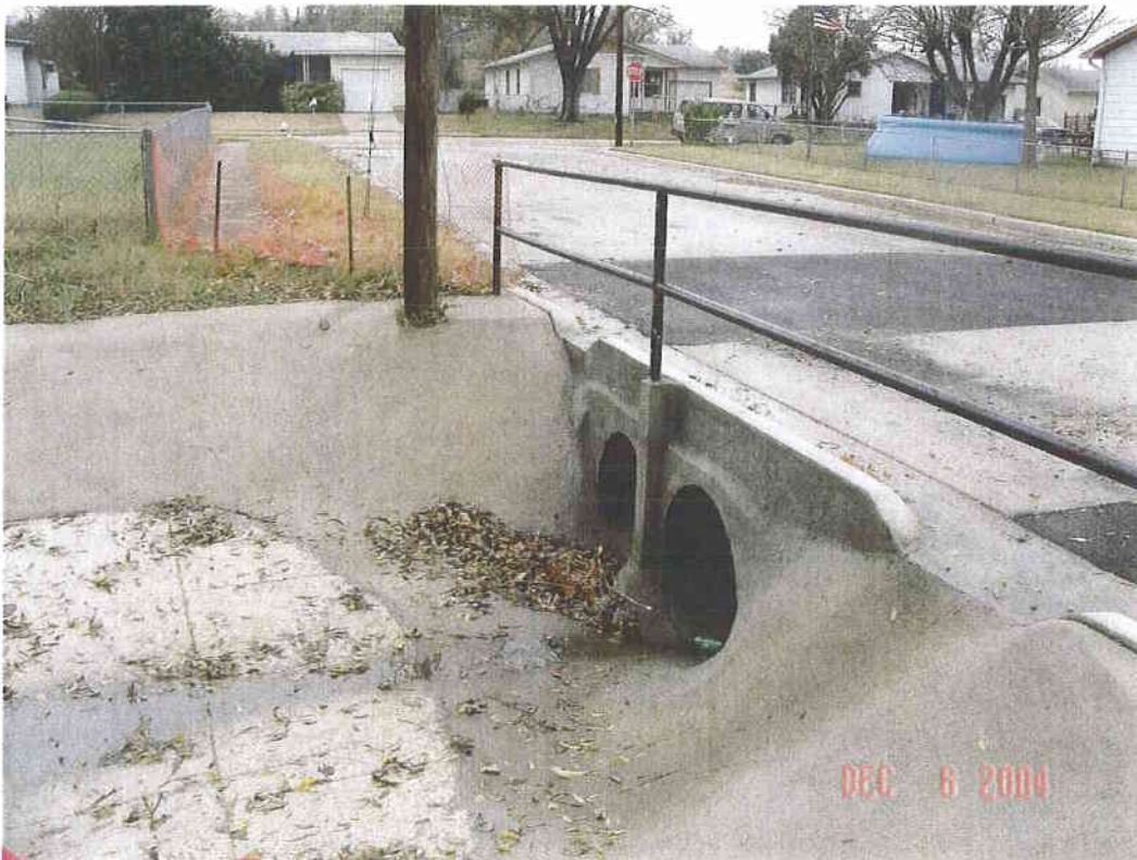
Upstream face of Short Ave
