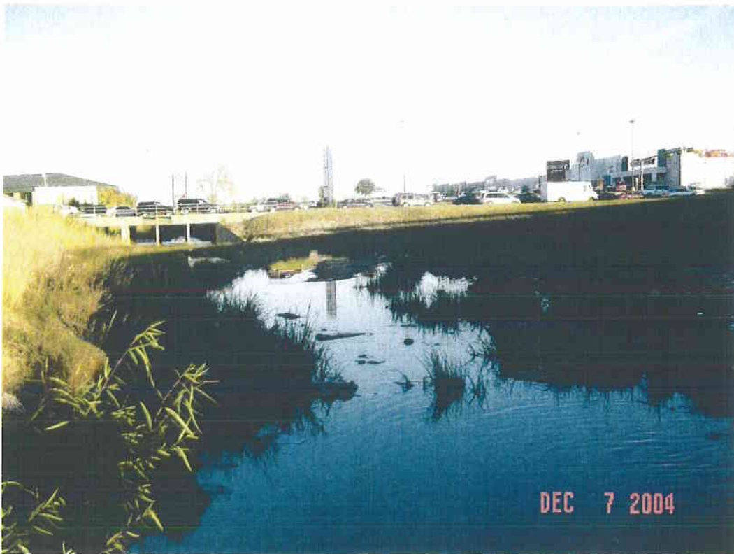
Culvert at WS Young, upstream side
