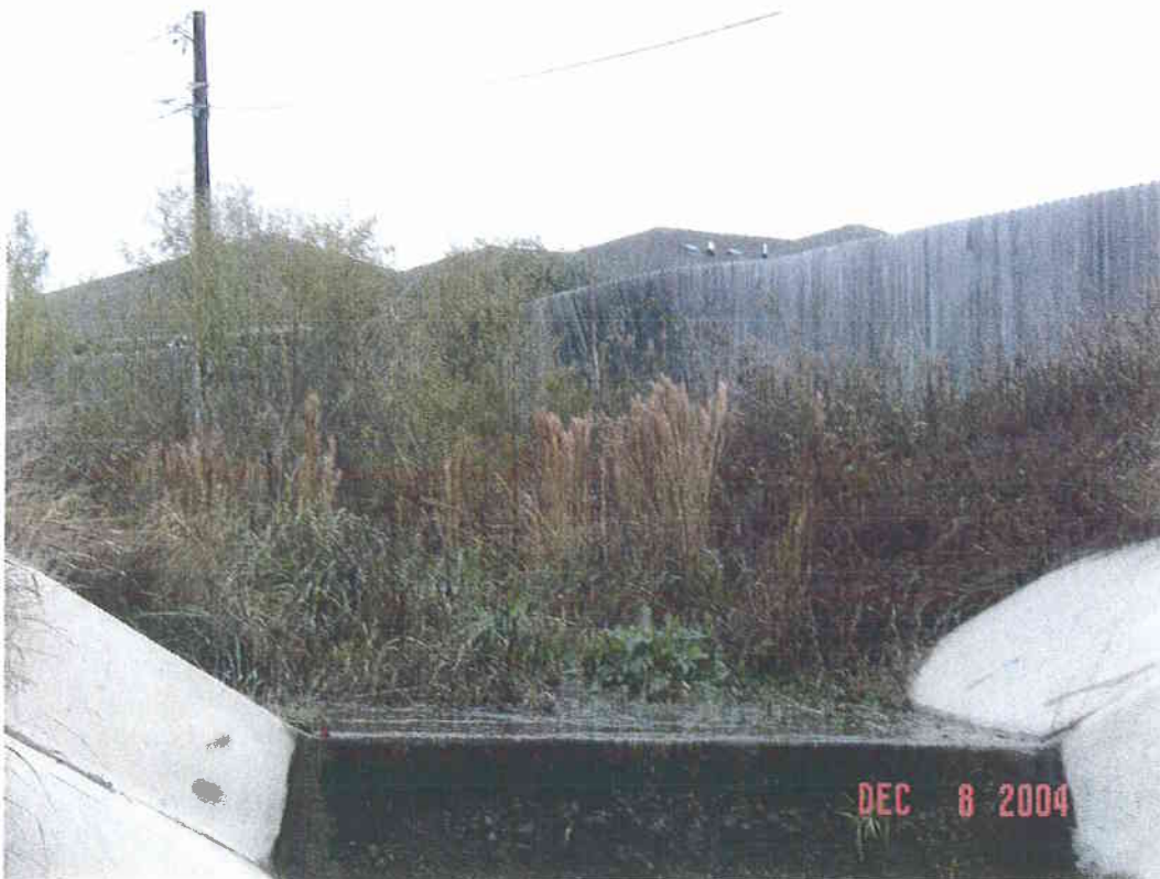
Upstream at earthen channel into drop structure
