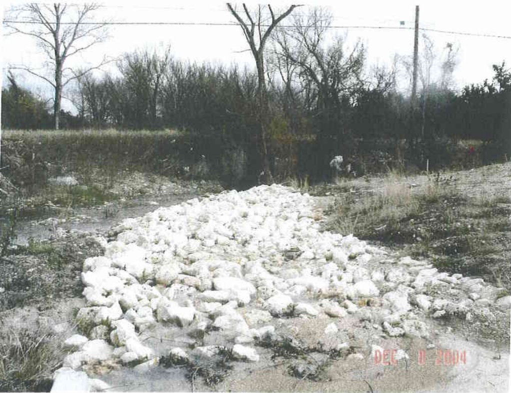
View of culvert under Onion Street. Rock rip rap for Rio Grande St flume.
