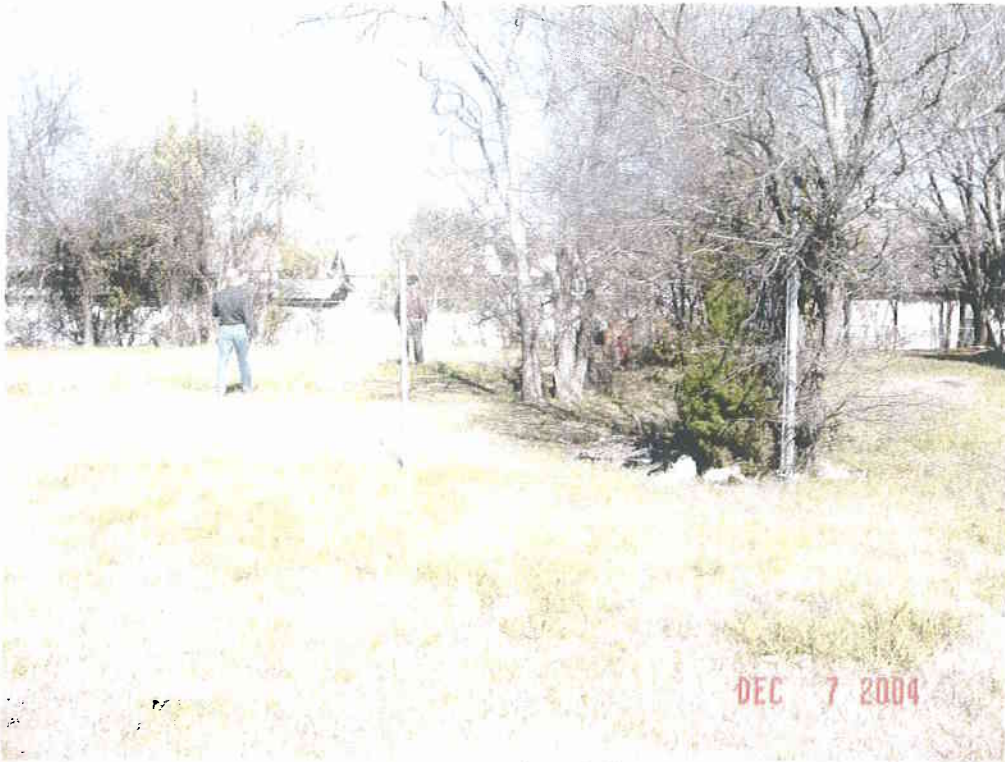
Street flow from Zephyr Rd overtops curb and flows through this vacant lot
