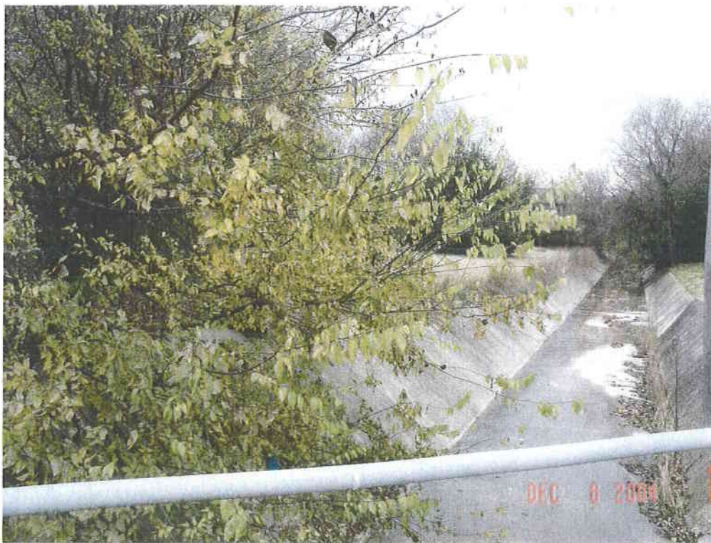
Stewart Ditch Trib downstream of 12 th Street
