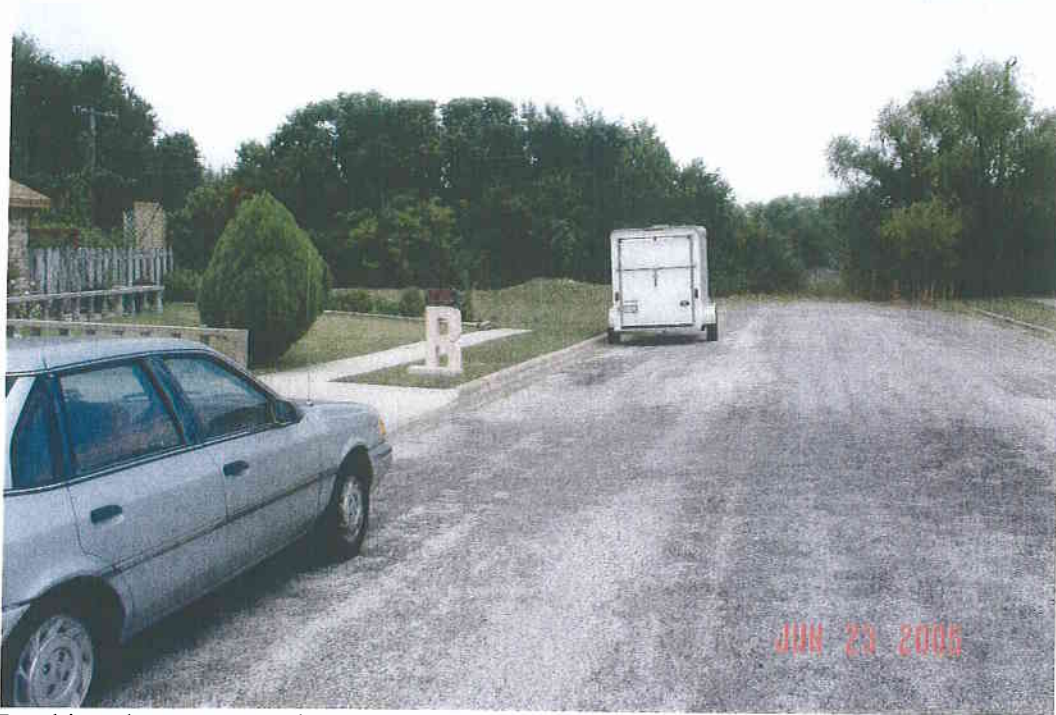
Looking downstream along El Dorado Dr
