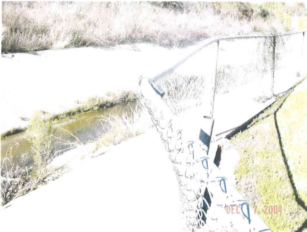
Top of concrete slope exposed
