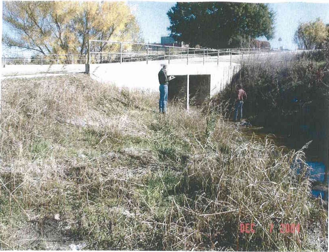
Downstream face of Hilliard Ave culvert
