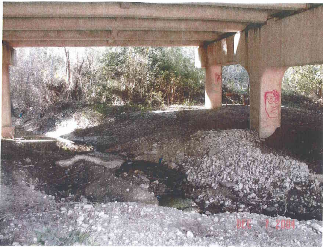
Flow from Dogwood channel directed under bridge
