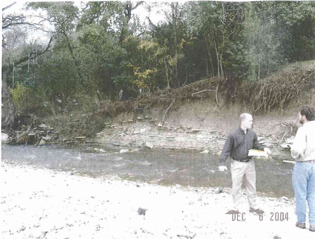
Downstream bank erosion continues
