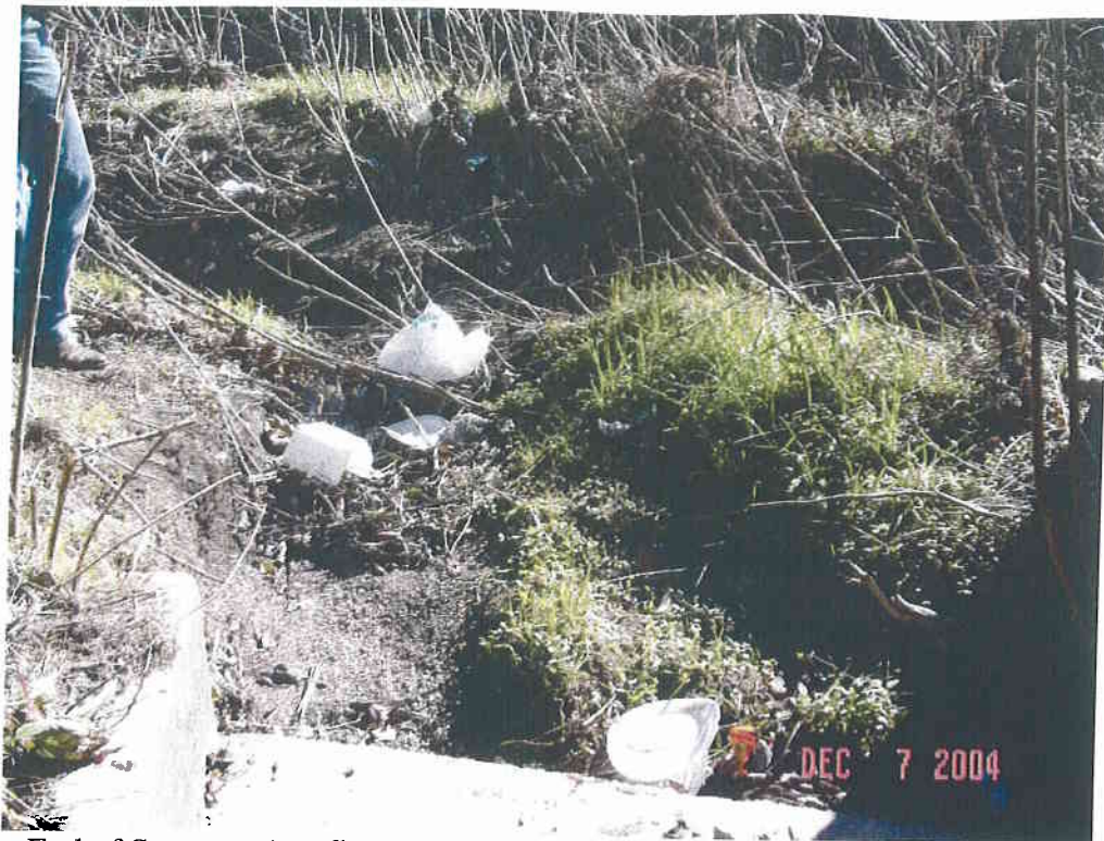
End of Saratoga Ave flume
