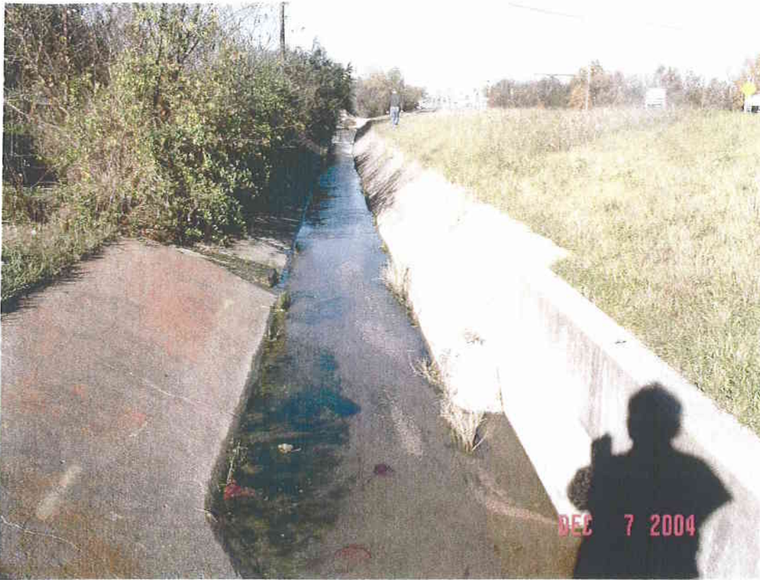
Concrete channel along SH 190
