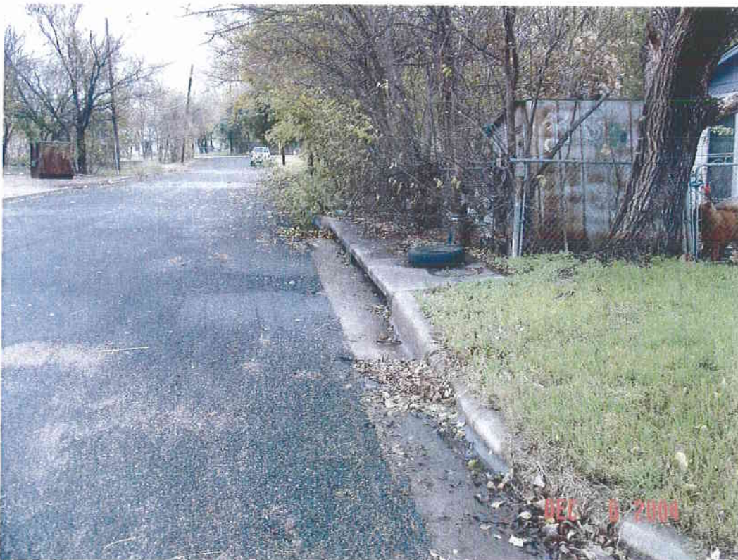
Curb inlets on Utah Street just north of Adams Ave.
