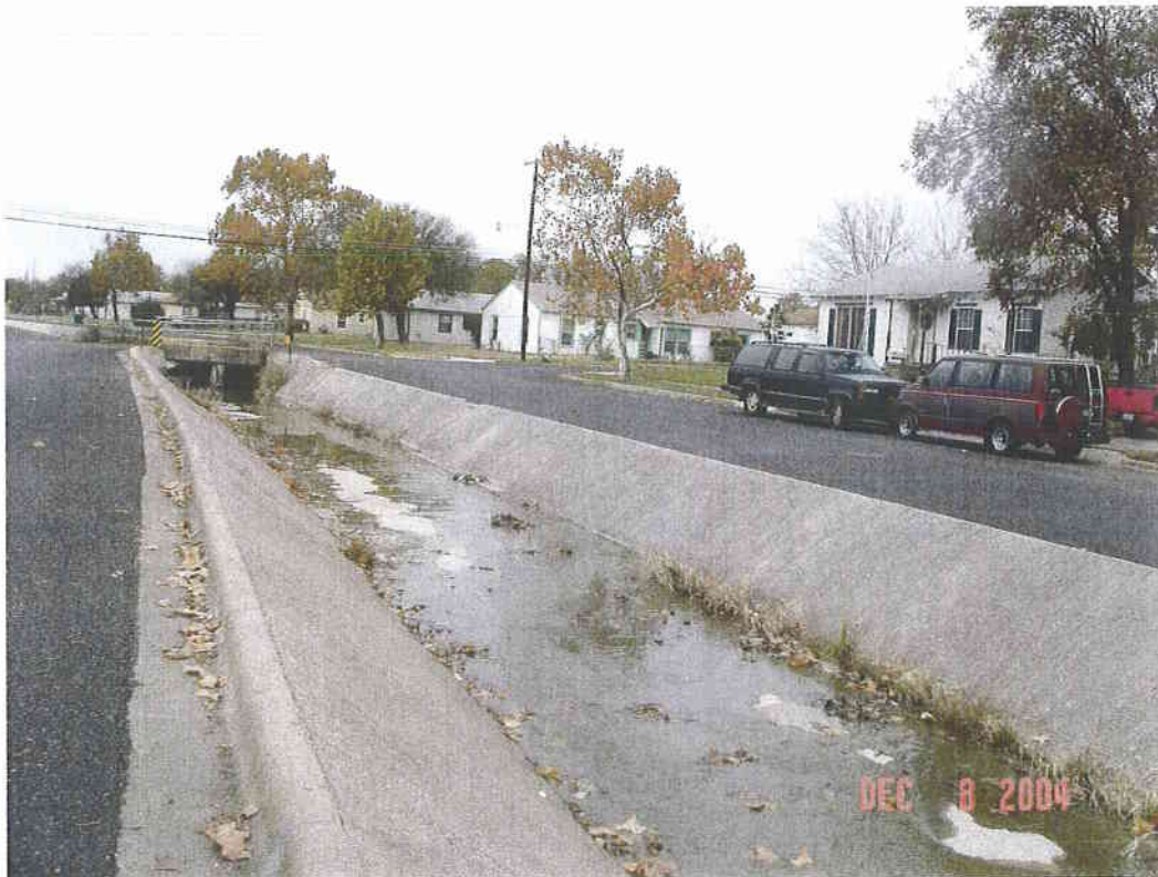
Looking upstream at Hillcrest Dr
