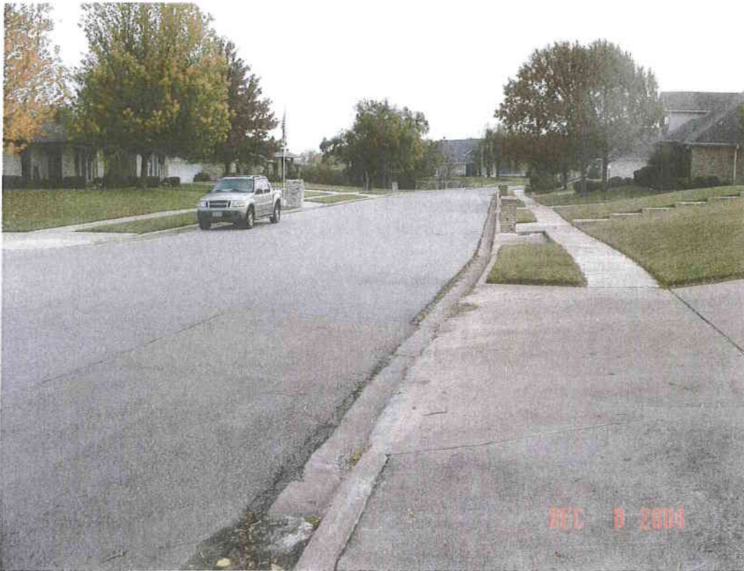
Looking east from golf course ditch and curb inlet
