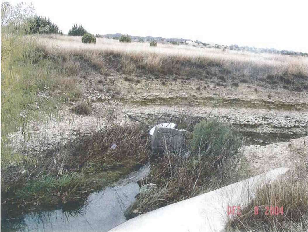
end of concrete channel
