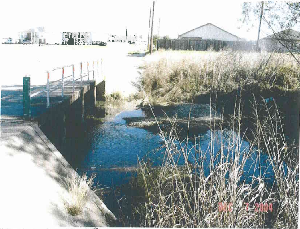
downstream face of N. 38 th Street culverts
