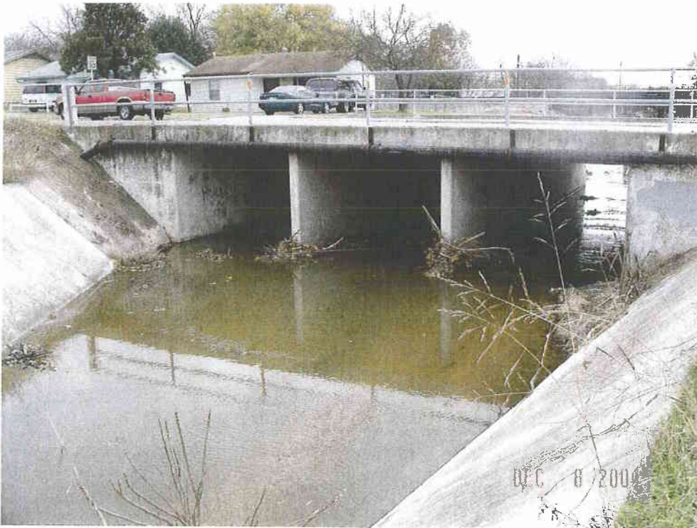
Upstream face of Greenwood Ave culverts
