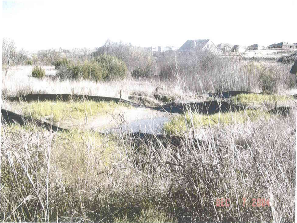
SWPPP Failure in new development
