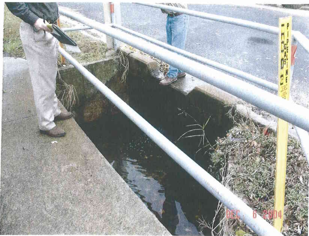
Downstream face of culvert
