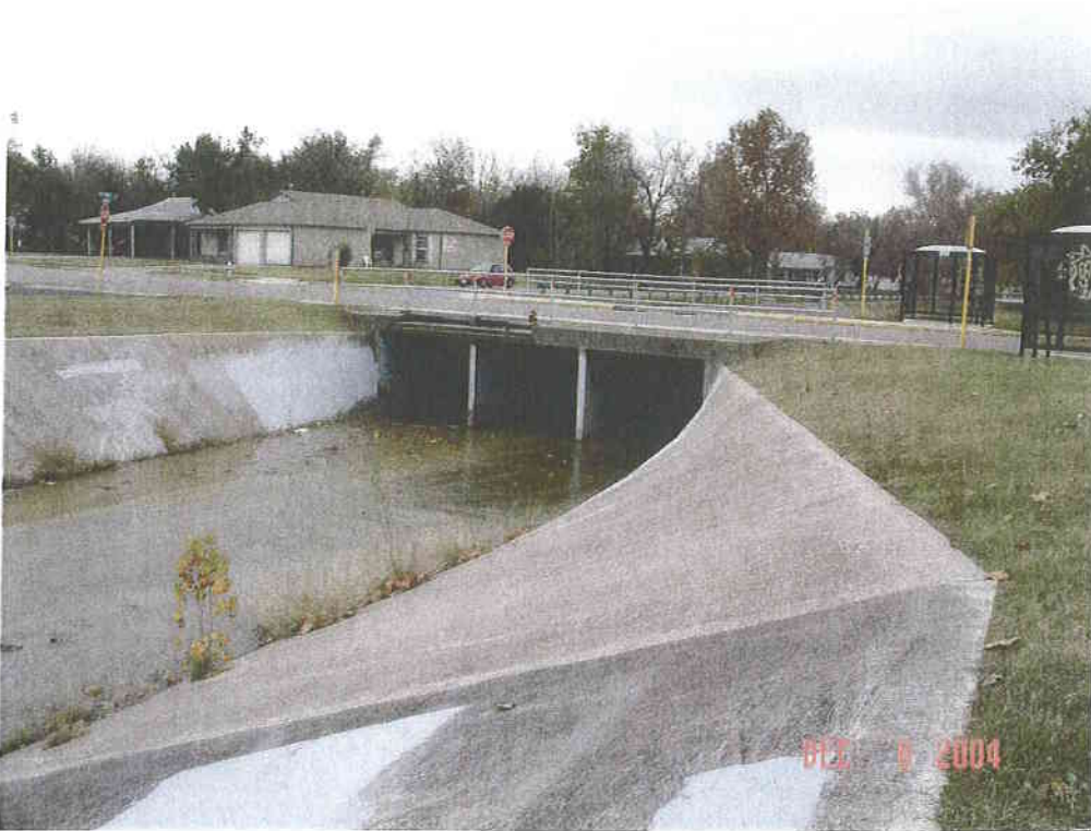
Downstream face of Culp Ave culvert
