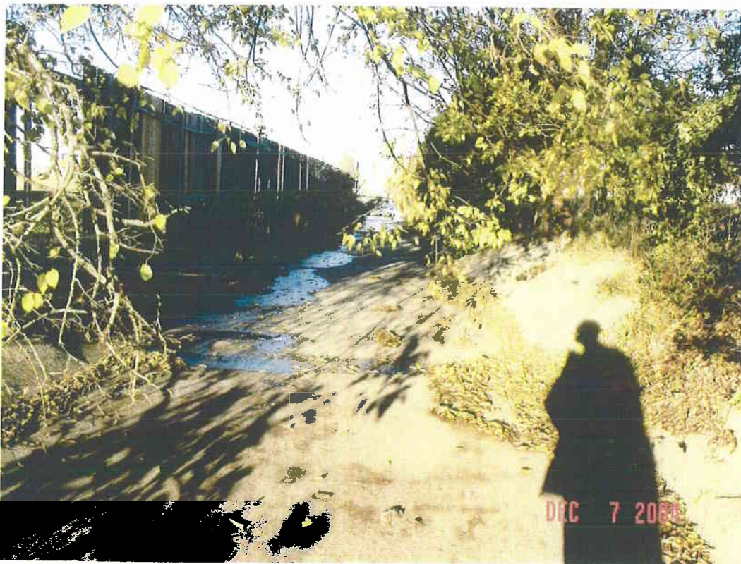
Upstream concrete channel into park
