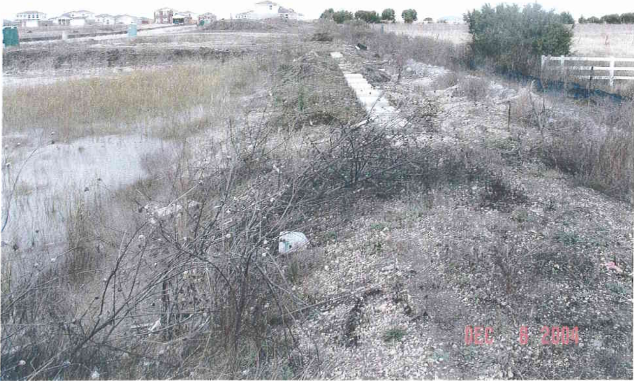
view of outlet structure
