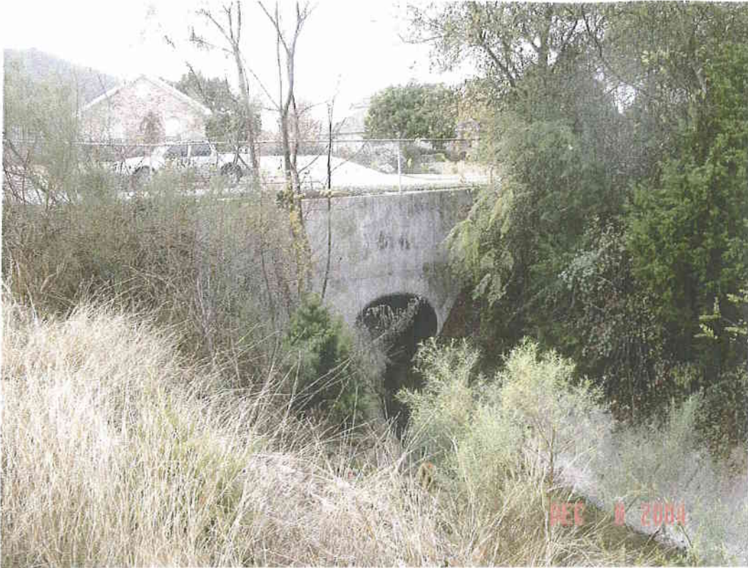
Downstream face of Stillwood Dr storm sewer
