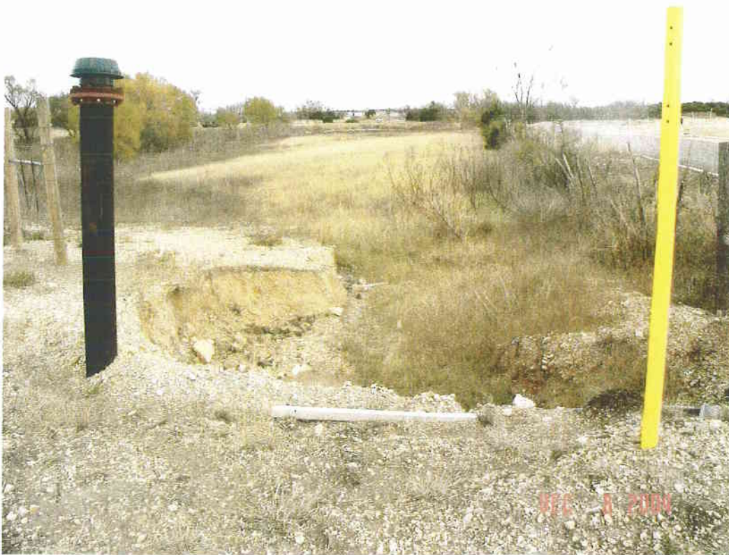
View downstream from Rio Grande culvert
