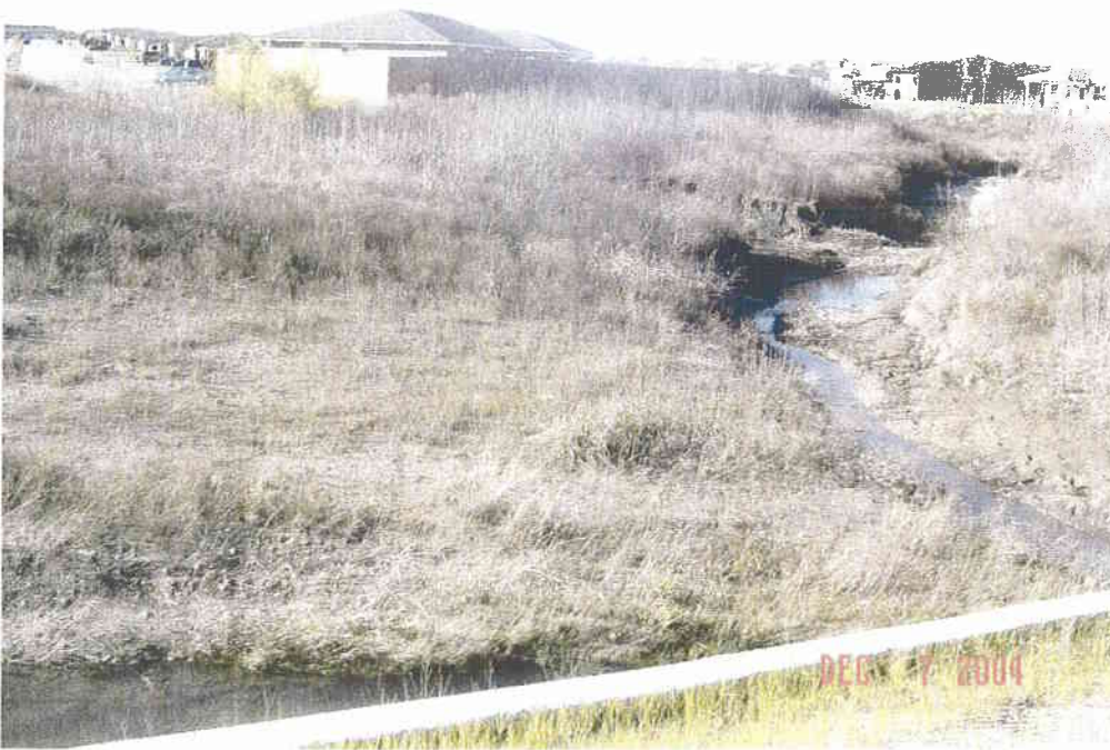
looking upstream SNC Tributary from Robinett Rd
