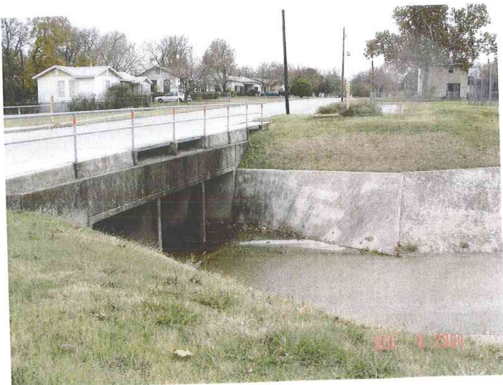
Upstream face of Culp Ave culvert
