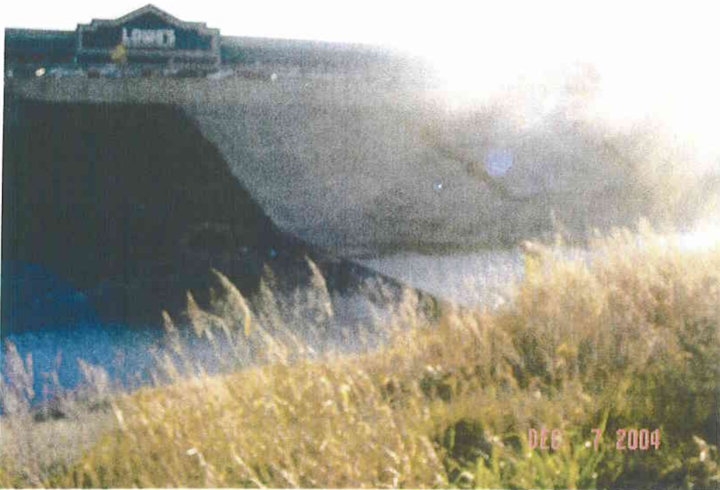
drop structure at Lowe's
