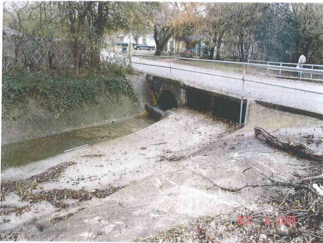
Culverts and channel
