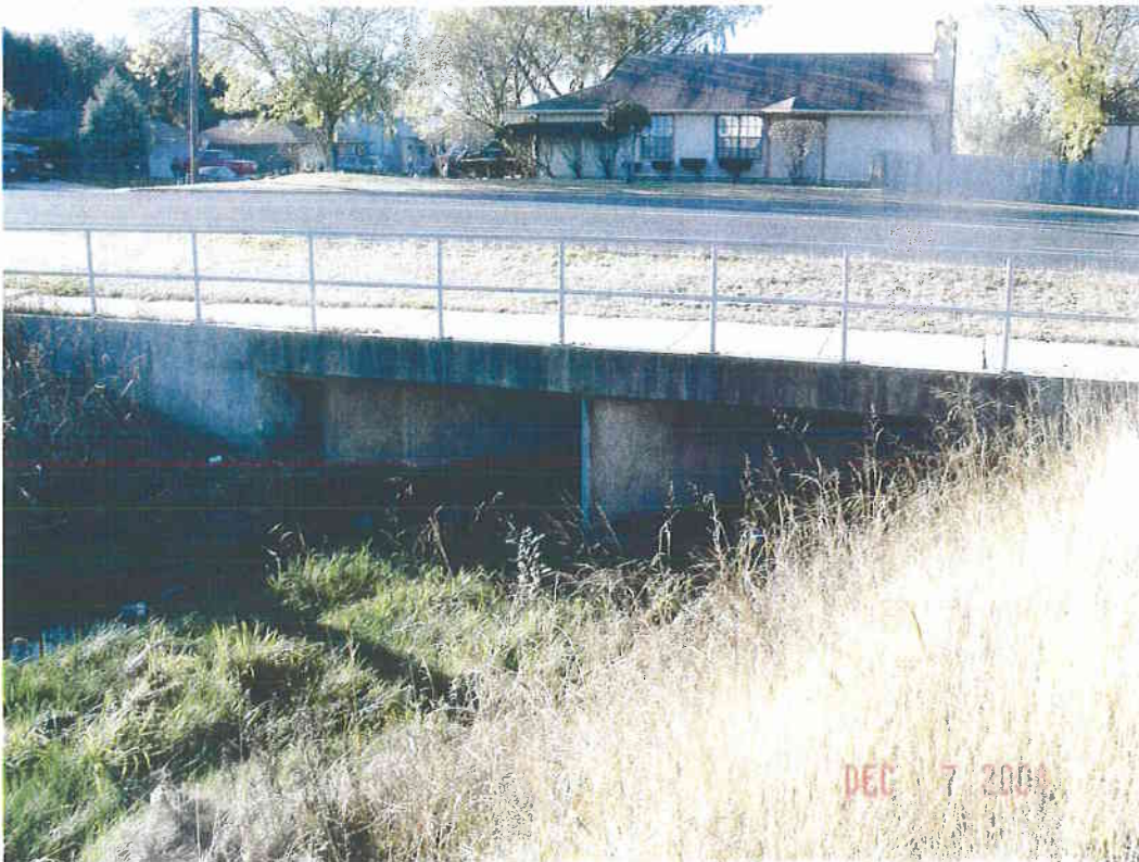
upstream face of Westcliff Rd culverts
