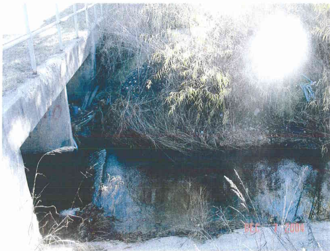
downstream face of Westcliff Rd culvert
