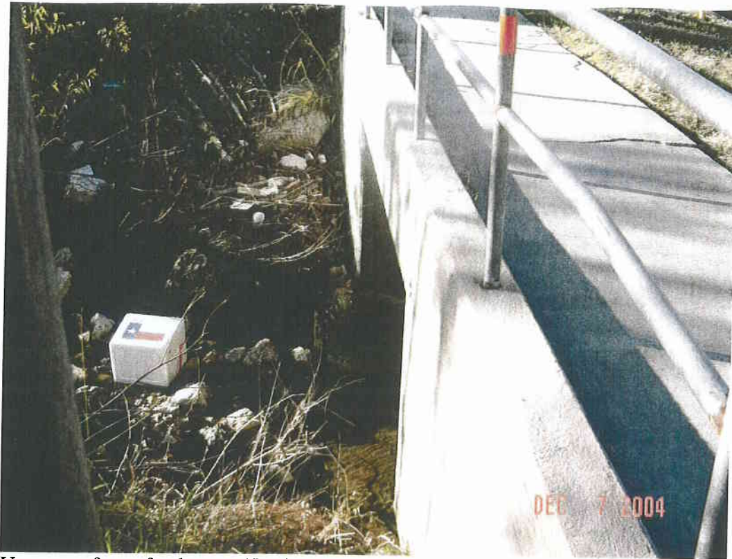
Upstream face of culvert at Turtle Creek Dr
