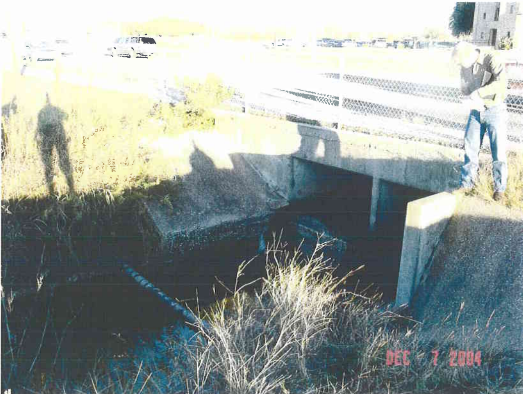
Downstream face of Rancier Ave culvert
