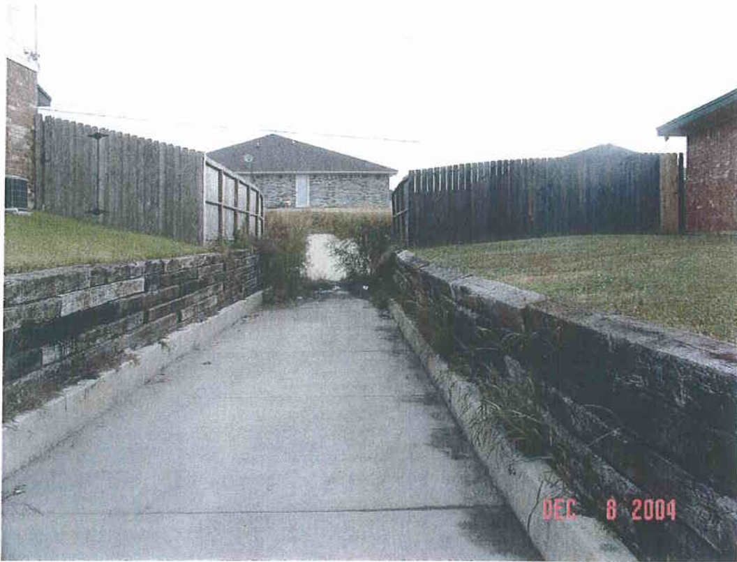
Looking down the flume from the road.
