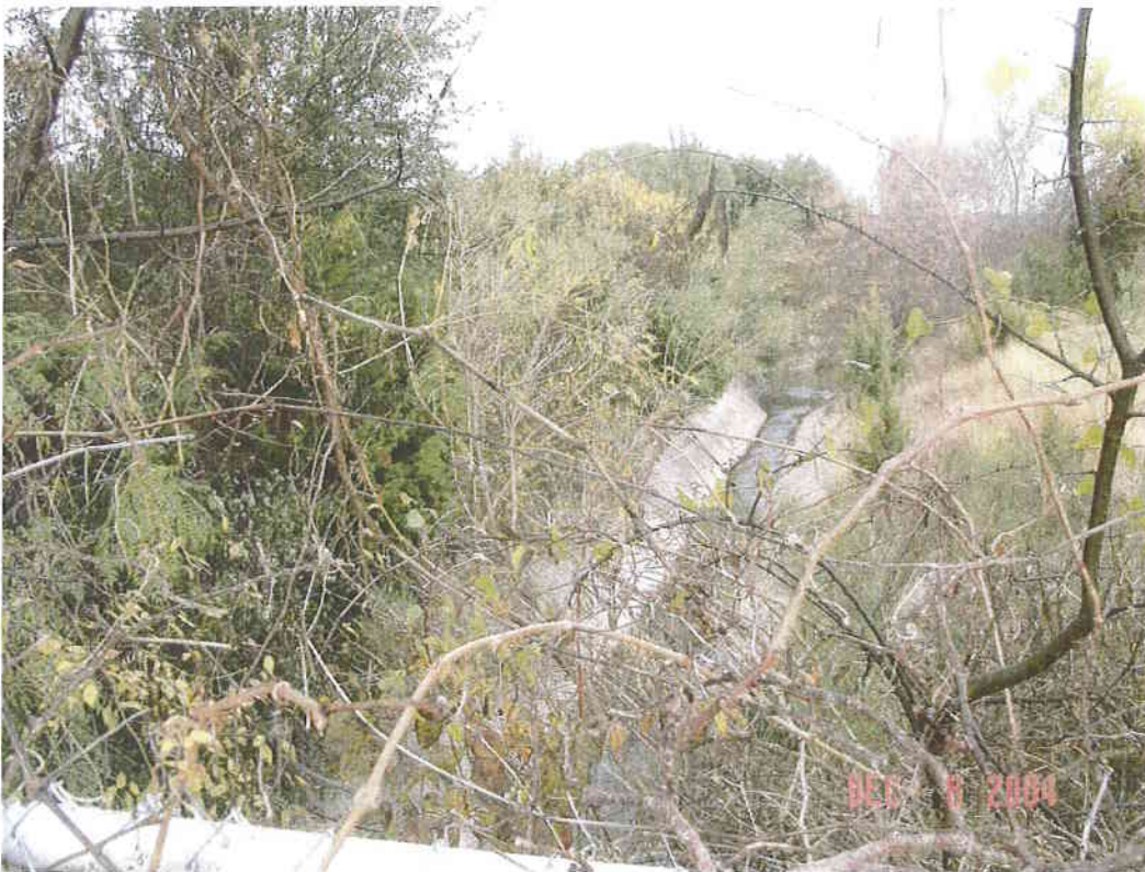
Looking downstream from Stillwood Dr, golf course ditch/ Stillwood storm sewer discharge
