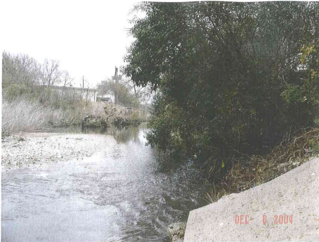
Looking downstream from concrete channel bank armoring, Odom Drive
