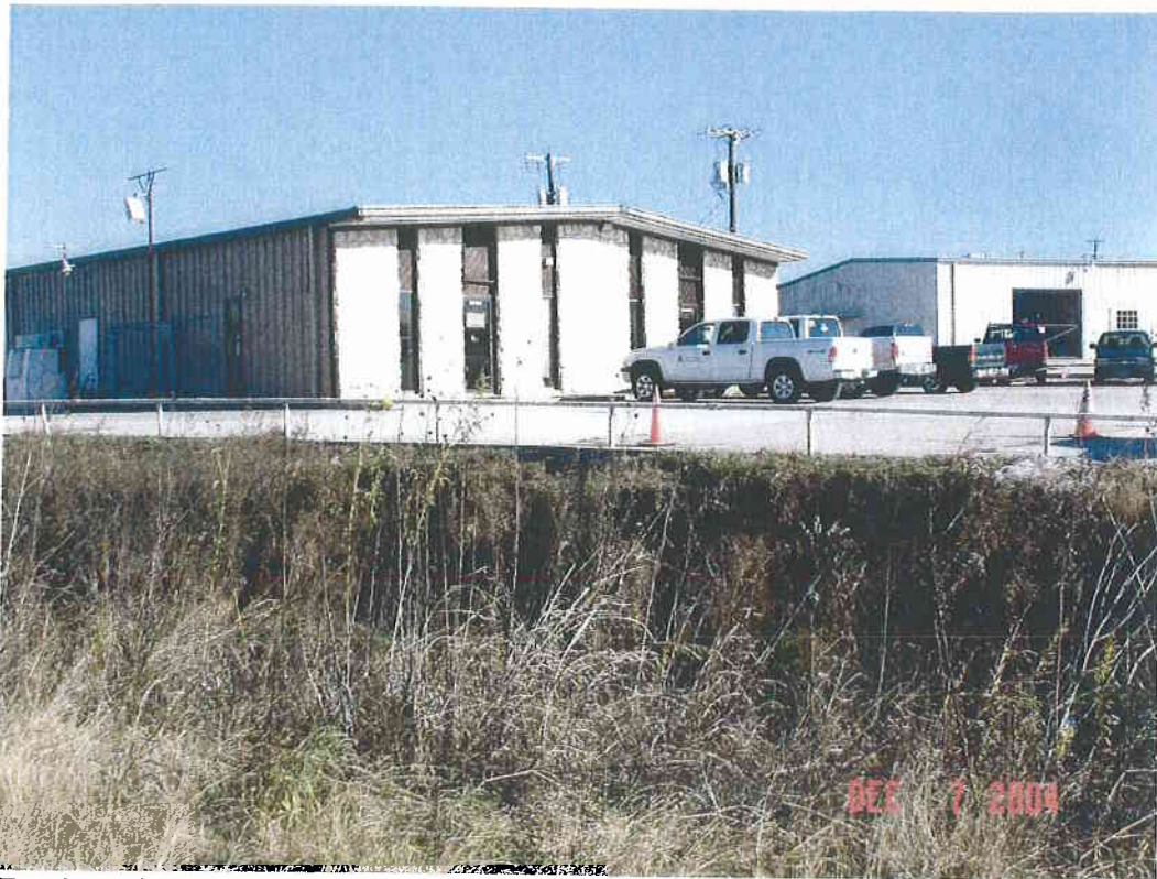
Erosion of bank just upstream of Jacobs Ln
