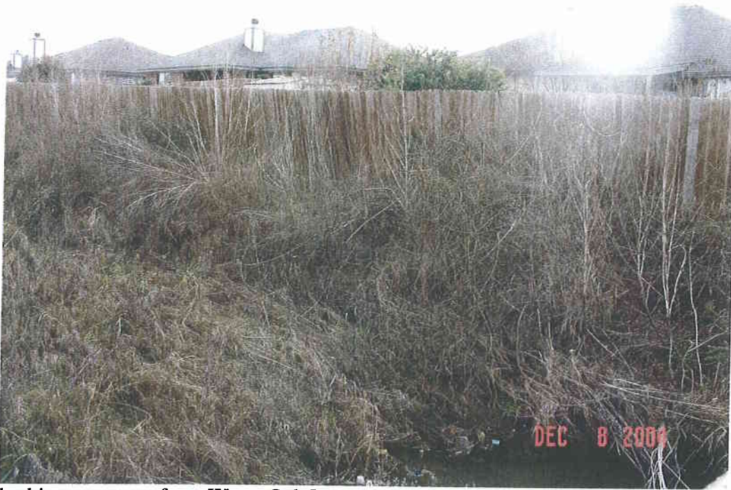
looking upstream from Water Oak Dr culvert, Embers Ditch East Trib
