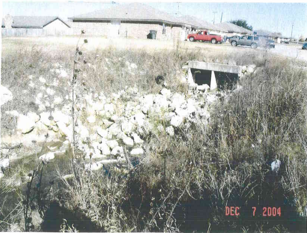
Downstream face of Long Branch Tributary culvert
