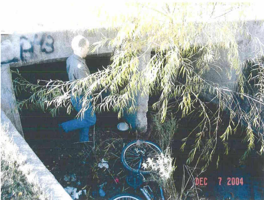
Upstream face of Trotwood Tr culvert
