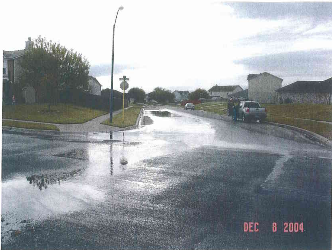
Down Misty Ln, significant street and gutter flow
