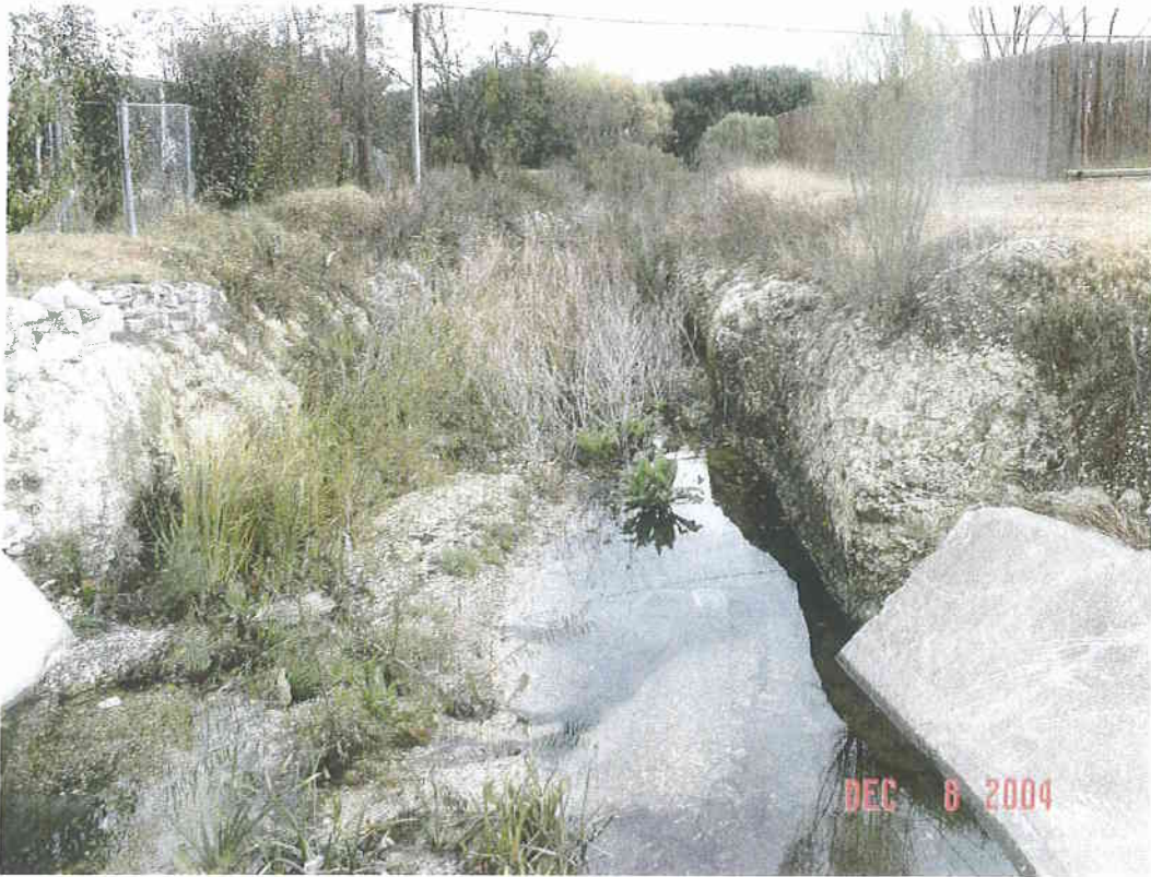
View downstream from Acorn Creek Trl culvert
