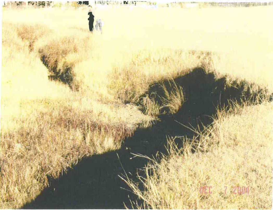
eroding banks of Long Branch Tributary
