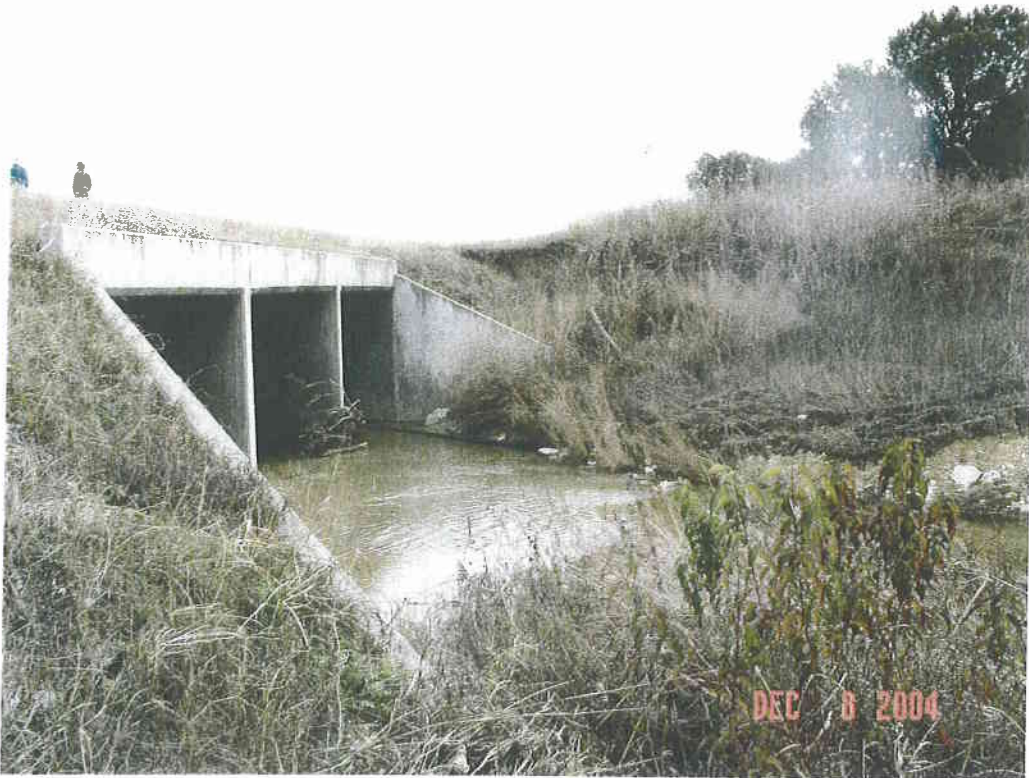
Upstream face of LNC culverts at Stan Schuetter Loop
