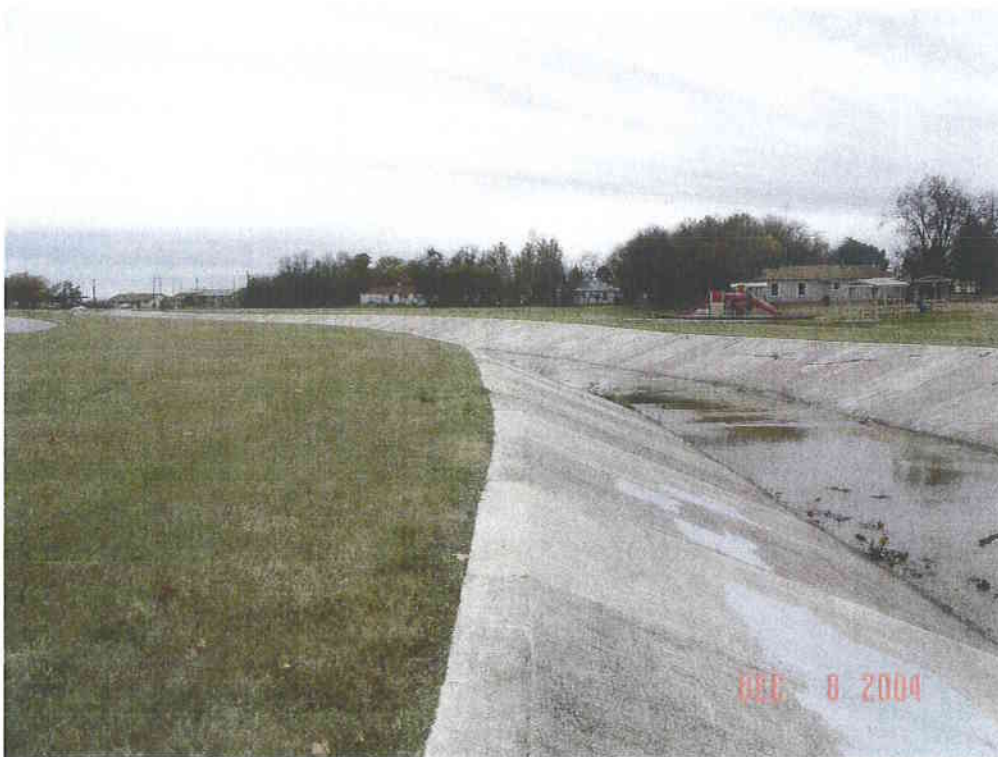
Looking upstream from Duncan Ave
