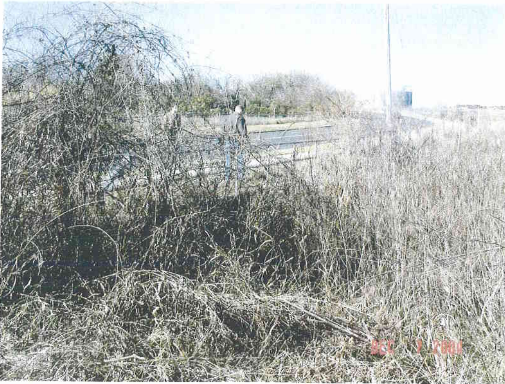
upstream face of Westcliff Rd. culvert
