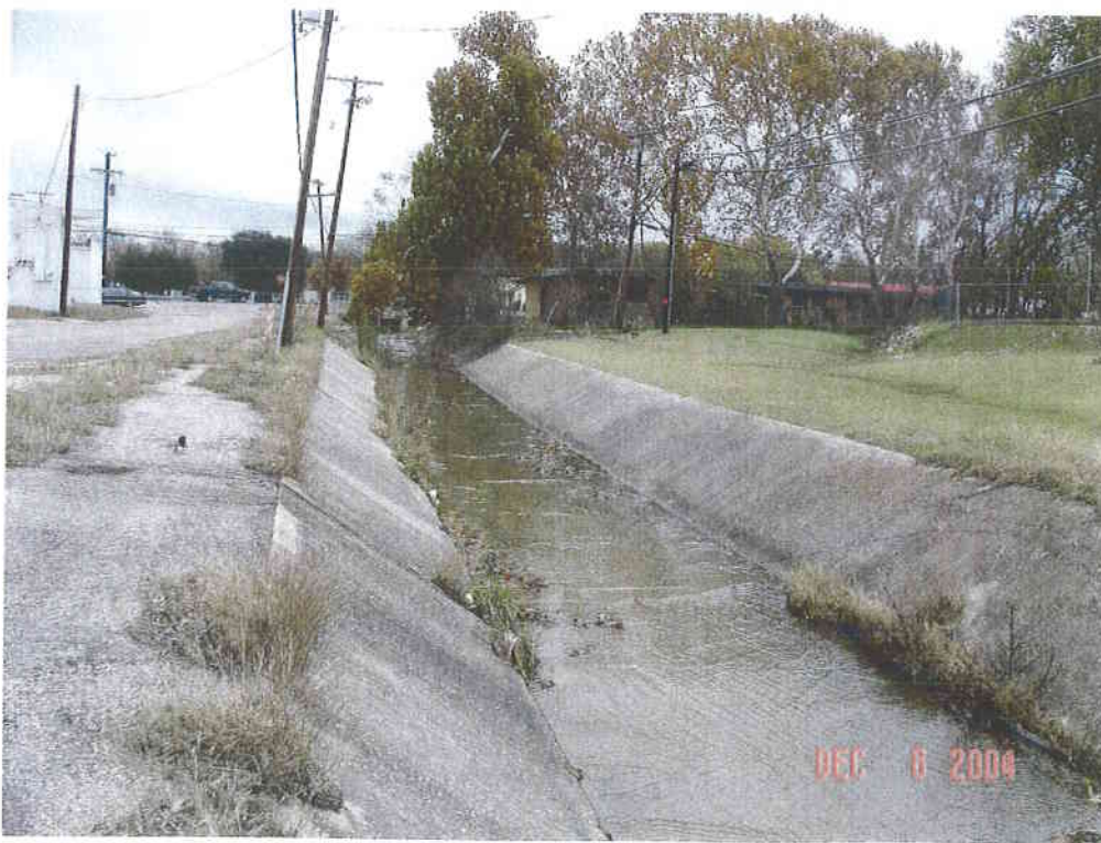
Looking upstream Stewart Ditch at Harris Ave
