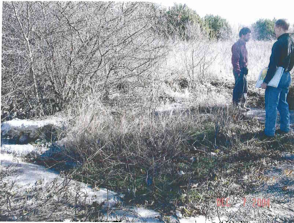
end of El Dorado Dr, street flows into drainage ditch to Long Branch
