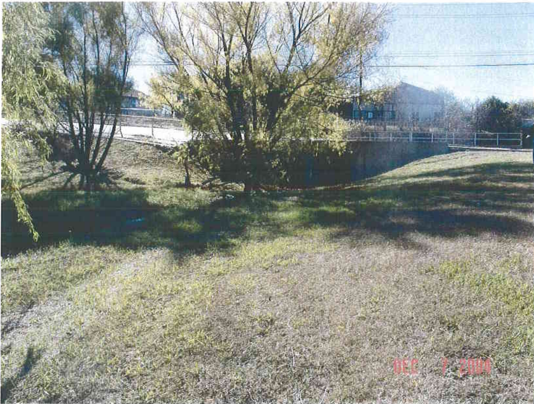
upstream face of Hilliard Ave culvert
