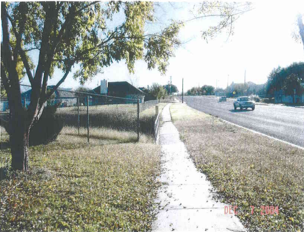
Looking east along Westcliff Rd, sidewalk depressed
