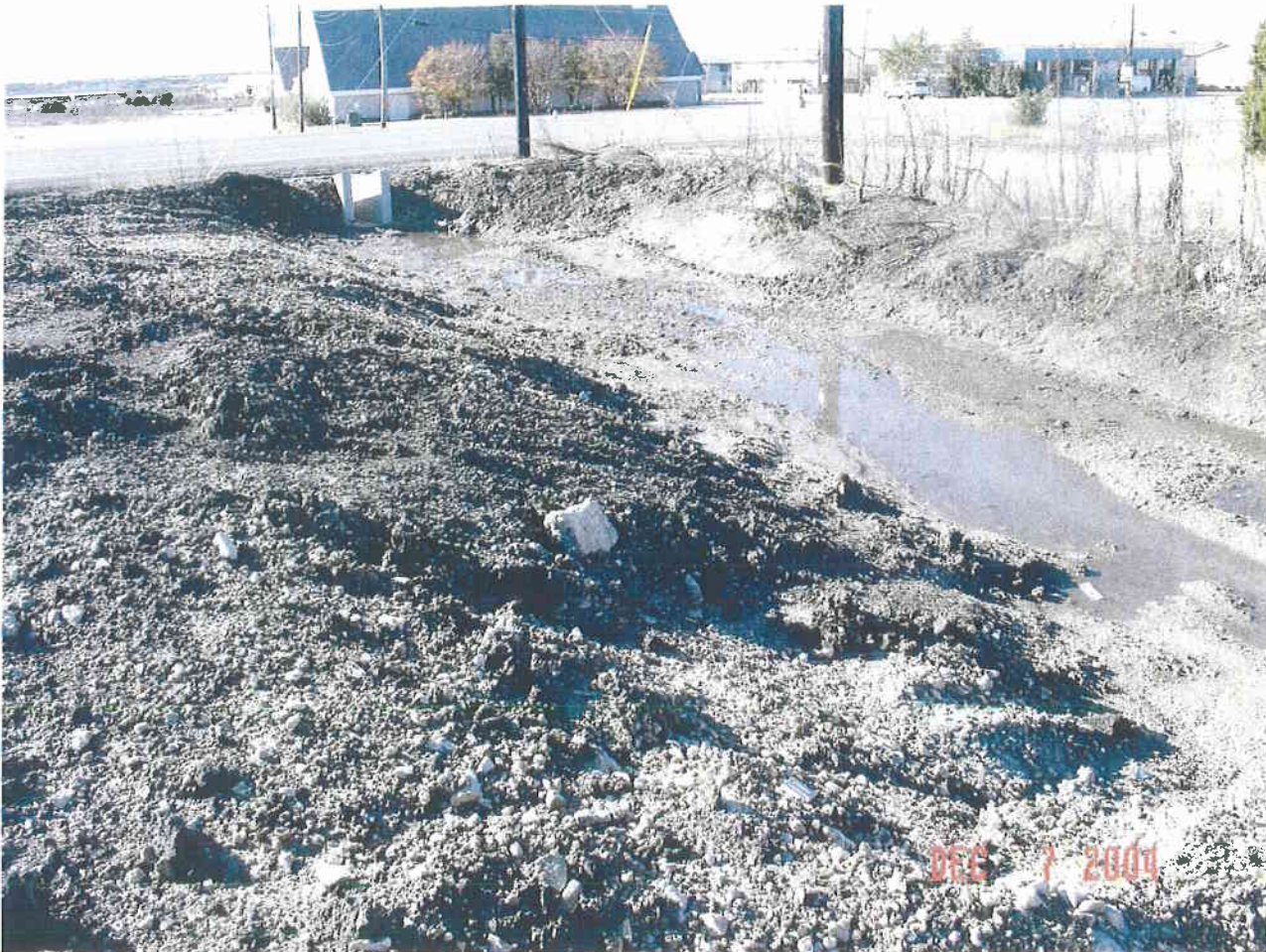
Outlet to ditch along road
