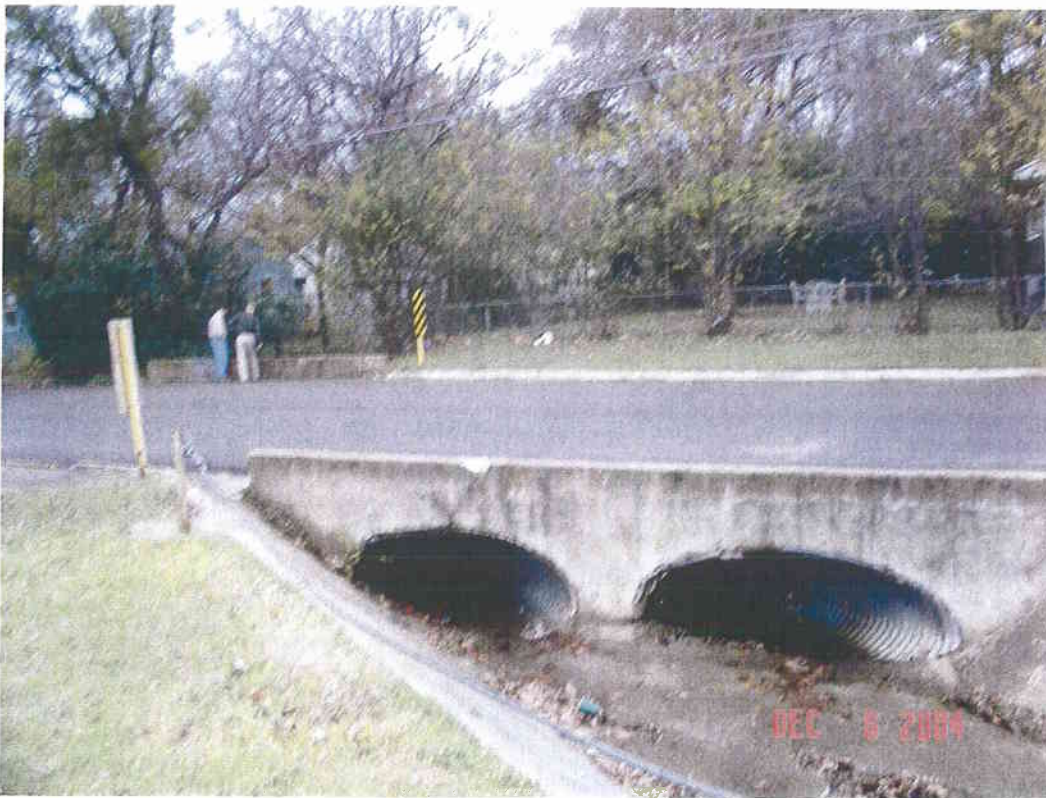
Downstream face of Gilmer Ditch culverts at Ave C
