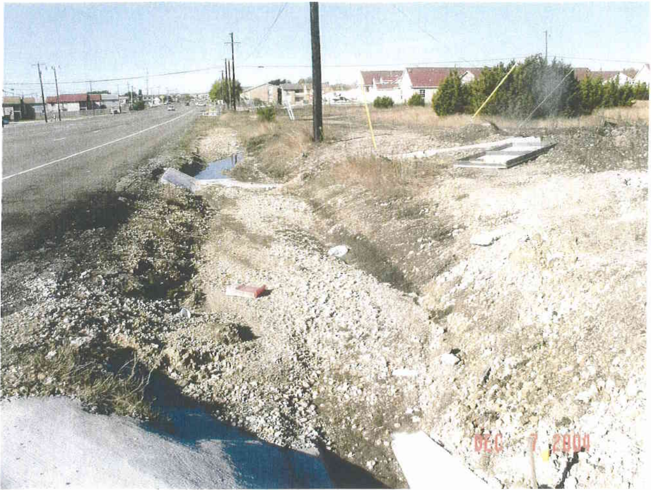
down the ditch
