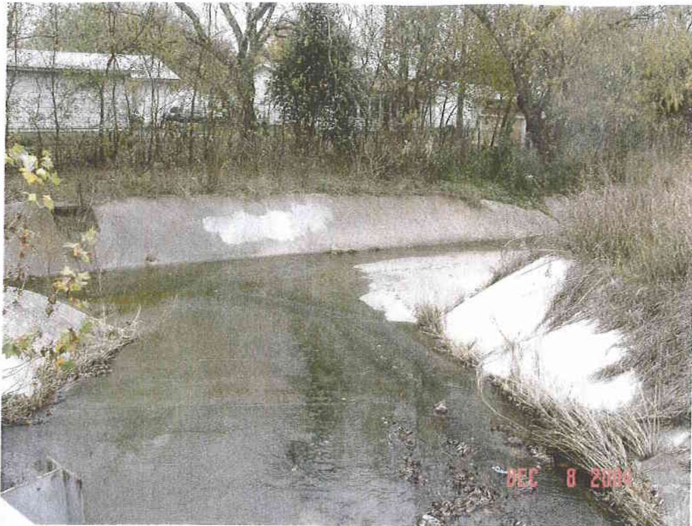
looking downstream at confluence of Stewart Ditch and Stewart Ditch Trib
