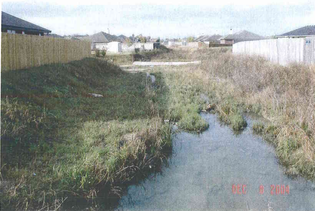
Embers Ditch East Trib, from Water Oak Dr, West Trib across Embers Ditch
