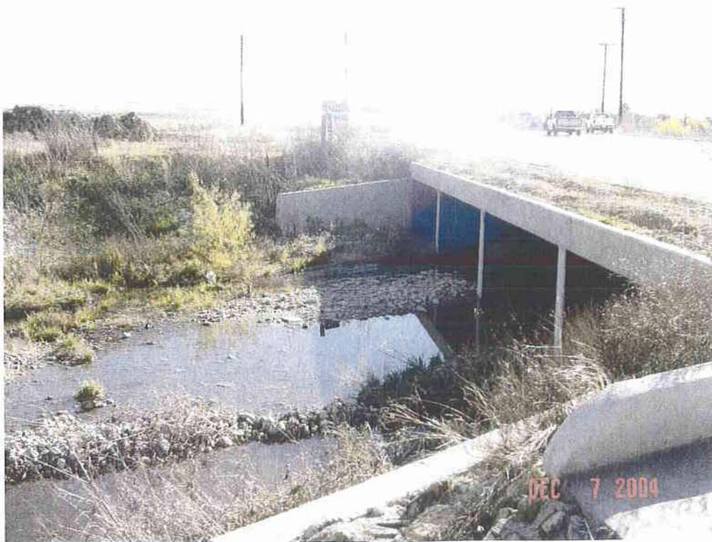
Downstream face of Robinett culverts
