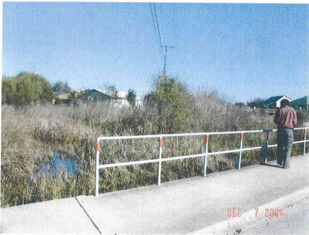
Looking upstream from N. 38 th St
