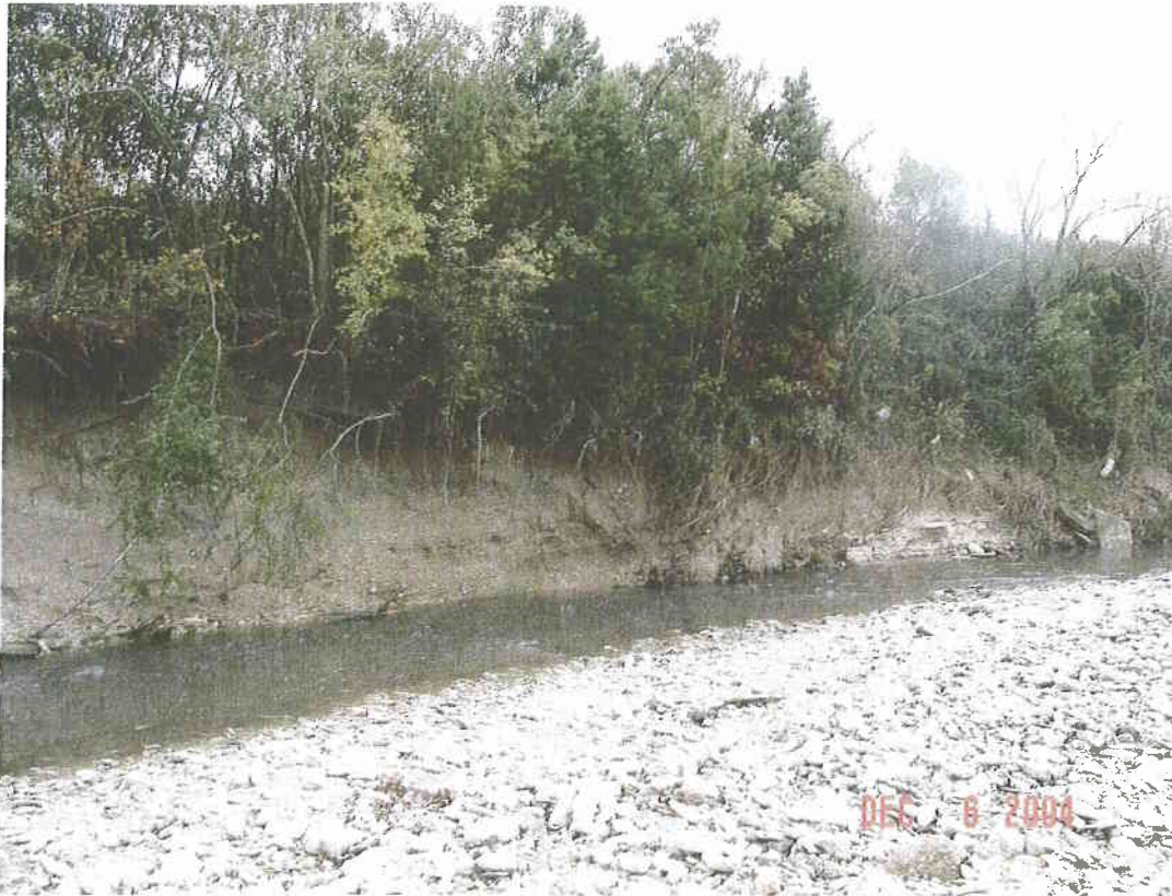
view of eroded bank
