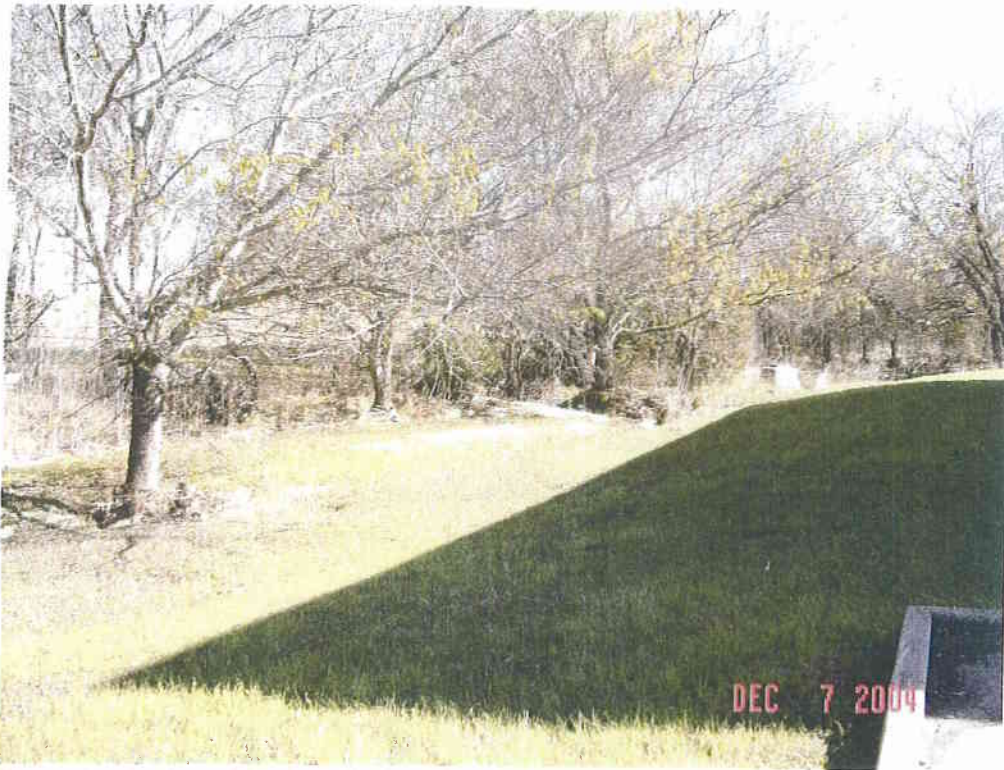
Patriotic Ditch at Charisse St, looking downstream
