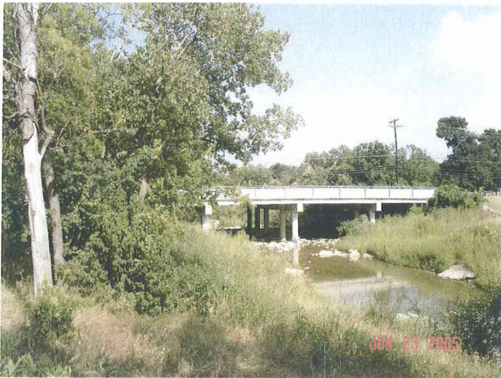
Upstream face of 2 nd Street bridge
