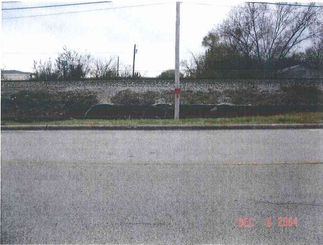
Railroad track culverts
