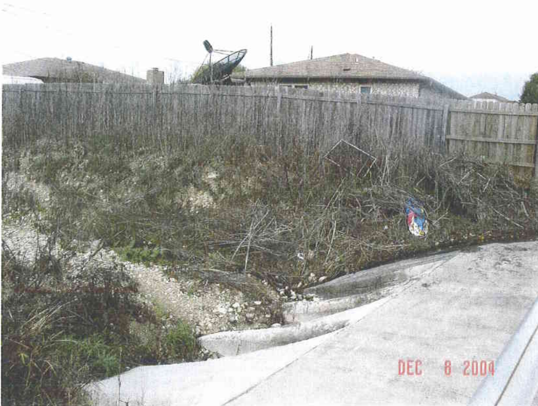
Bending Creek, upstream face of Acorn Creek Trl culvert
