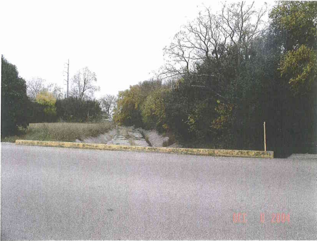
looking upstream from Ave A
