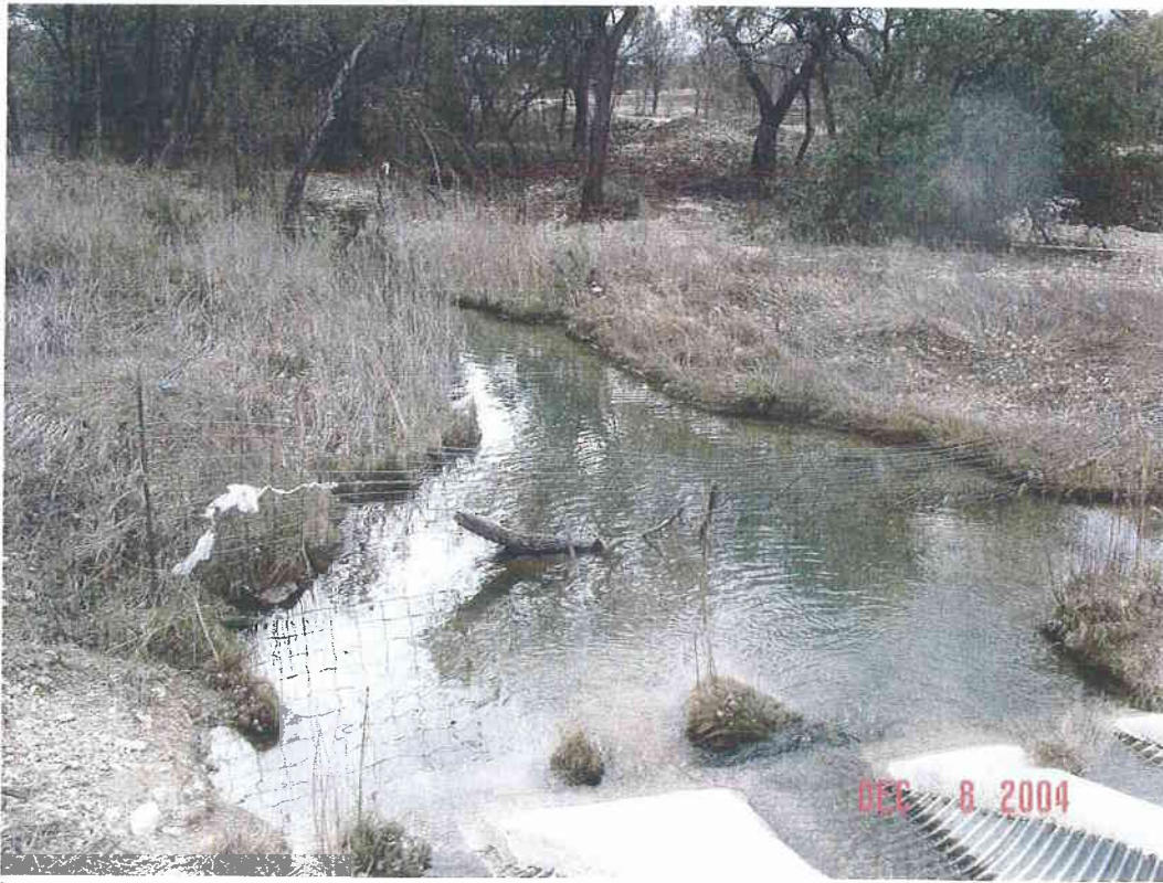
Downstream of culverts.
