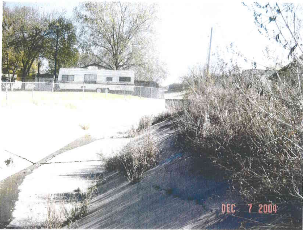
Upstream concrete channel, from Janis St
