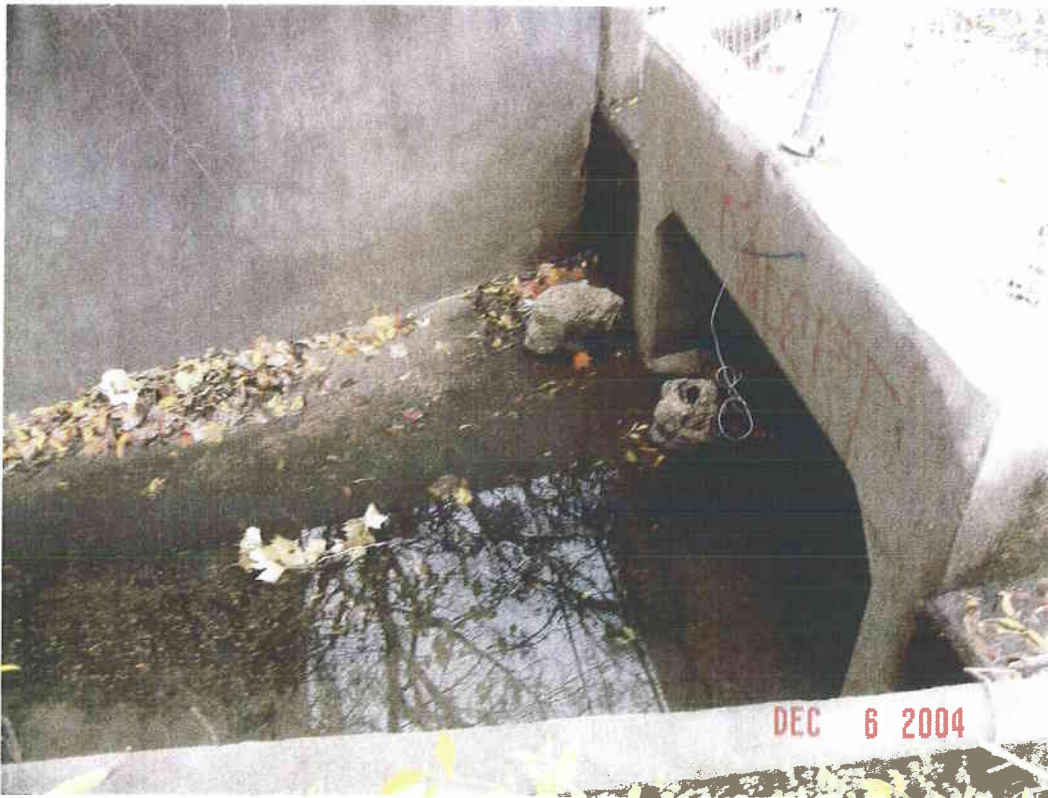
Downstream face of Adams St culvert
