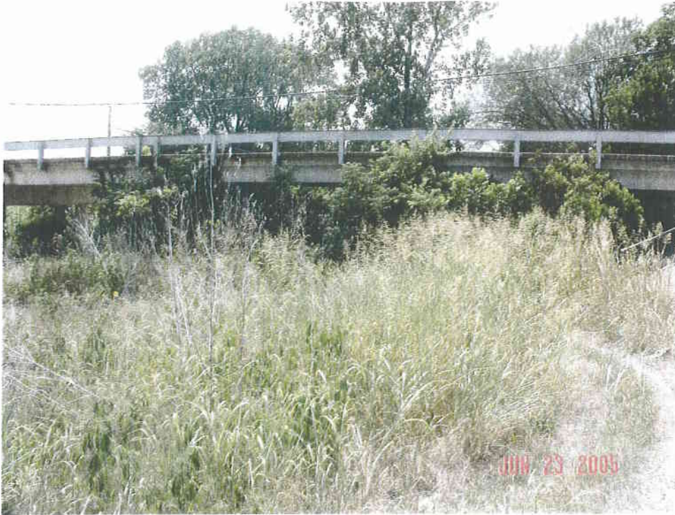
Looking upstream at Dimple St
