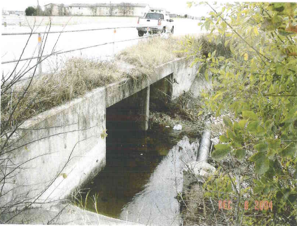
upstream face of Liberty St culverts with sediment and utility crossing
