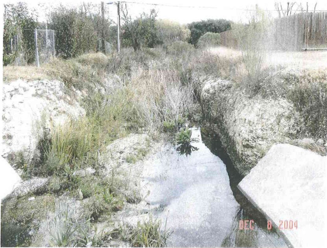
View downstream from Acorn Creek Trl culvert
