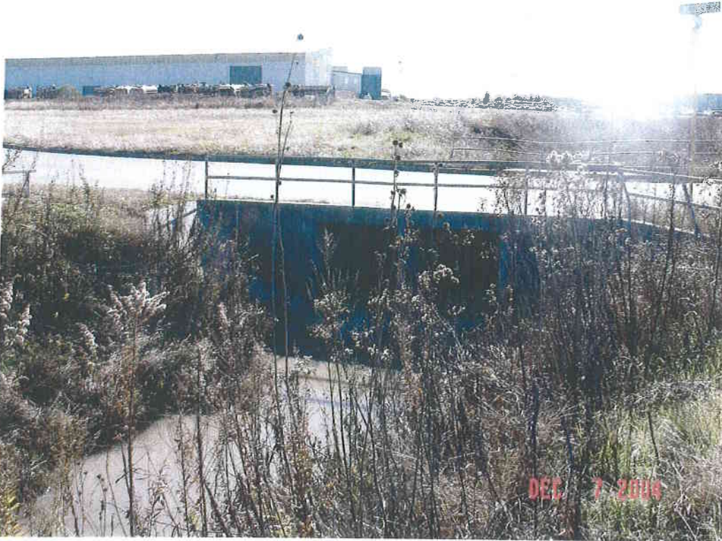
Upstream face of Jacobs Ln culvert
