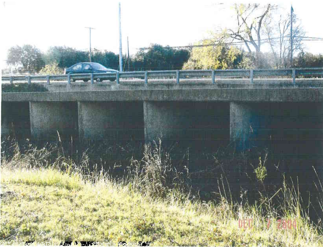
upstream face of Rancier Ave culverts
