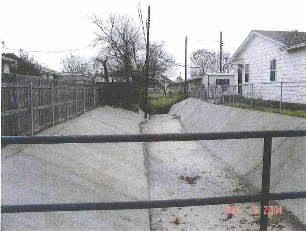
Looking downstream from Bryce Ave. Wolf Ditch flows to 42" CP
