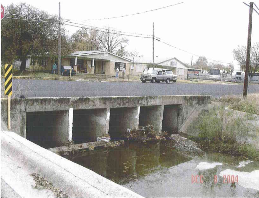
Upstream face of Ave A culvert
