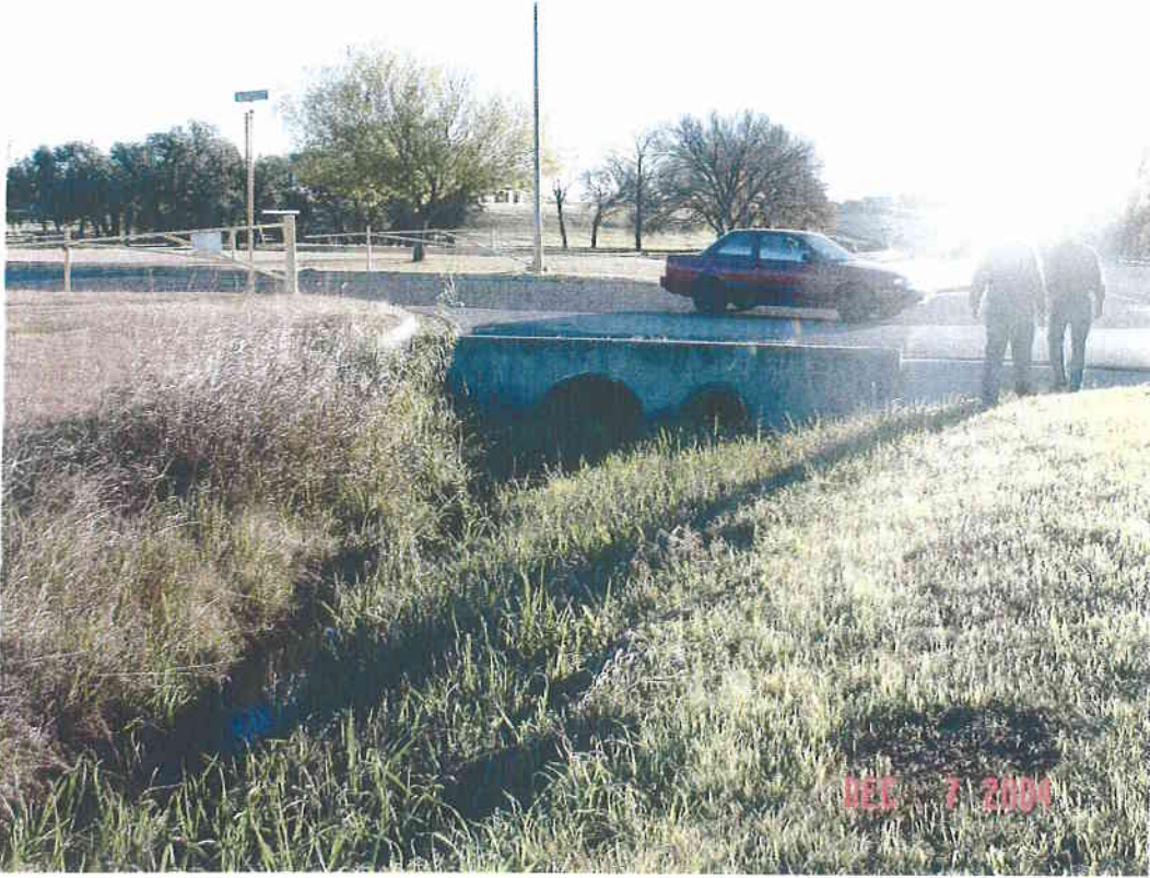
Upstream face of Branch Dr culverts
