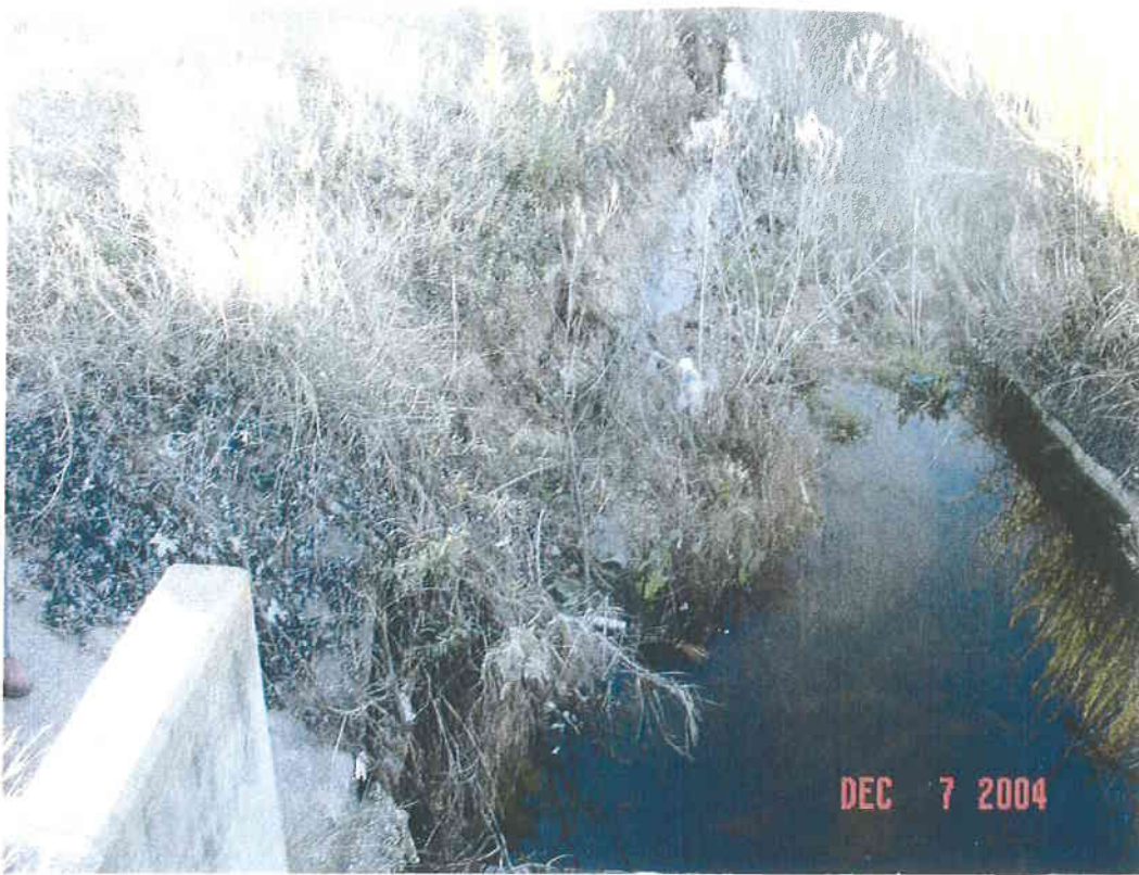
channel, just downstream of Rancier Culvert
