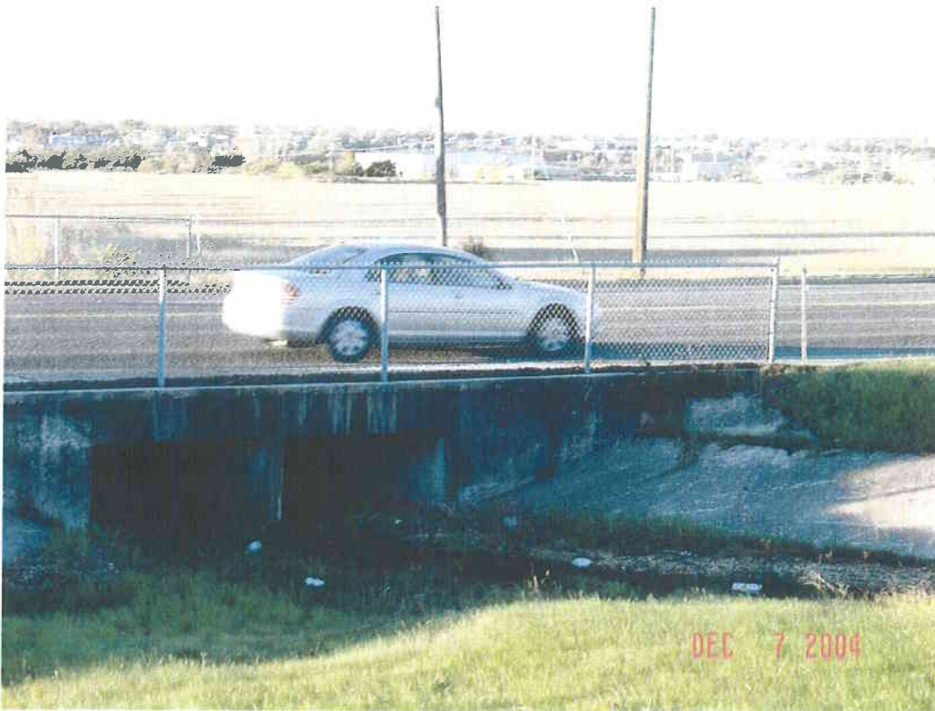
Upstream face of Rancier Ave culvert
