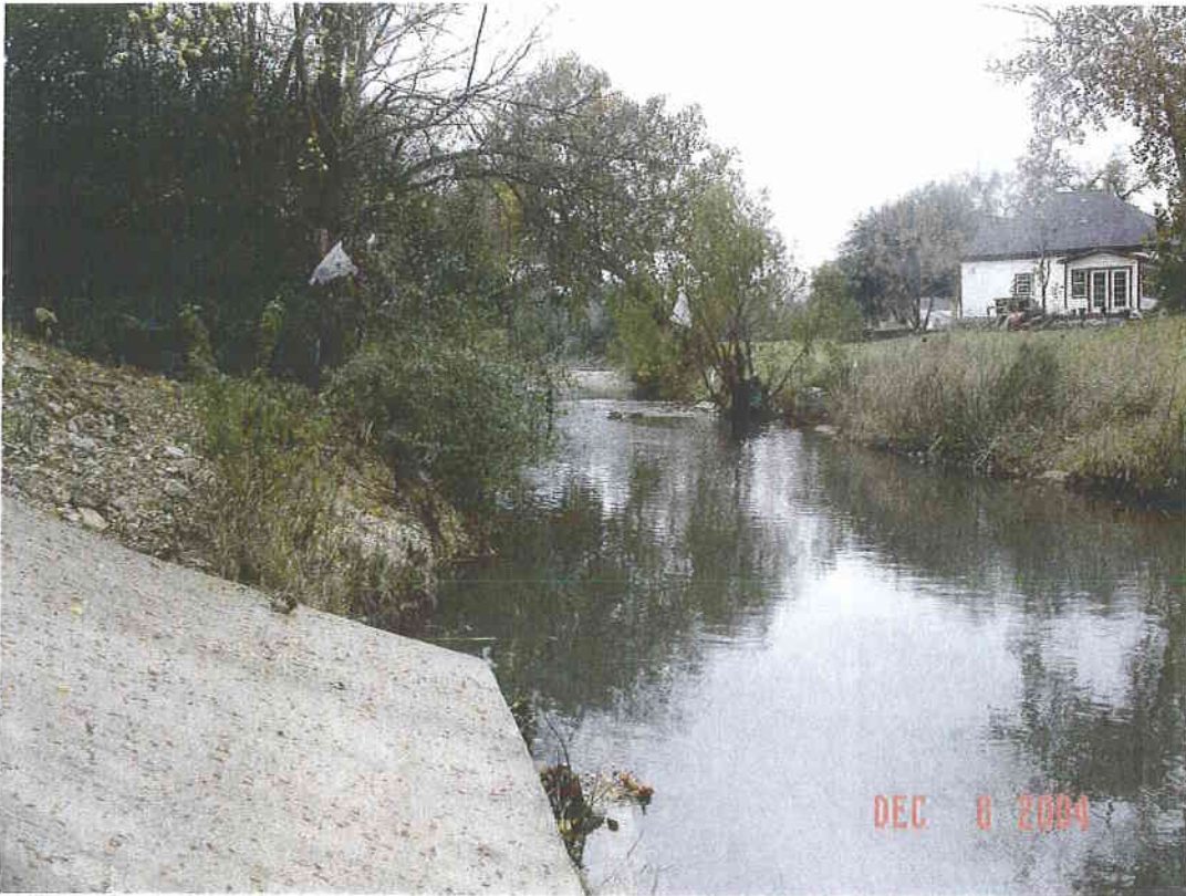
Looking upstream from concrete channel bank armoring, Odom Drive
