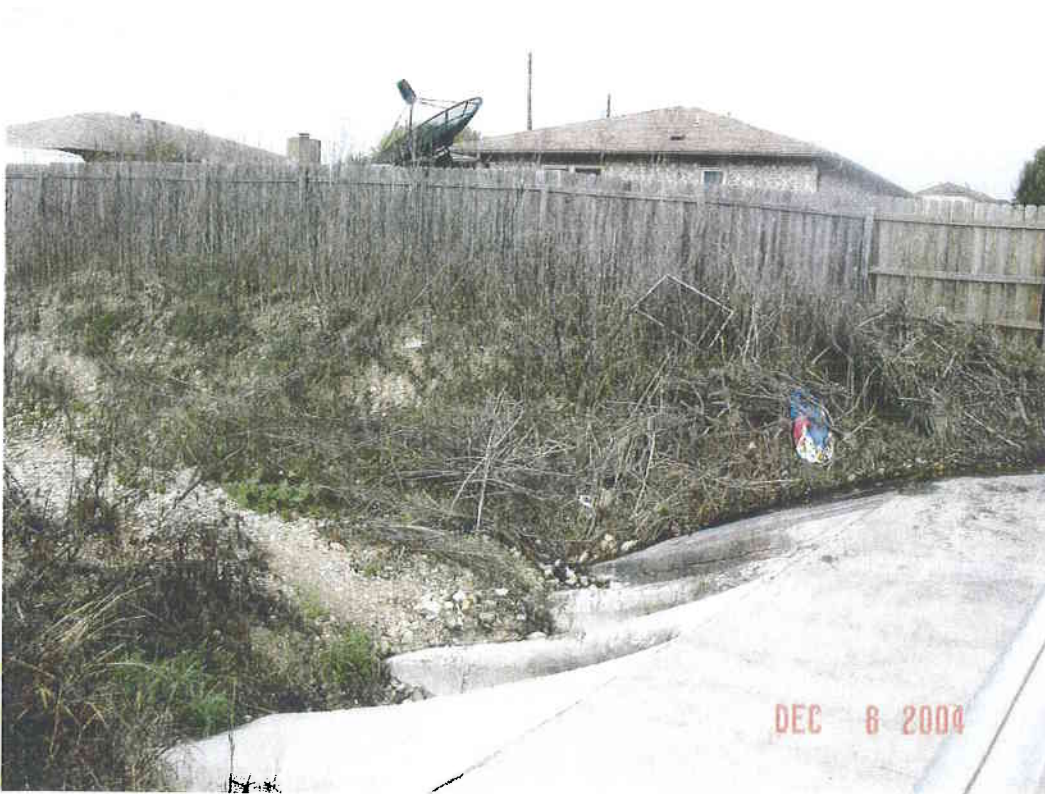
Bending Creek, upstream face of Acorn Creek Trl culvert
