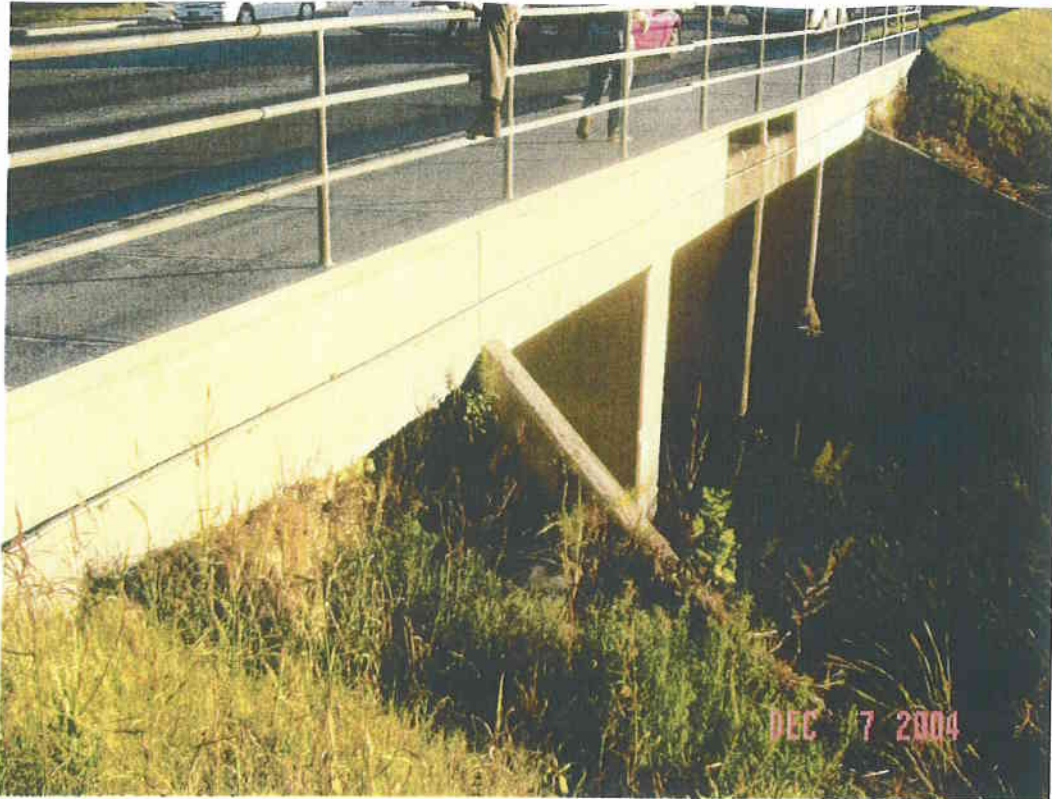
Upstream face of culvert at WS Young
