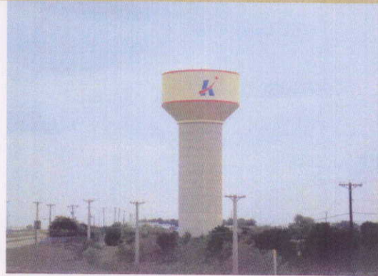
Water tower located at the Airport
