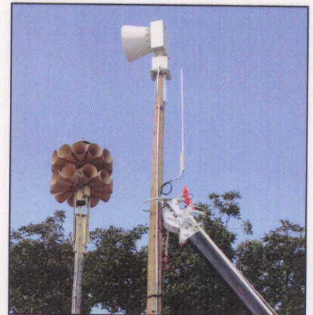
Twenty-one new emergency warning sirens will be installed in Killeen.
