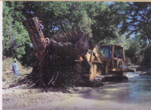
Drainage Utility Crew removing blockage from Nolan Creek
