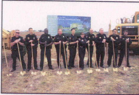
The Killeen Police Department breaks ground on its new headquarters.
