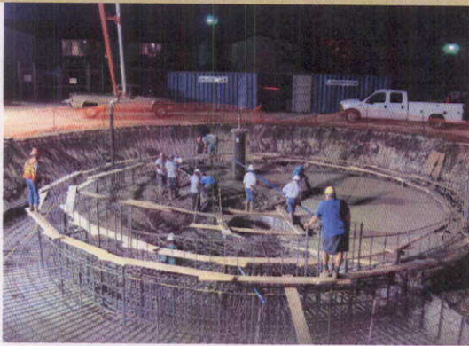
Foundation for new 1.5 million gallon Bundrant Water tower
