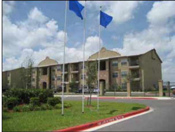
San Pedro at Sharyland Apartments
