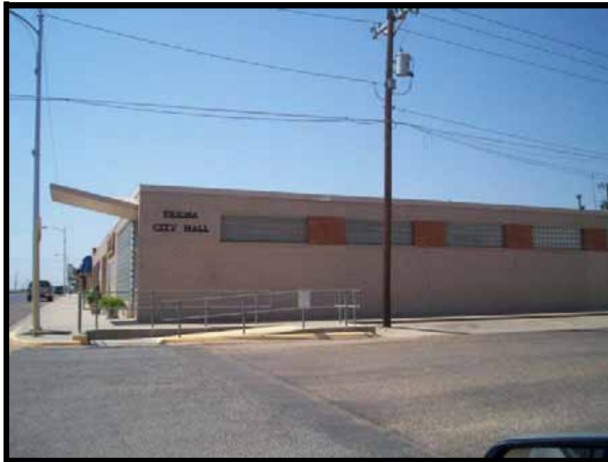
Friona City Hall
