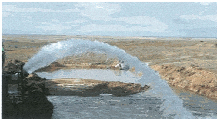
Photo at left shows the step draw test of our first prototype production well. This well is capable of pumping 1000 gpm of high quality water!
