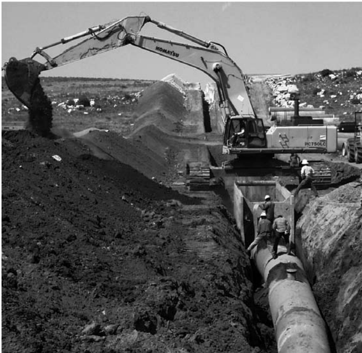
▲ CRMWA installing Ogallala Aquifer well field pipeline in Roberts County.
