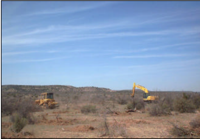
Bulldozers and other heavy machinery are used to effectively clear brush.
