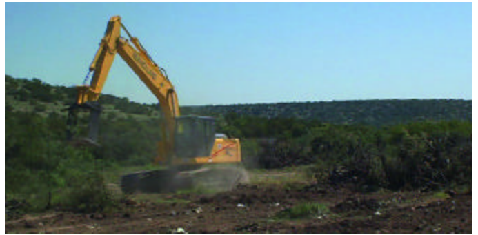
Excavator at work on the Mimms Ranch in Coke County.
