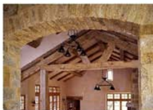
Exposed Roof Structure
