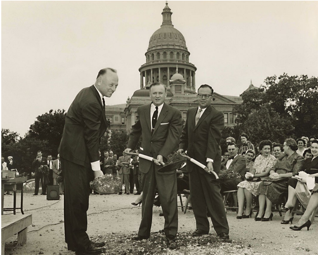
In this photo released by the Texas State Library and Archives Commission, Governor Daniel, center, breaks ground next door to the State Capitol for the new Lorenzo de Zavala State Archives and Library Building in 1959.
