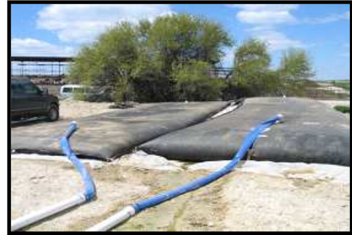
Partially filled Geotubes™
