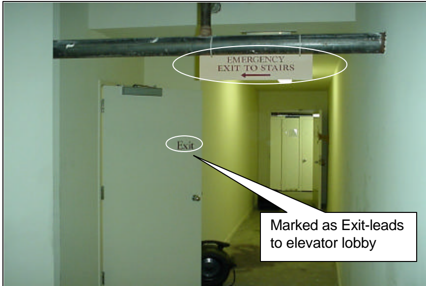
Figure 4-Confusing and inadequate exit signage in Stair C exit pathway
