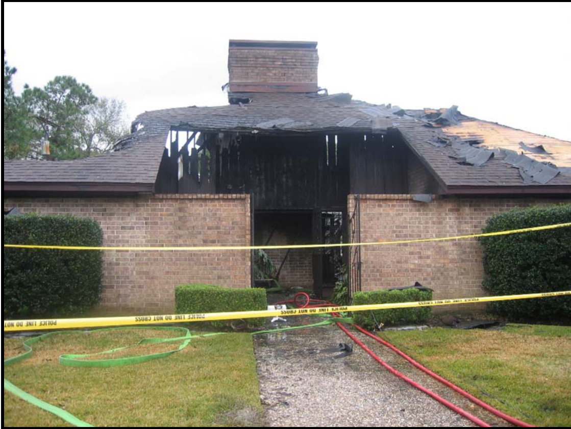
North (main entrance) side of the building
