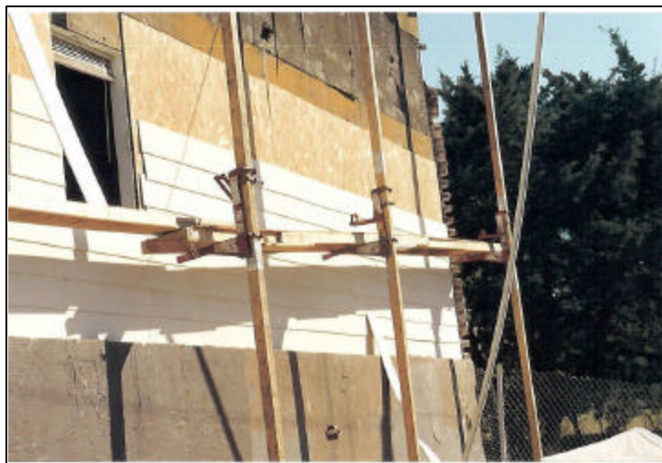
Figure Eight. Southeast end of Section 3 showing brick removal. Photo by BATF.
