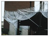
The maximum net opening can't be more than 6 inches on a side, center-to-center. OSHA's design and performance requirements for safety net systems are in CFR 1926.502 (c).
