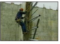
between a positioning device system and a personal fall arrest system is that the positioning device system supports you on an elevated surface and limits a fall to two feet. A personal fall arrest system, on the other hand, doesn't offer support but stops a free fall. Positioning device systems are also called "Class II" work positioning systems. OSHA design and performance requirements for positioning device systems are in CFR 1926.502 (e).
