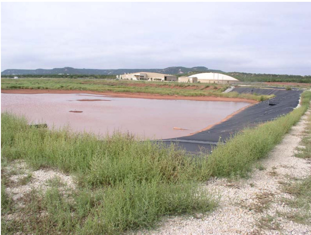
Figure 12-13. City of Abilene west pond showing the liners employed to control wave action
