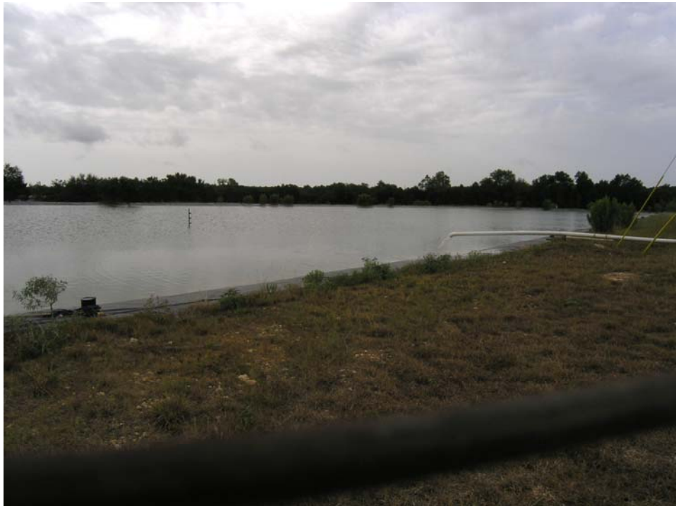
Figure 12-7. View of River Oaks Ranch evaporation pond showing concentrate outfall and water-level gage
