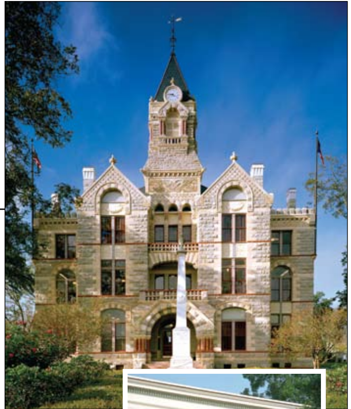
1891 Fayette County Courthouse, rededicated on June 25, 2005
