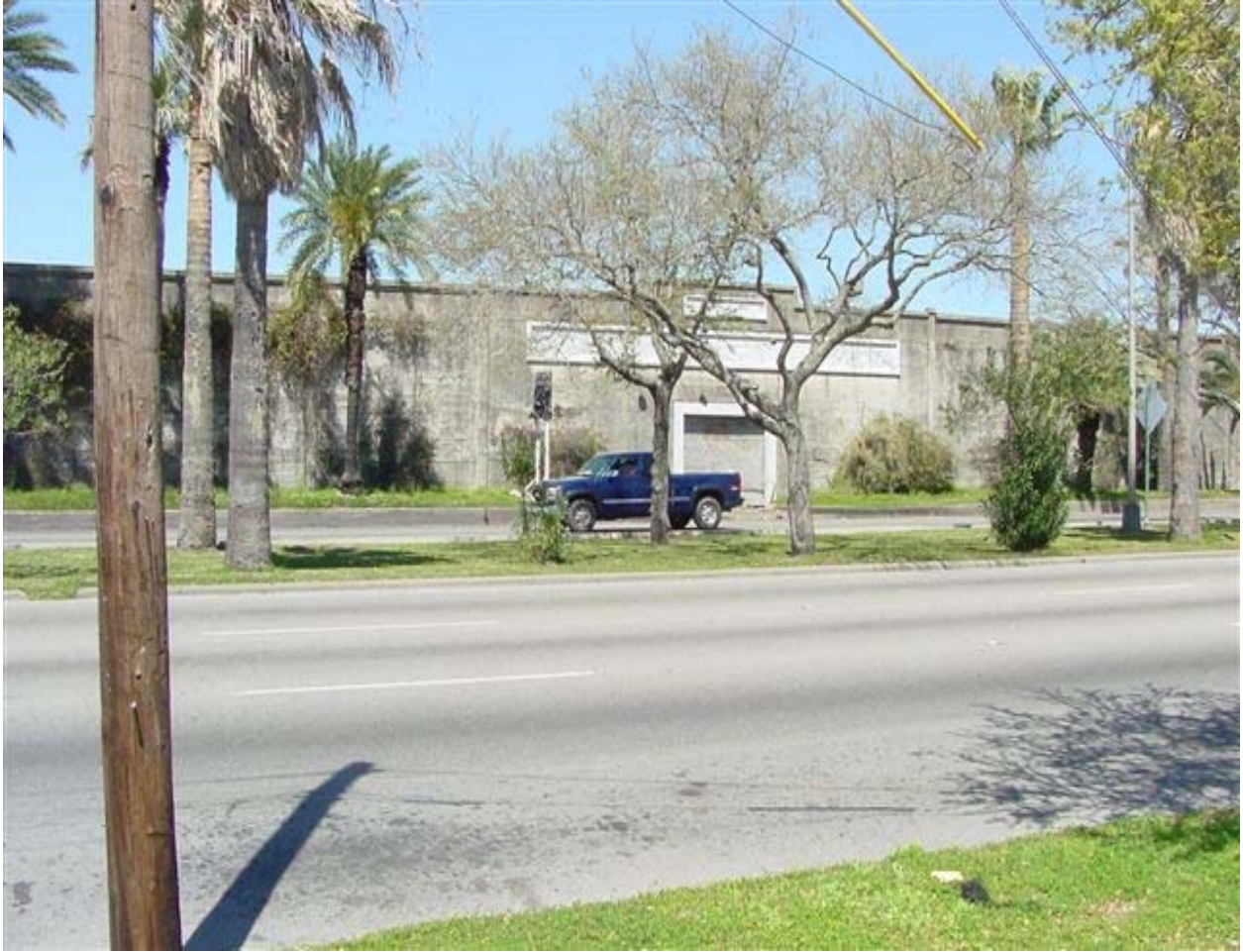
Looking North across the Broadway Esplanade at the Exterior Walls of the Former Moody Cotton Compress, Site of the Future Galveston County Justice Center 2003
