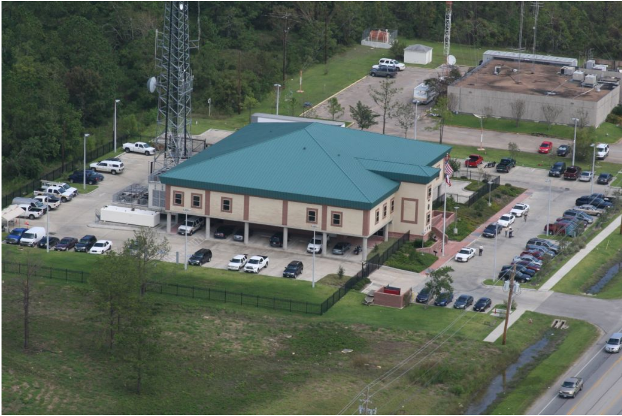
Galveston County's Emergency Management Building in Dickinson, Texas, the command center for county officials when monitoring the approach of a hurricane.
