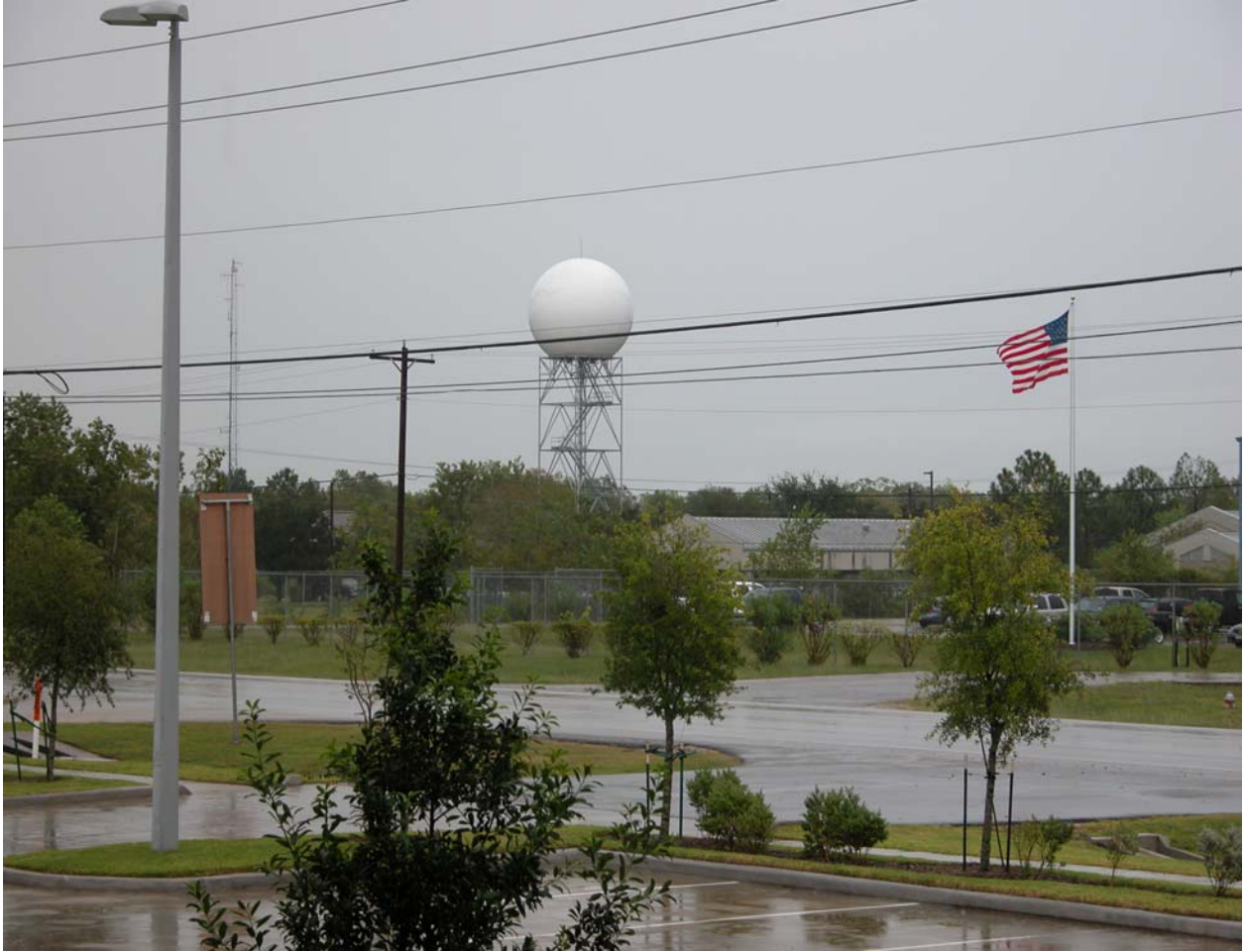
Galveston County Emergency Management Facility National Weather Service Radar Tower and Dome
