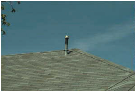
FIGURE 18: PLUMBING VENT
