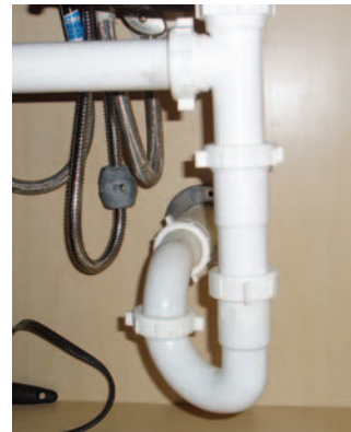
FIGURE 19: PLUMBING TRAP
