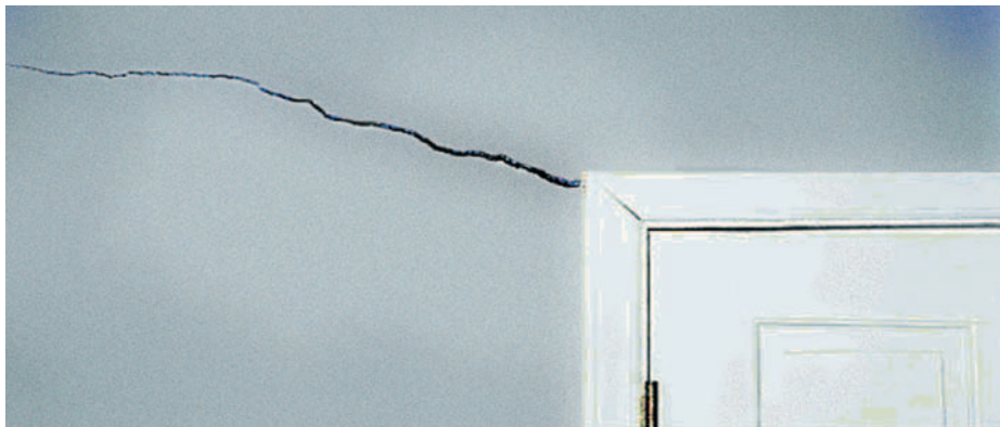
FIGURE 6: DRYWALL CRACK
