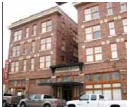
Historic Rogers Hotel to become a premier boutique/event hotel.
