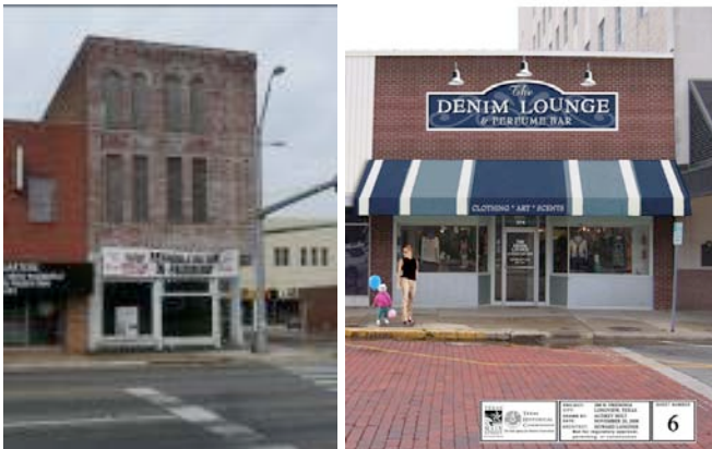
Rehab in progress banner on the Gregg-Link building in Palestine (l) and TMSP design rendering done for Longview (r)
