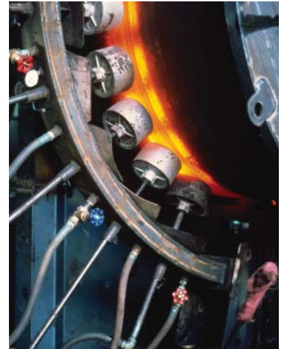
Boilers are inspected periodically by TDLR Commissioned inspectors
