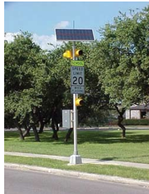
EXHIBIT 3-21 School Zone Warning Light. An Example of a Stand-Alone Solar Application
