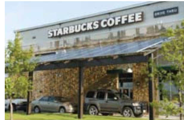
EXHIBIT 3-20 Commercial-scale PV Systems
