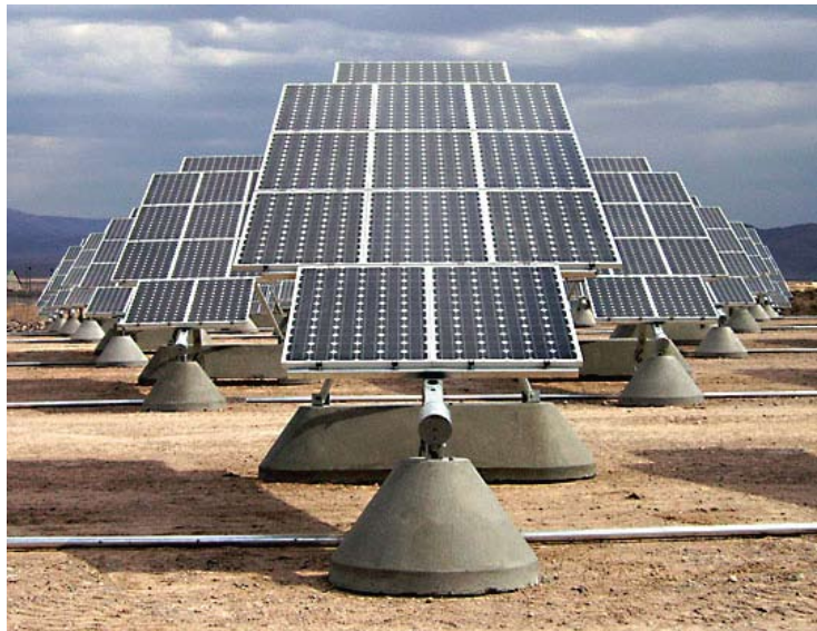
EXHIBIT 3-17 15 MW Tracking PV Array at Nellis Air Force Base, Nevada
