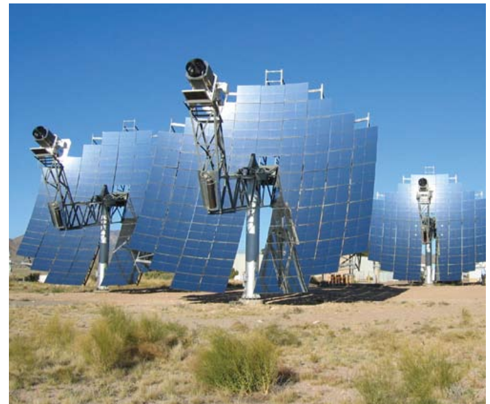
EXHIBIT 3-15 Dish concentrator (dish Stirling design)
