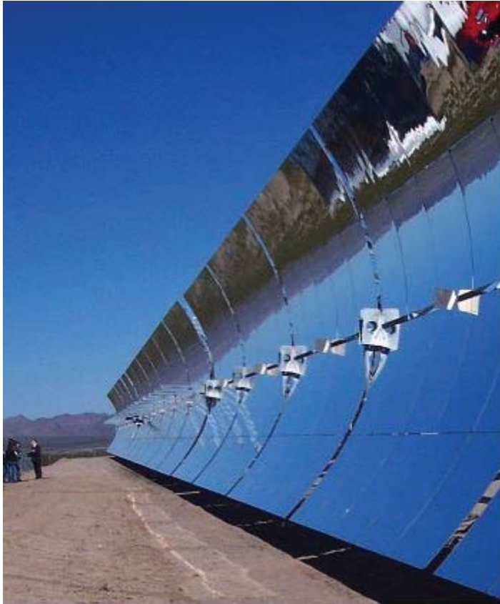
EXHIBIT 3-13 Nevada Solar One (parabolic trough linear concentrator design)
