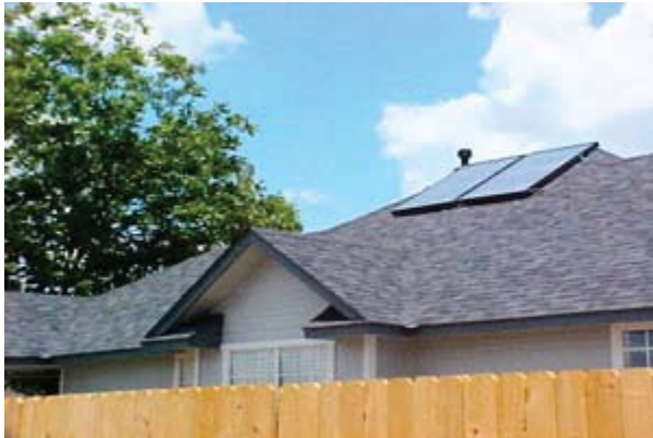
EXHIBIT 3-18 Domestic Solar Thermal Water Heater
