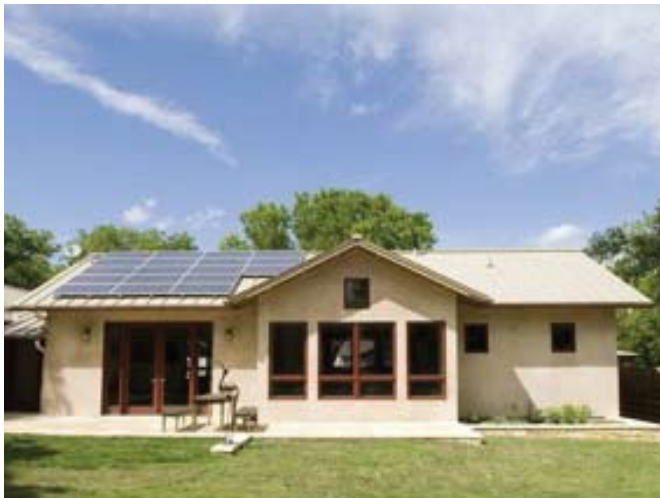
Exhibit 3-19. Residential-scale PV System
