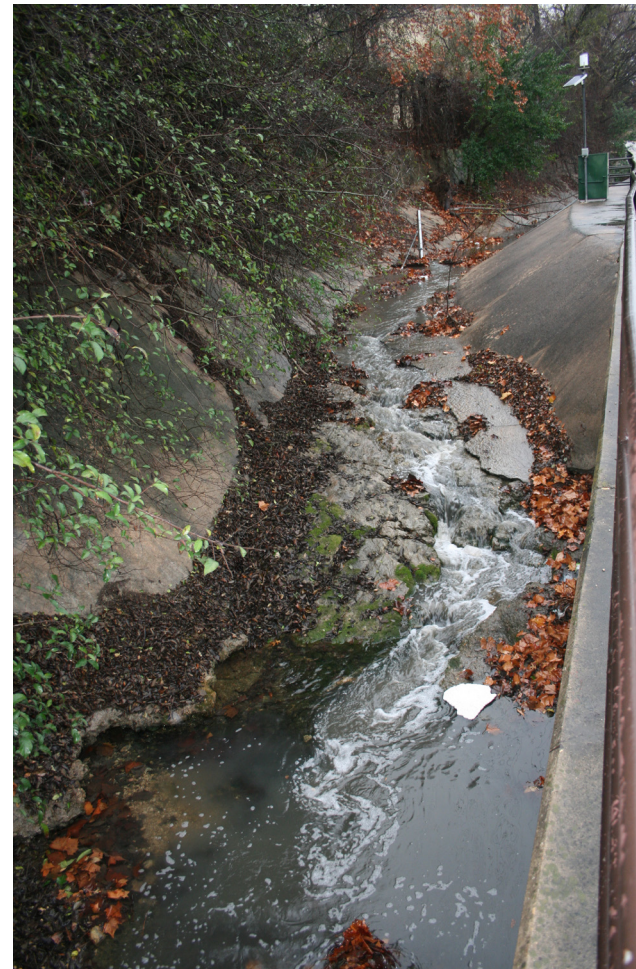
J. Buratti, An Open Storm Water Drainage in Central Texas
