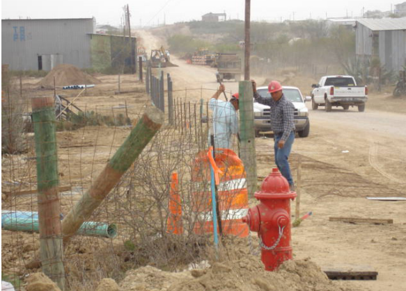
O. Muñoz, Pre-plumbing Preparation in a Colonia
