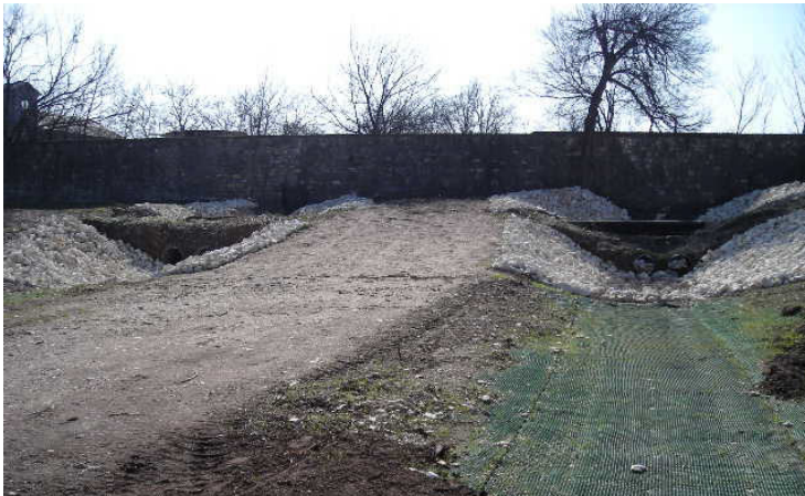
Infiltration trenches for Brady Creek during construction
