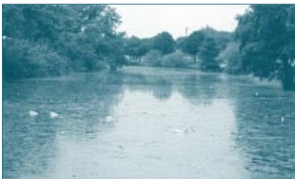
The amount of debris reaching the river has been substantially and visibly reduced since completion of the Civic League Park structure.
